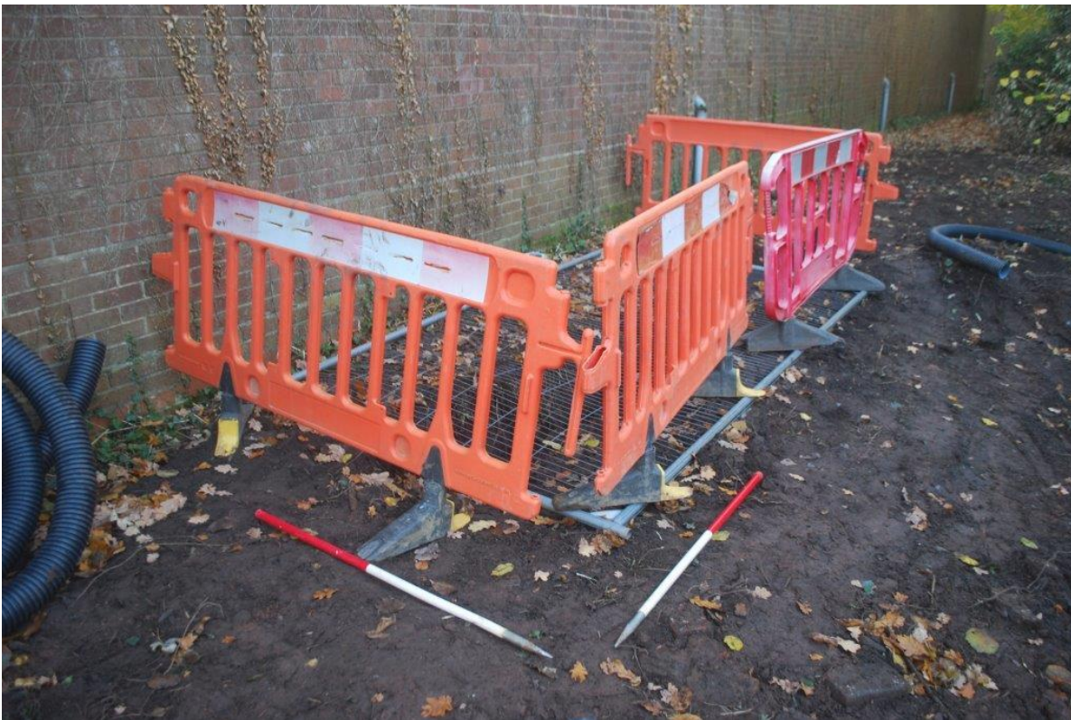
Plate 4 Proposed gas tank location fenced off around trench 4. 2 x 1m scales.
