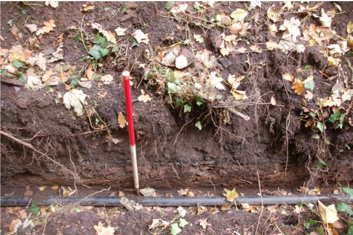
Plate 2 Sample section of trench 4, showing topsoil, clinker demolition deposit and disturbed natural at base.
