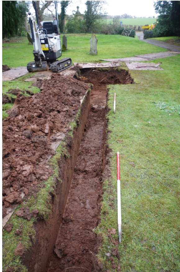
Plate 5: Looking north-east across the excavation of Trench 2, scales 1m.
