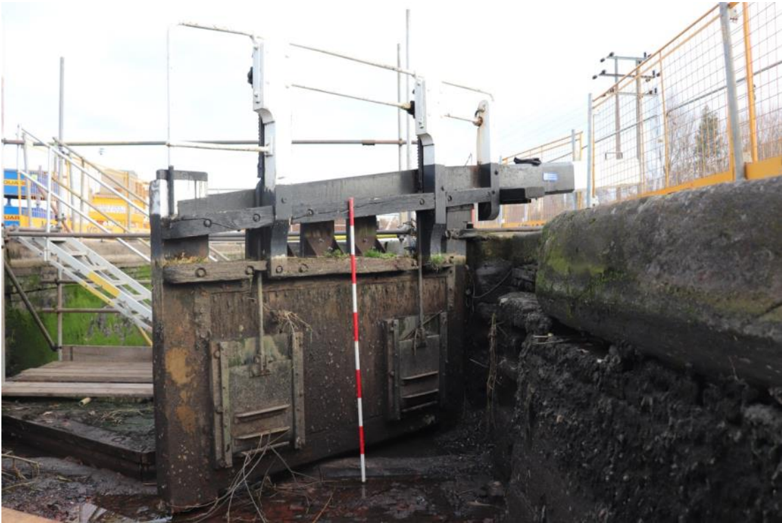
Plate 12 Head gate with double paddles, looking north-east, 2m scale
