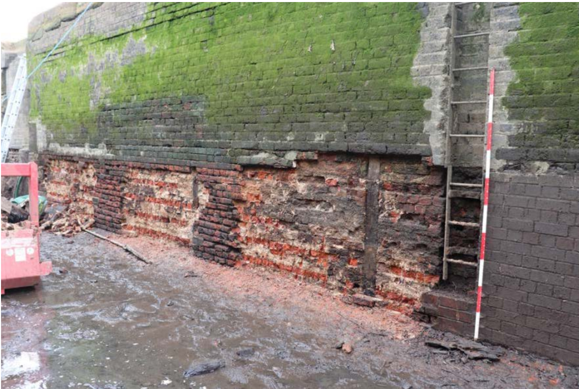
Plate 6 Vertical timbers within the walls, looking east, 2m scale
