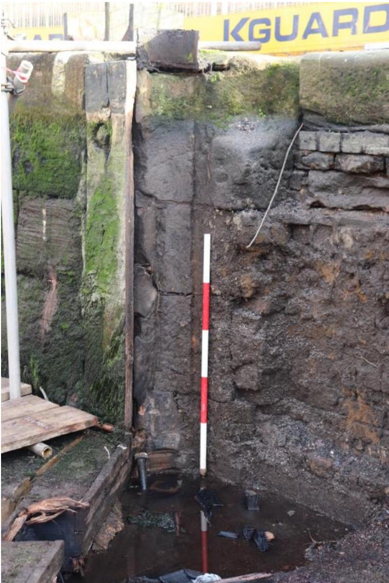
Plate 8 Stonework at the pivot of the head gates, looking north-east, 2m scale
