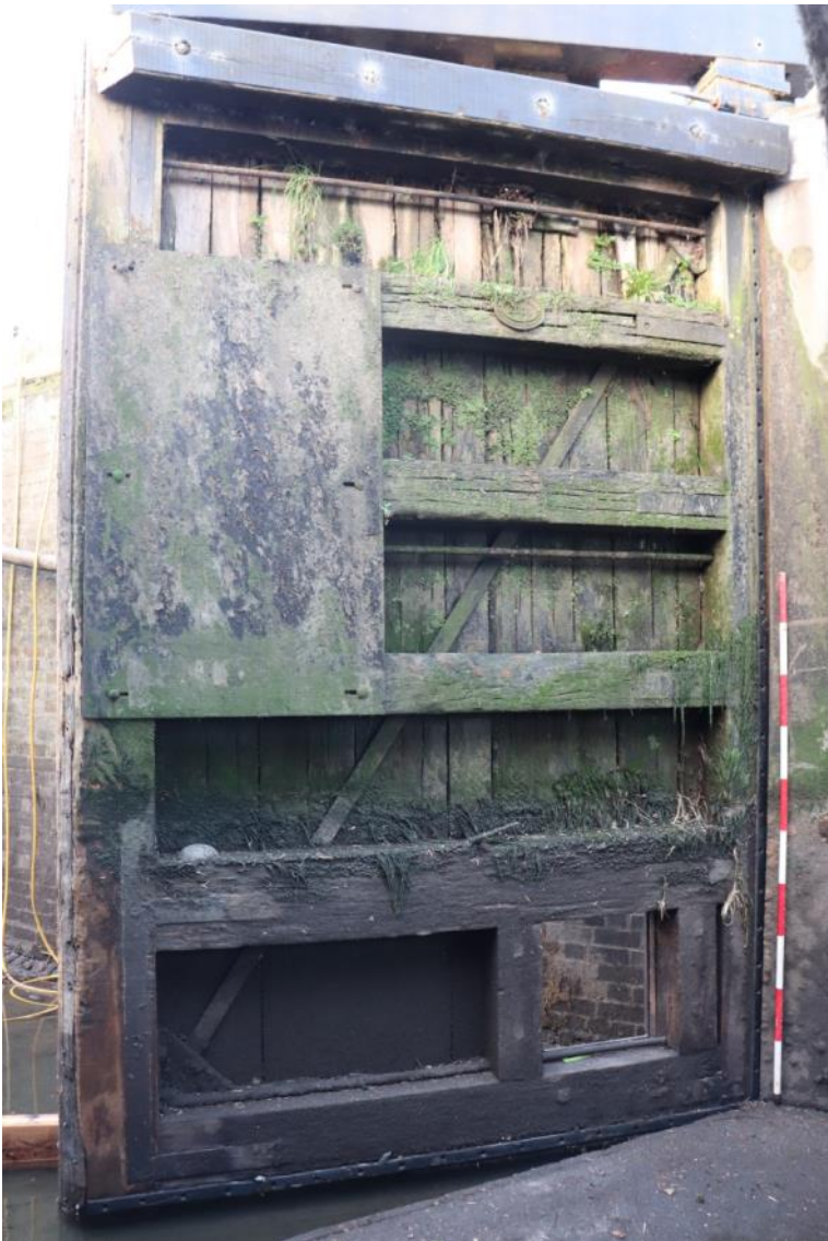
Plate 10 Tail gate with single paddle, looking south-west, 2m scale
