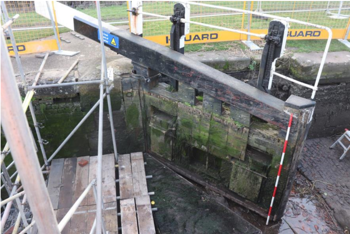
Plate 11 Head gate with double paddles, looking south-east, 2m scale
