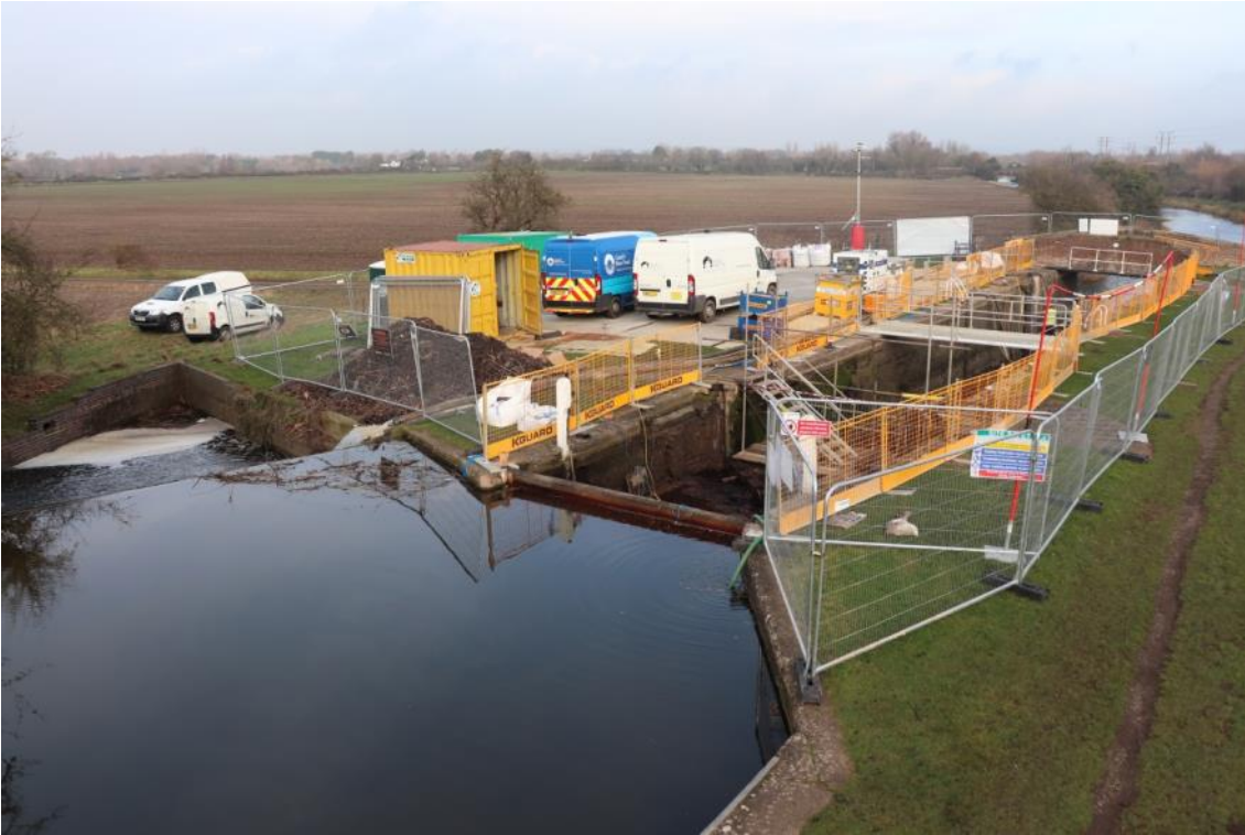
Plate 1 The lock, looking north
