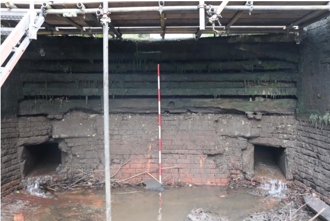
Plate 5 The timber cill with ground paddle culverts visible below, looking south-west, 2m scale
