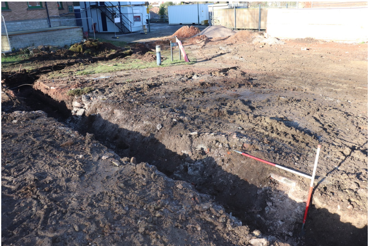
Plate 4: Trench 1, limestone footings from Lawnstone house; view north-west 2x 1m scales
