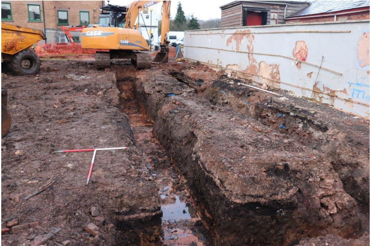
Plate 9: Trench 3, north block footings in progress; view west; 2x 1m scales
