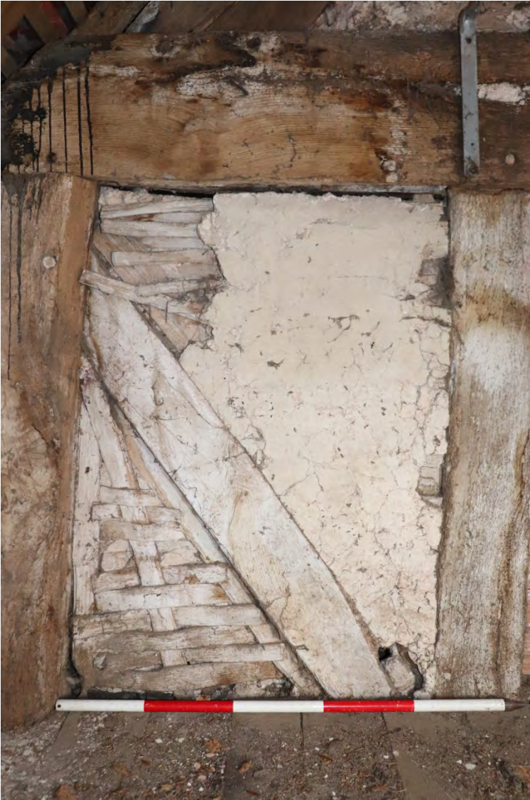
Plate 12 Phase1 wattle panel with later lime plaster, looking east, scale 1m
