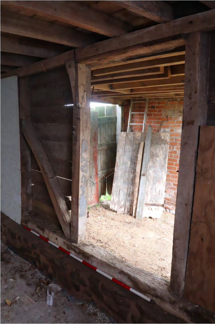
Plate 24 Phase 3 sill, wall framing and brace, looking north-east, scale 2m
