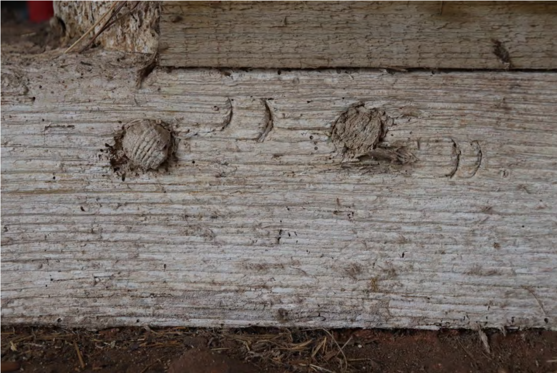
Plate 26 Phase 3 Carpenters marks, looking west
