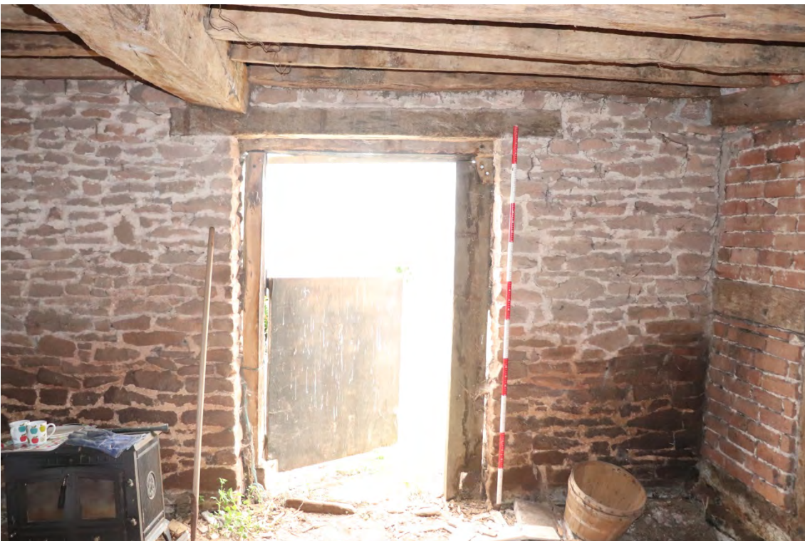
Plate 16 Phase 2 element, looking south, scale 2m
