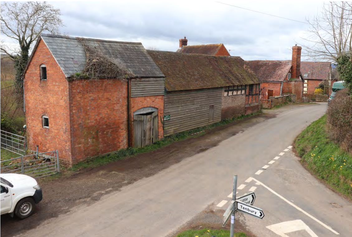
Plate 1 The building, looking south-west
