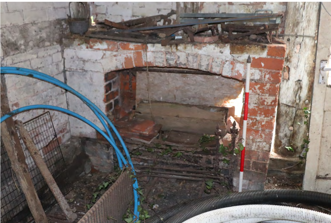
Plate 29 Phase 4 added fireplace, looking south, scale 1m
