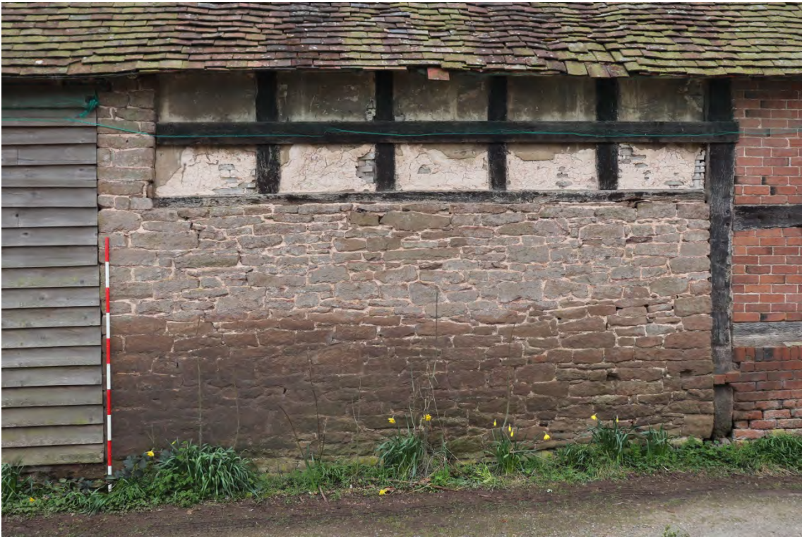
Plate 13 Phase 2 element, looking south, scale 2m
