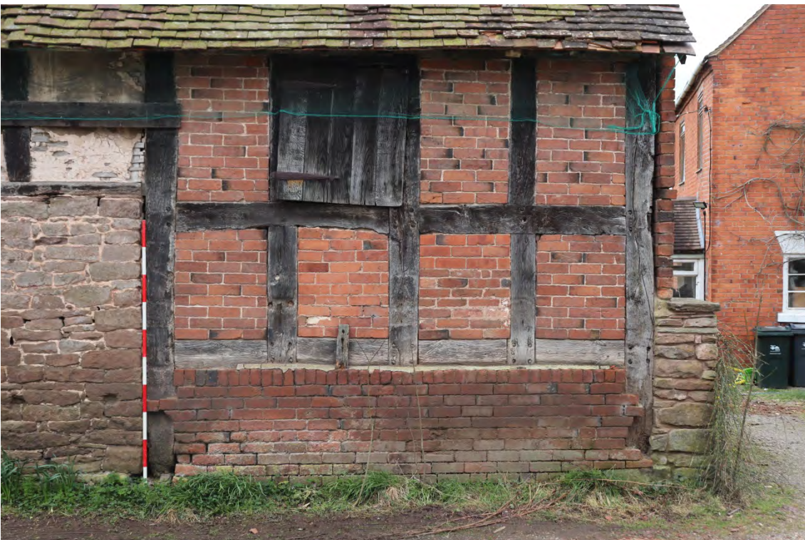
Plate 6 Phase 1 element, looking south, scale 2m
