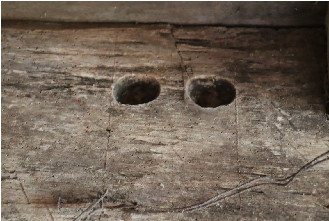
Plate 17 Phase 2 element started mortices, looking west
