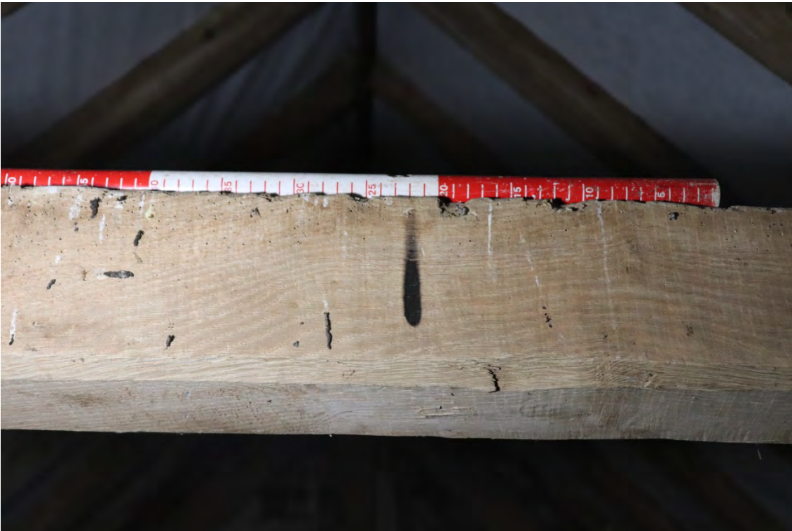
Plate 28 Phase 3 tie collar and candle burn mark, looking east, scale in centimeters in 20cm sections above
