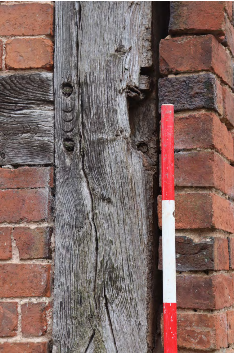
Plate 10 Phase1 empty mortice, looking south,20 cm of 2m scale visible
