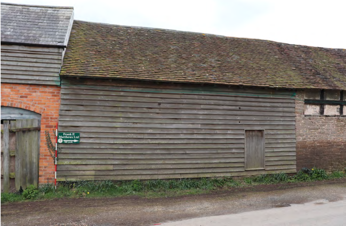
Plate 18 Phase 3 element, looking south, scale 2m
