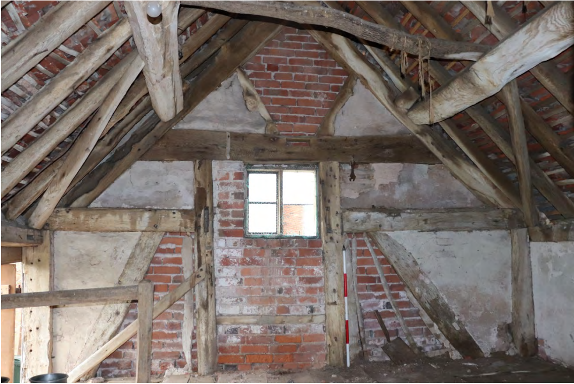
Plate 9 Phase1 former central, now gable truss, looking west, scale 1m
