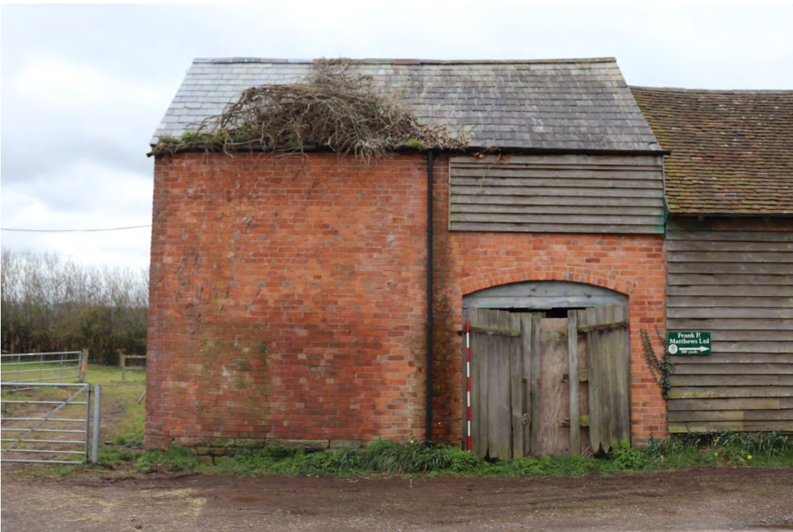
Plate 31 Phase 4 element, looking south, scale 2m
