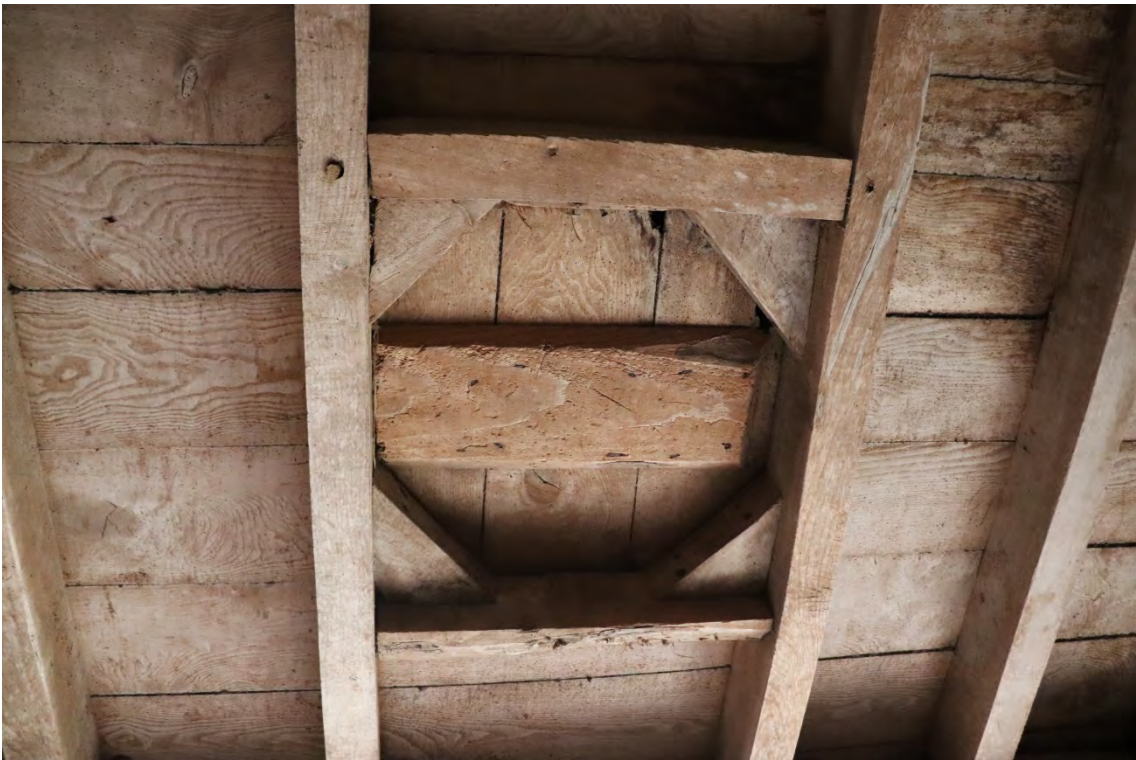
Plate 41 Phase 4 additional hatch, looking south
