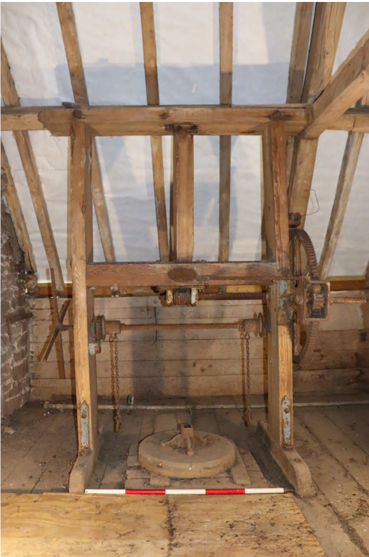
Plate 38 Phase 4 hop press, looking north, scale 1m
