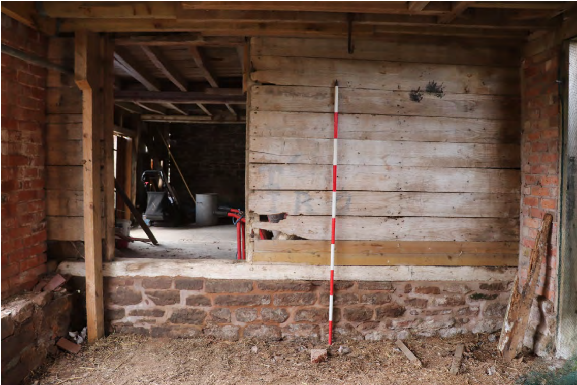
Plate 20 Phase 3 gable weather boarding, looking west, scale 2m
