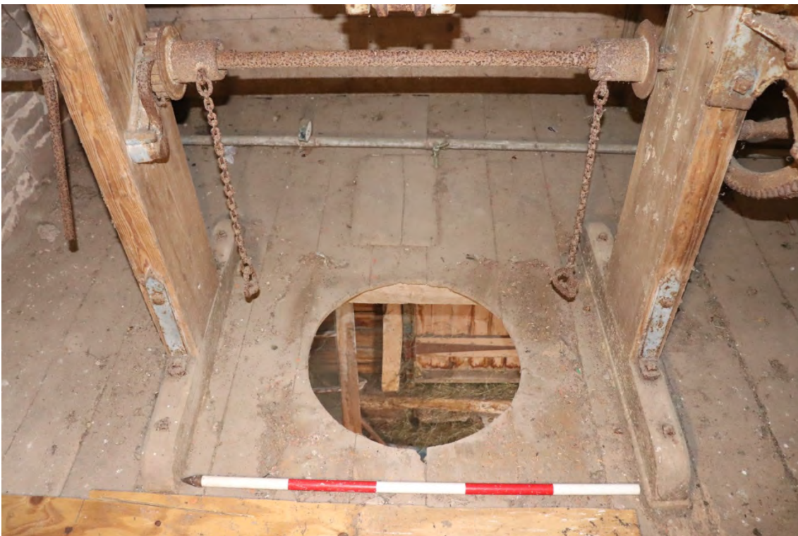
Plate 40 Phase 4 hop press, looking north, scale 1m
