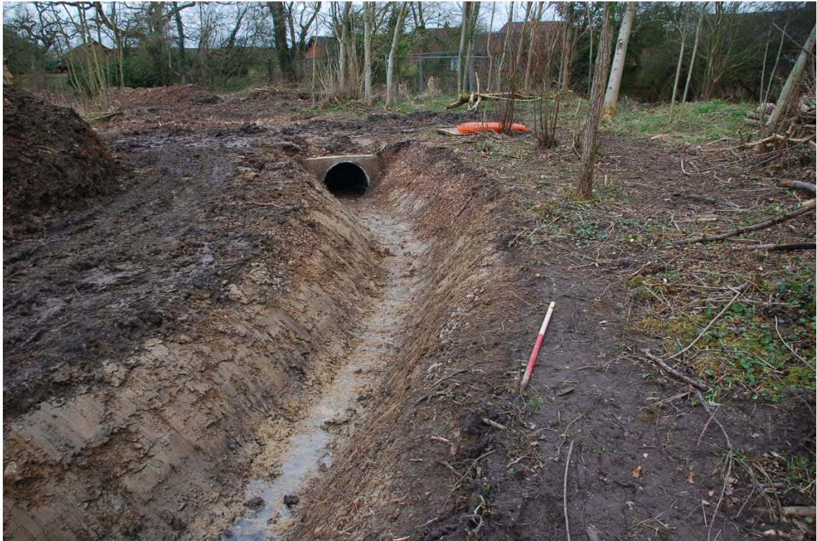
Plate 3: An example of the previously excavated stream diversion in the south of the site. The control structure can be seen towards the rear, 1m scale.
