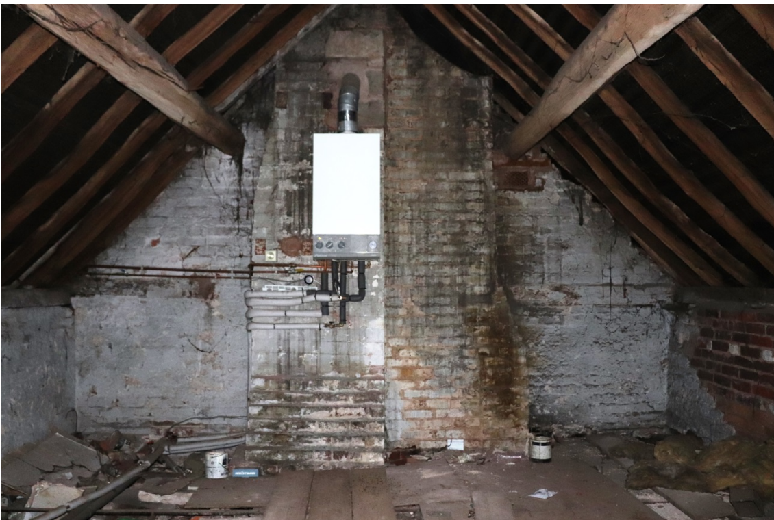
Plate 11 The building first floor, room over the cafe, looking east
