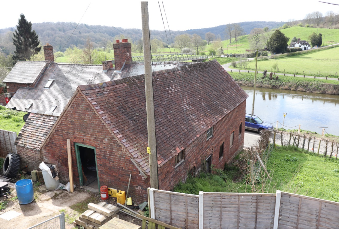
Plate 3 The building, looking south
