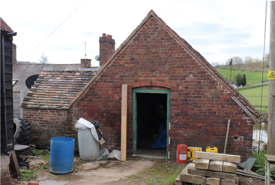
Plate 10 The building first floor entrance, looking south, scale 1m
