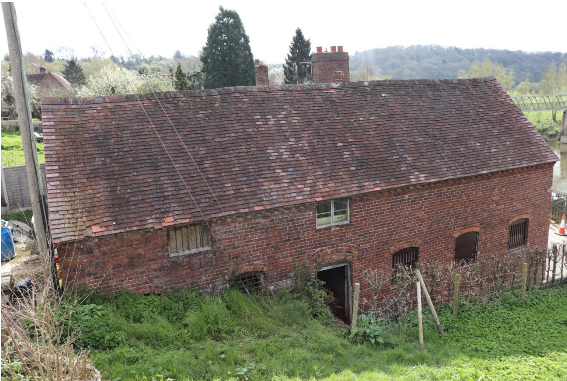
Plate 8 The building, looking south-east, scale 1m
