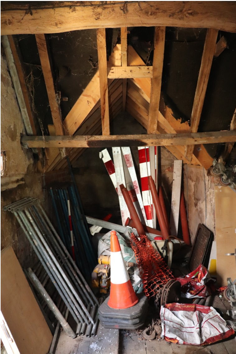
Plate 13 The building first floor, looking east, scale 1m
