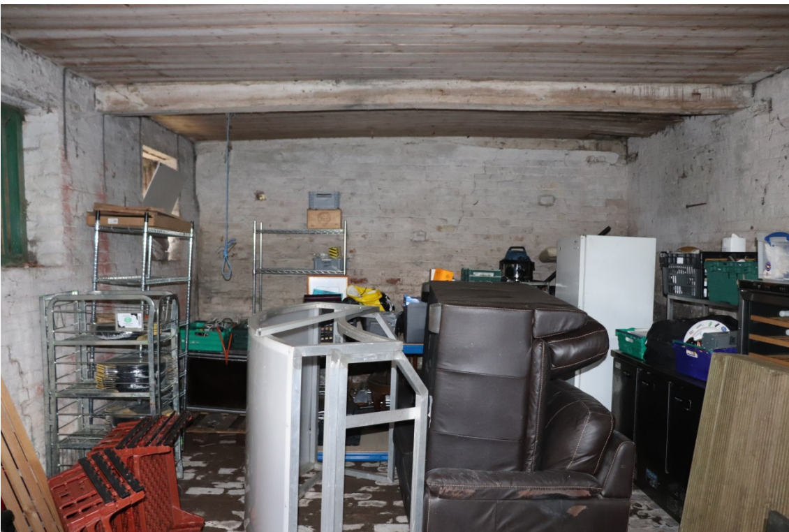
Plate 4 The building ground floor, looking north
