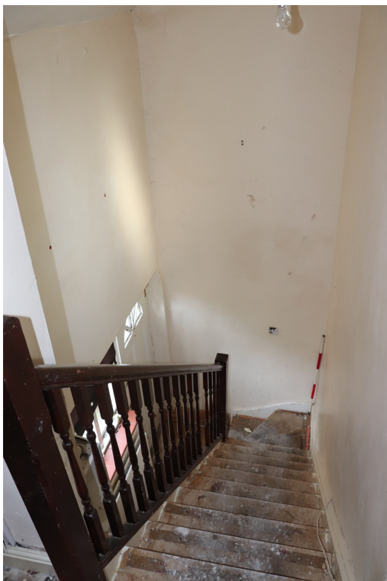
Plate 31 The house second floor, added stairwell, looking east, scale 1m
