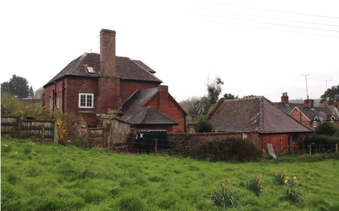
Plate 3 The house and garage, looking south east
