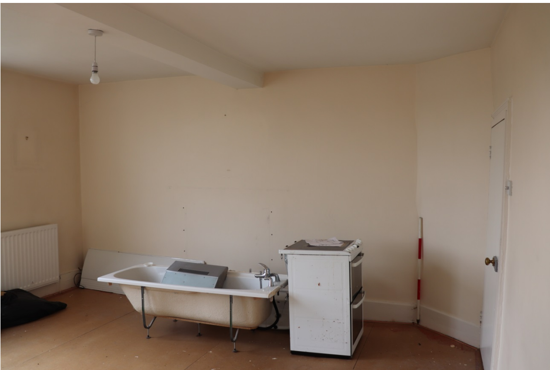
Plate 24 The house first floor, south-west room, looking west, scale 1m
