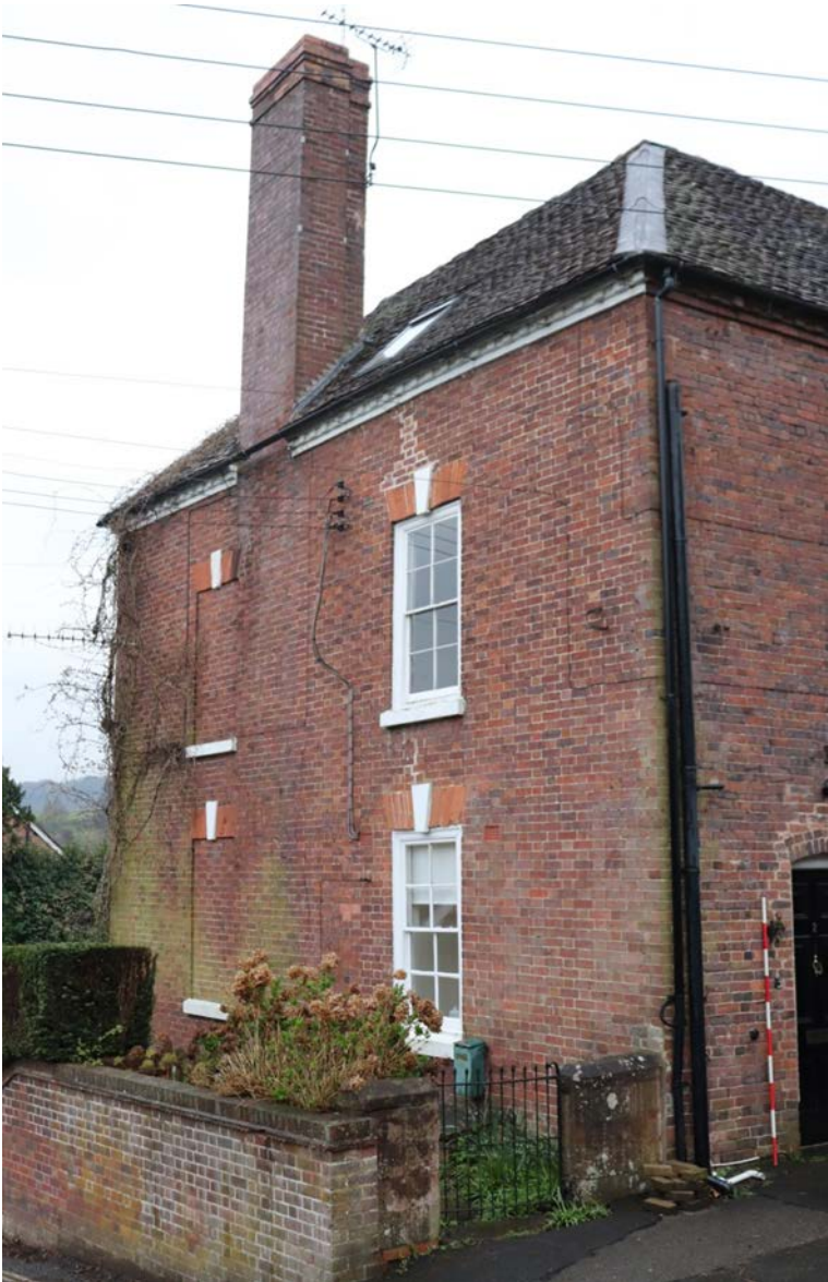
Plate 6 The house, looking south-west, scale 2m
