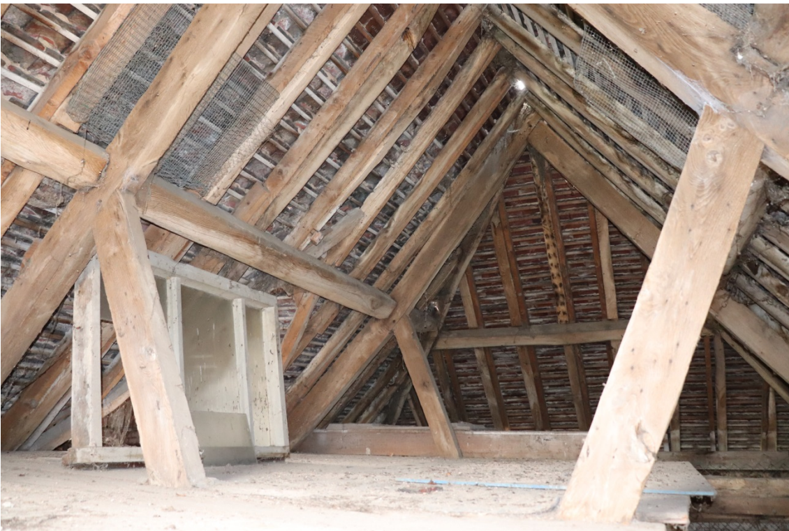
Plate 37 The garage, looking west
