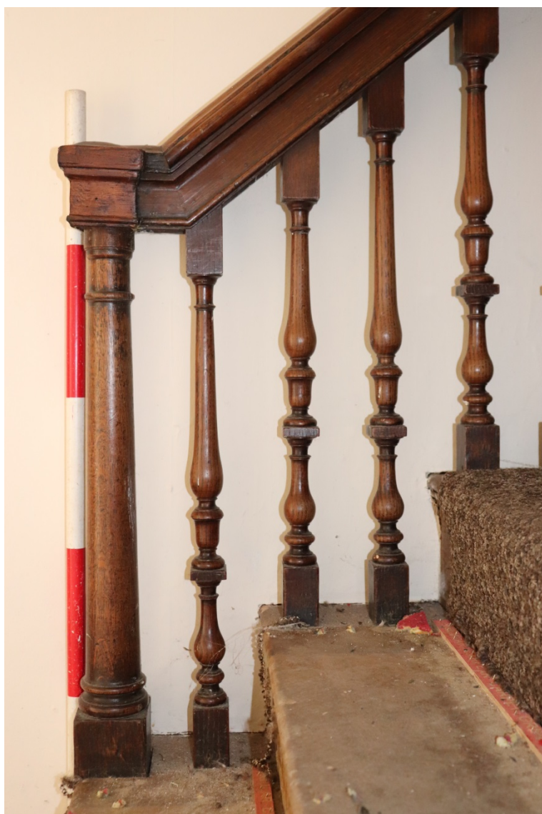
Plate 15 The house ground floor north-east room and staircase, looking south, scale 1m
