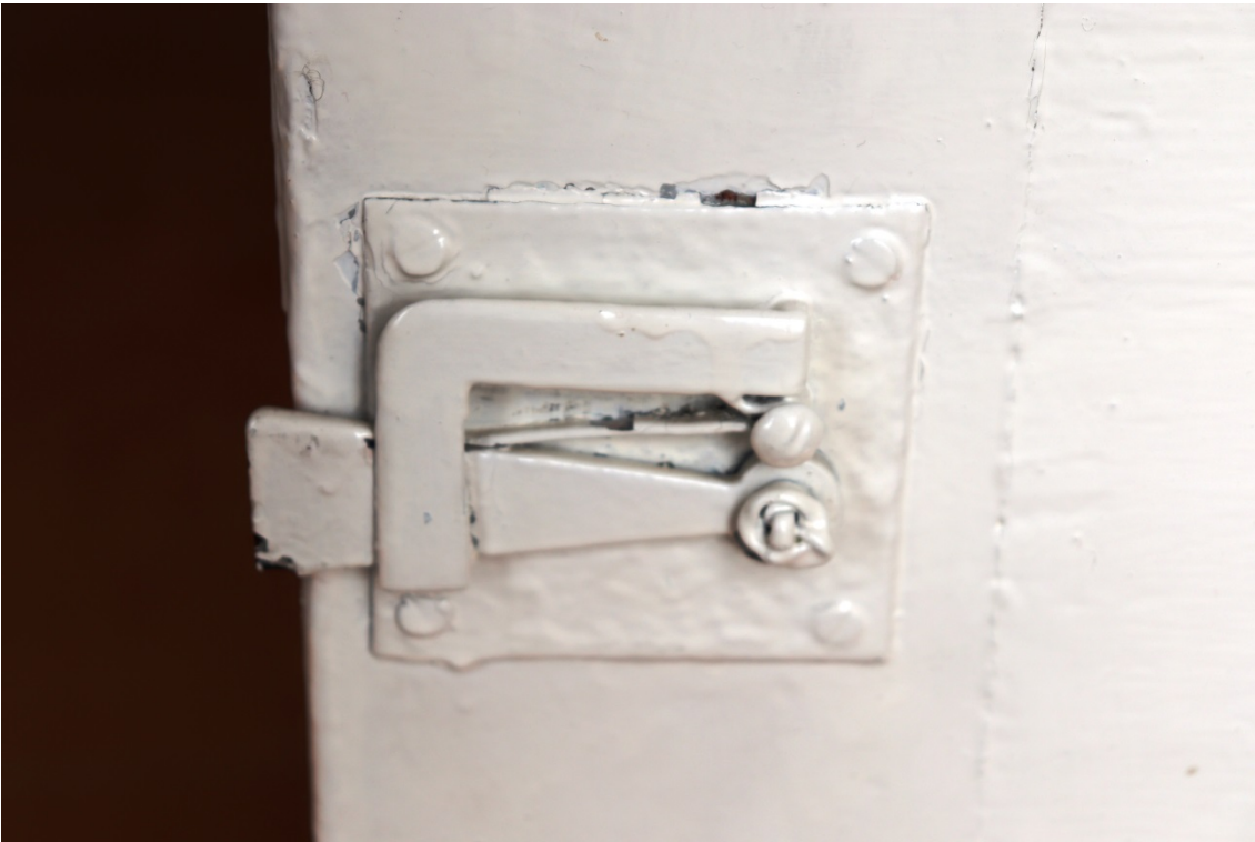
Plate 23 The house first floor with original thin 2 panel door and rear latch, south-east room
