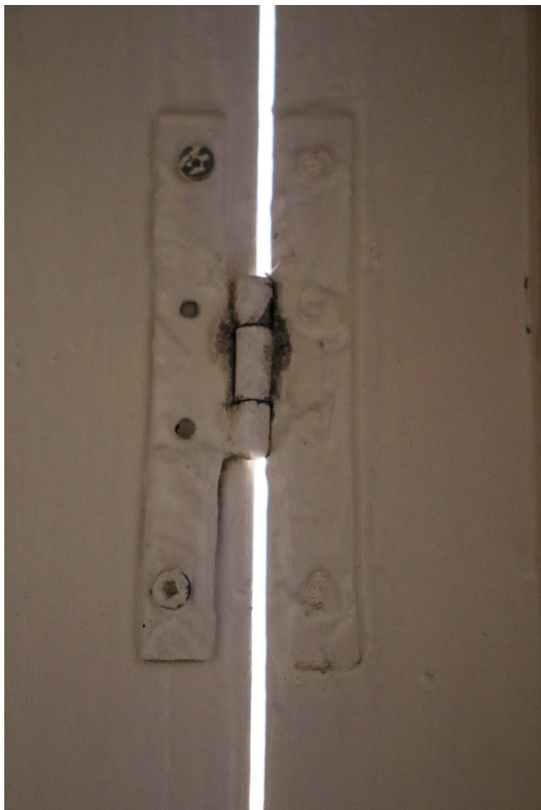
Plate 11 The house ground floor south-west room original shutter hinge
