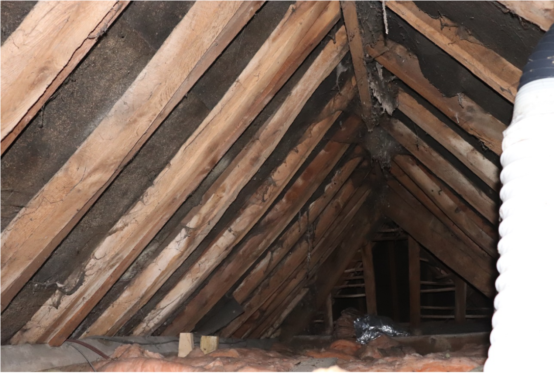
Plate 32 The house second floor, roof structure
