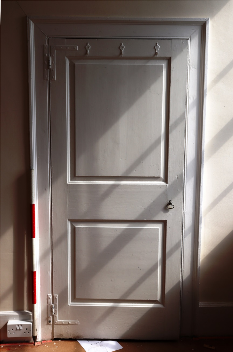
Plate 22 The house first floor with original thin 2 panel door and hinges, south-east room, looking east, scale 1m
