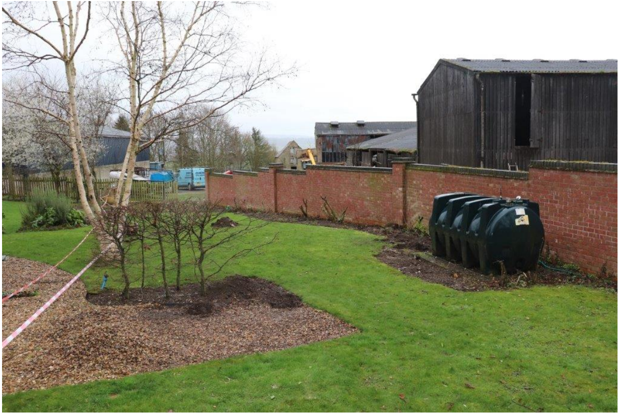
Plate 1: General view south-east of the garden before start of groundworks, no scales
