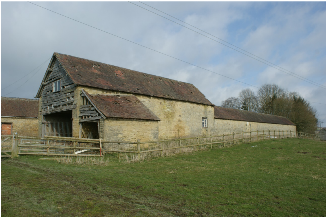
Plate 26 Barn 2, Phase 3 cart shed, stable and storage building, looking north-west (1m scale)
