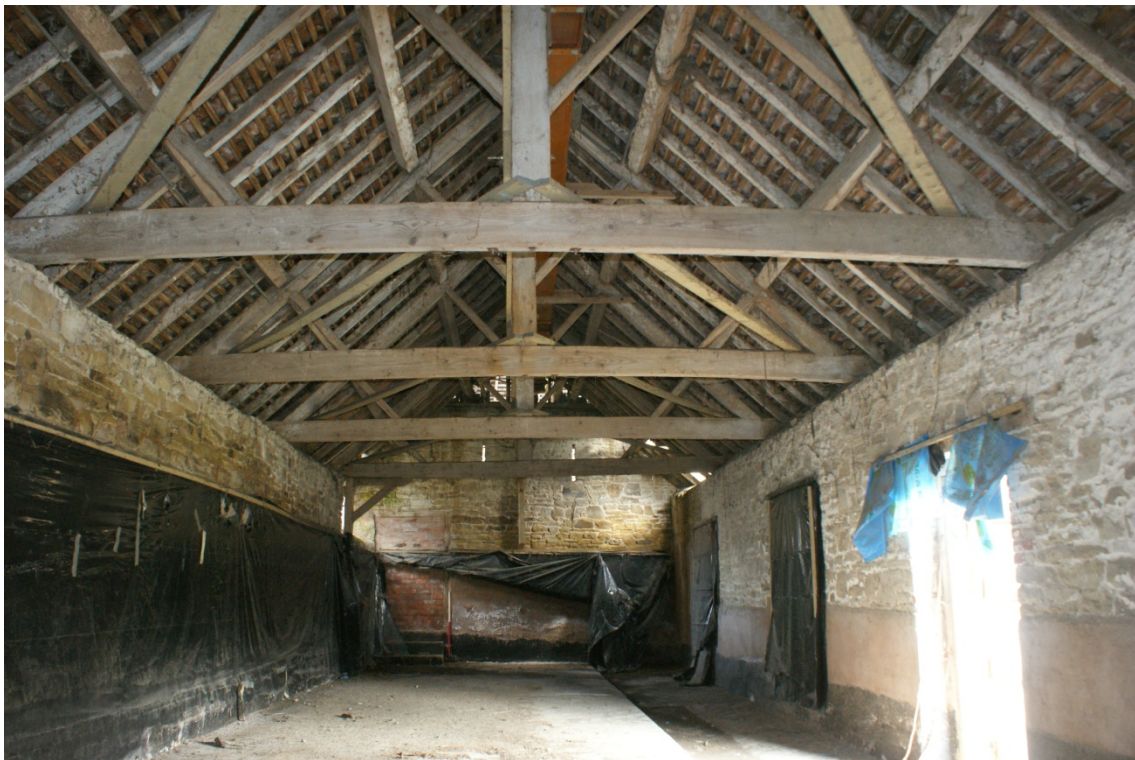
Plate 22 Barn 1, Phase 3 cow house, looking north-east (1m scale)
