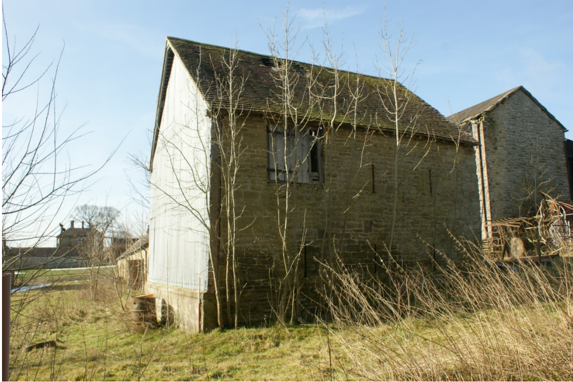
Plate 8 Phase 2 barn, looking south-west, at north end of Barn 1 (1m scale)
