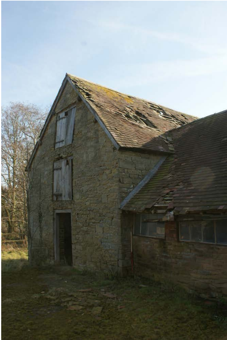
Plate 7 Phase 2 barn, looking north-east, at north end of Barn 1 (1m scale)
