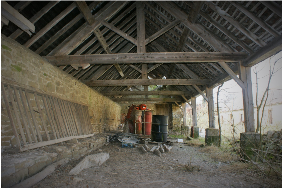
Plate 14 Barn 2, Phase 3 shelter shed, looking south-west (1m scale)
