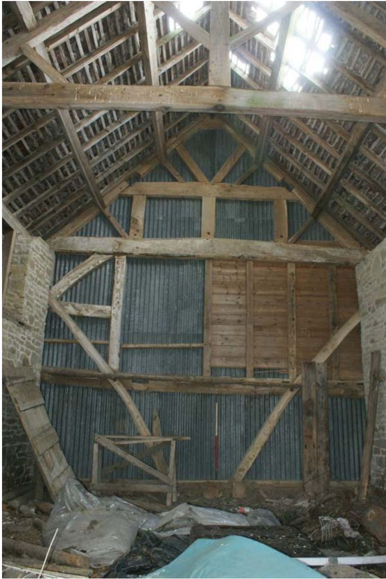
Plate 4 Phase 1 truss, looking east in north end of Barn 1 (1m scale)
