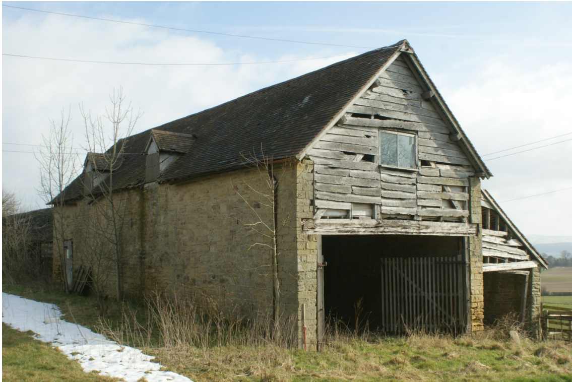
Plate 25 Barn 2, Phase 3 cart shed, stable and storage building, looking north-east (1m scale)
