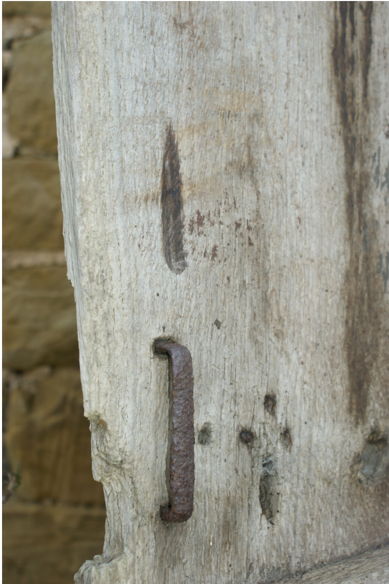
Plate 29 Barn 2, candle burn mark on the interior of the door into the Phase 3 cart shed, stable and storage building, looking south-east (no scale)
