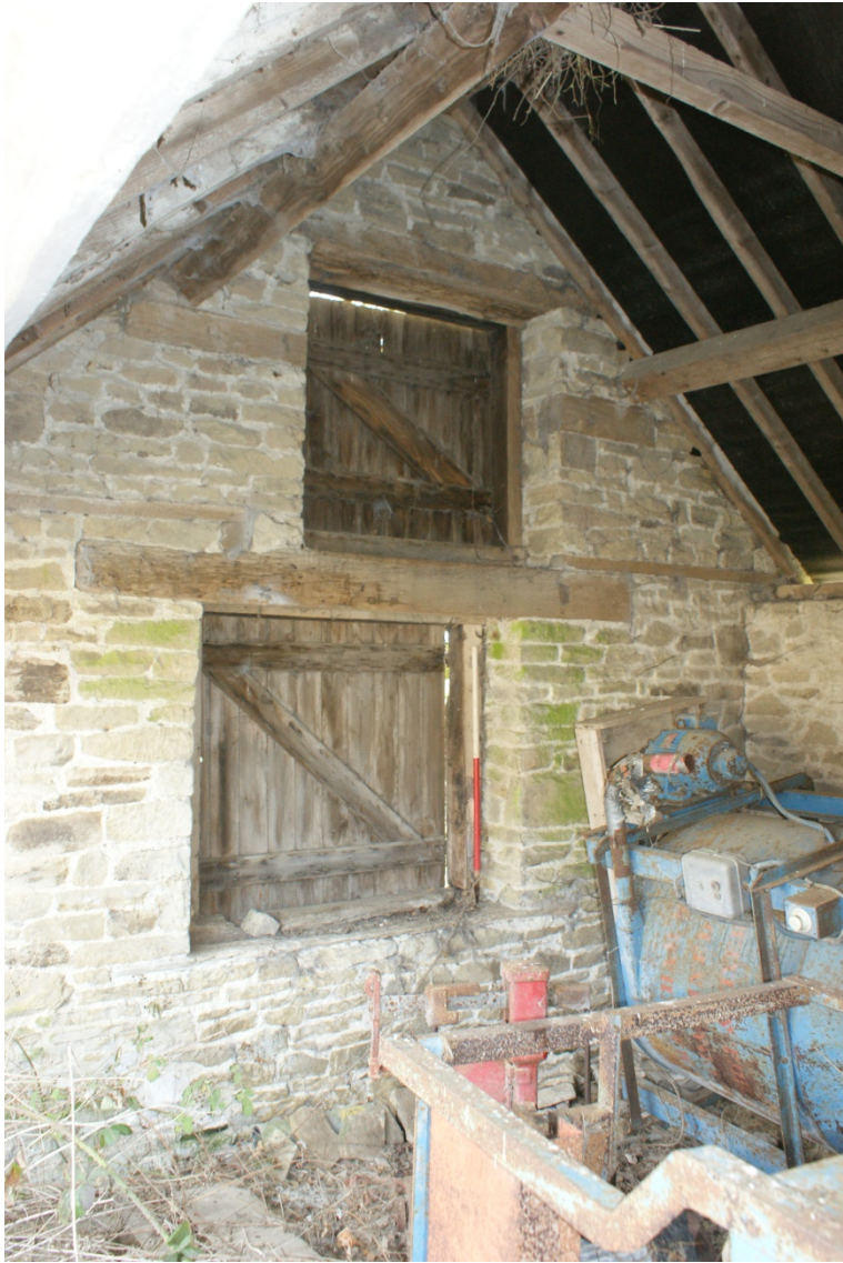
Plate 13 Barn 2, Phase 3 shelter shed, looking north-east (1m scale)
