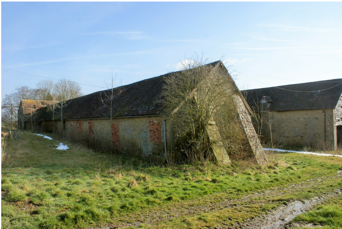
Plate 20 Barn 1, Phase 3 cow house, looking north-east (1m scale)
