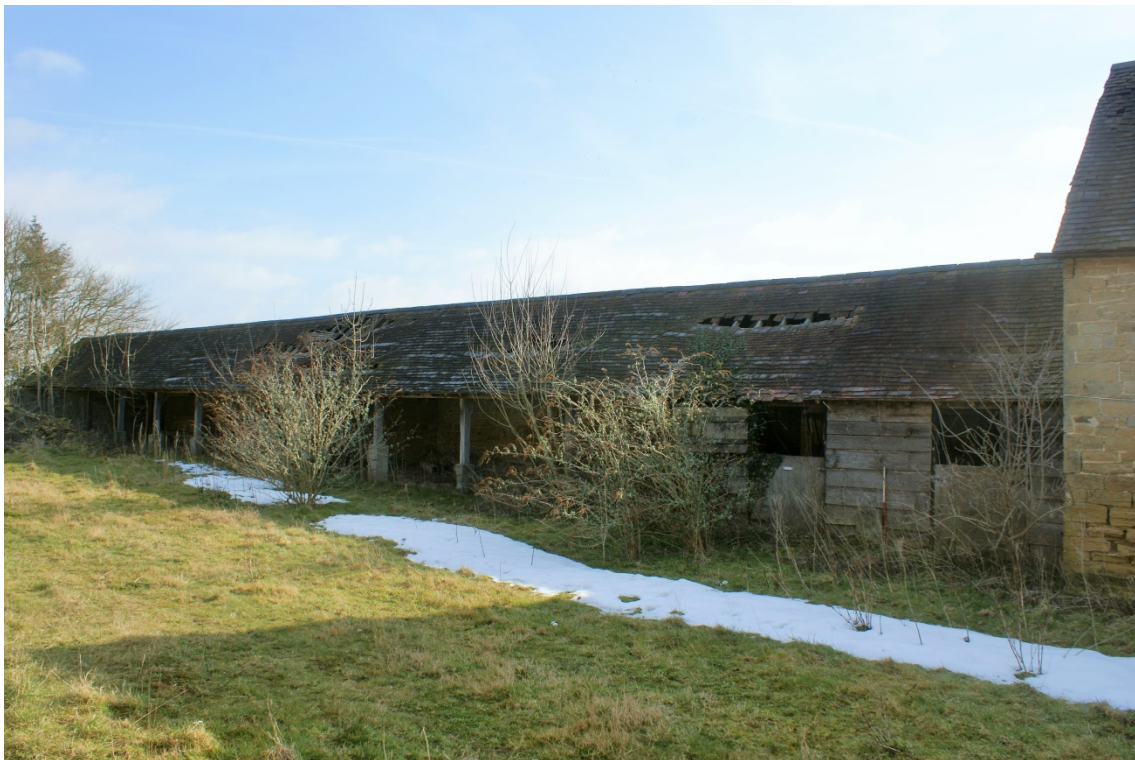
Plate 11 Barn 2, Phase 3 shelter shed, looking north-east (1m scale)
