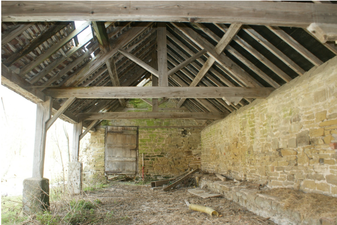
Plate 17 Barn 2, Phase 3 shelter shed, looking north-east (1m scale)
