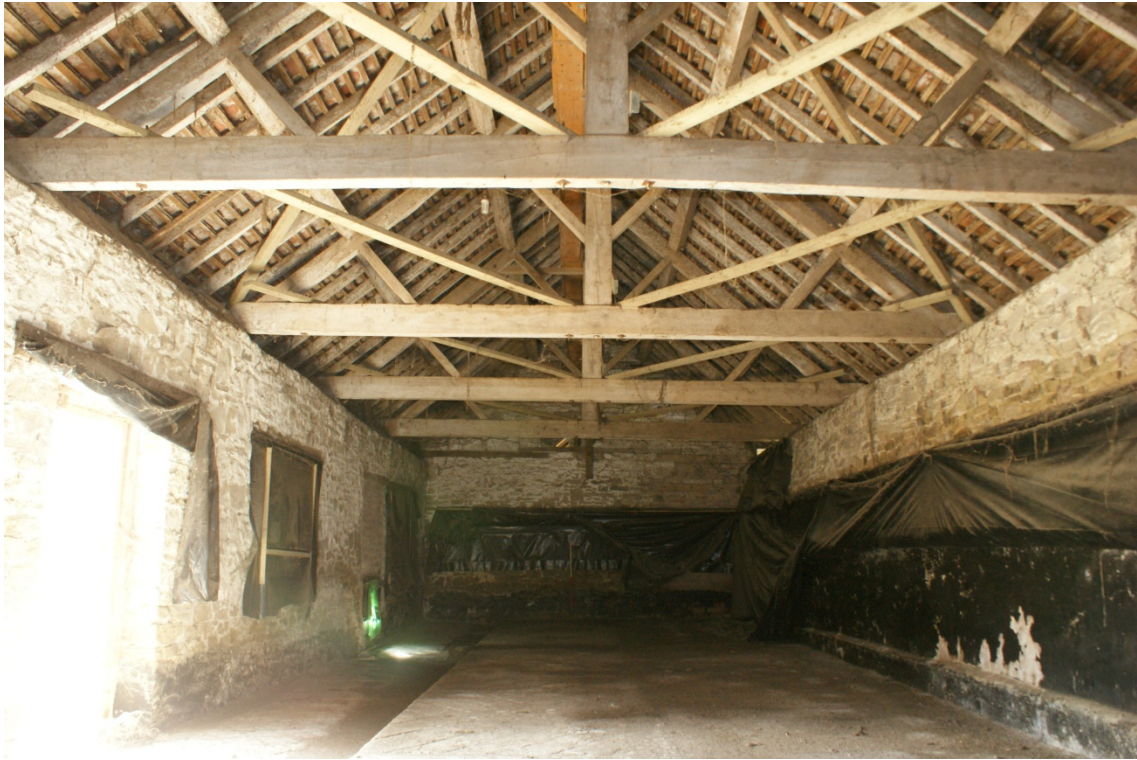
Plate 23 Barn 1, Phase 3 cow house, looking south-west (1m scale)
