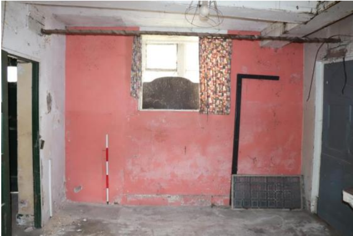
Plate 95 Phase 2 room G20, looking north-west, scale 1m
