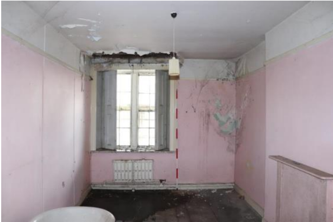
Plate 140 Room S6a, looking north-east, scale 2m
