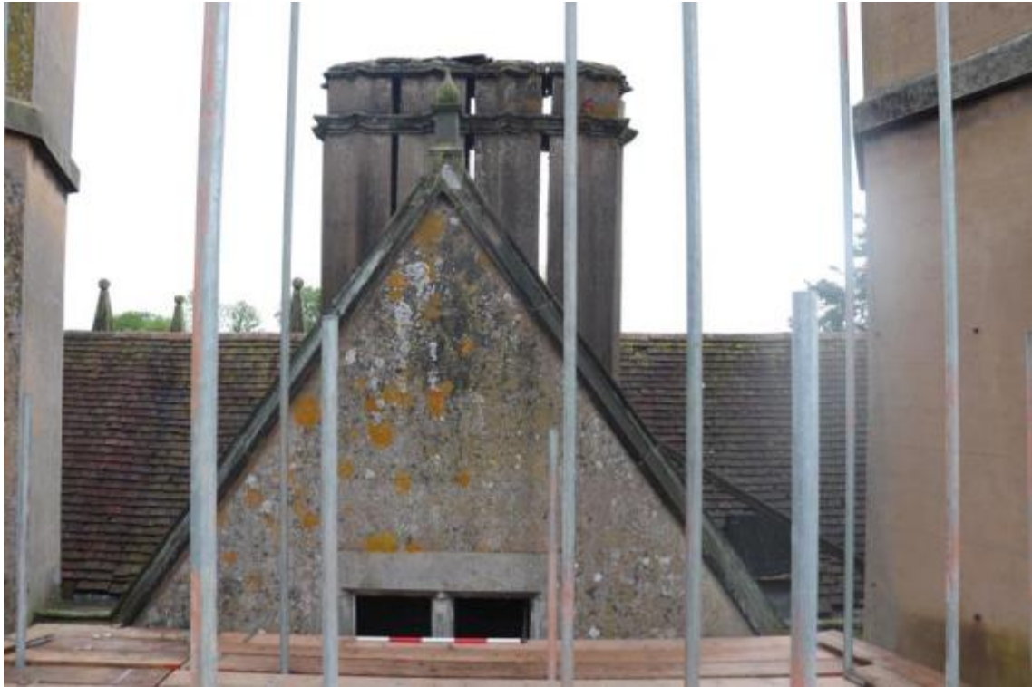
Plate 110 Phase 3 stone and chimney detailing, looking north-east, scale 1m
