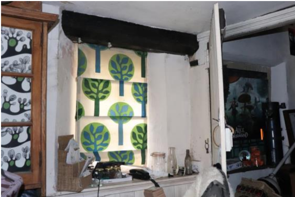
Plate 105 Phase 2 gable end window position in room G24, looking north-east, no scale
