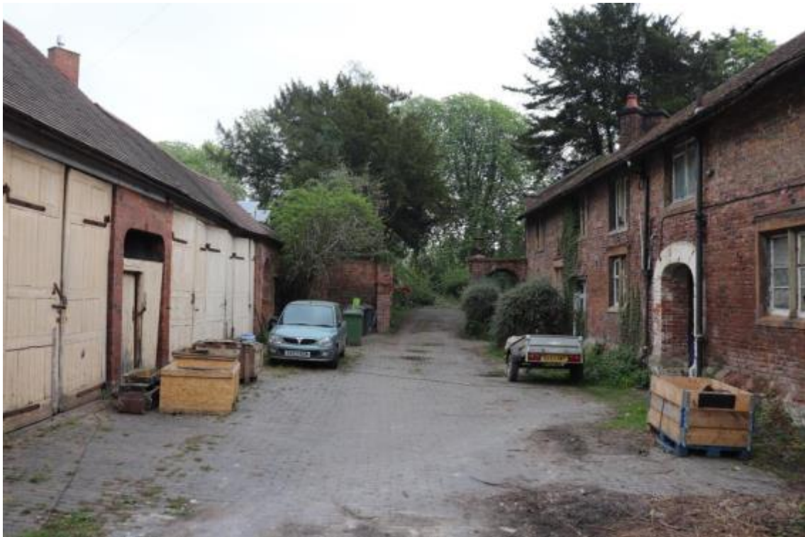
Plate 80 Phase 2 north-east to south-west aligned service wing on the right with later buildings on the left, looking north-east
