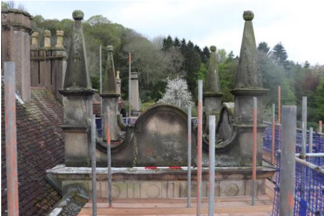
Plate 112 Phase 3 decorative details above the porch, looking north-west, scale 1m
