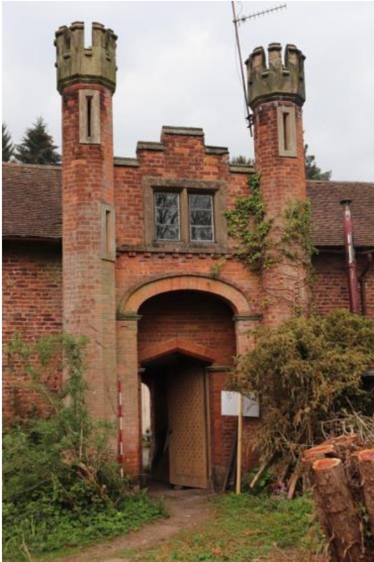
Plate 156 Phase 5 addition to the service wing, looking north-west, scale 2m
