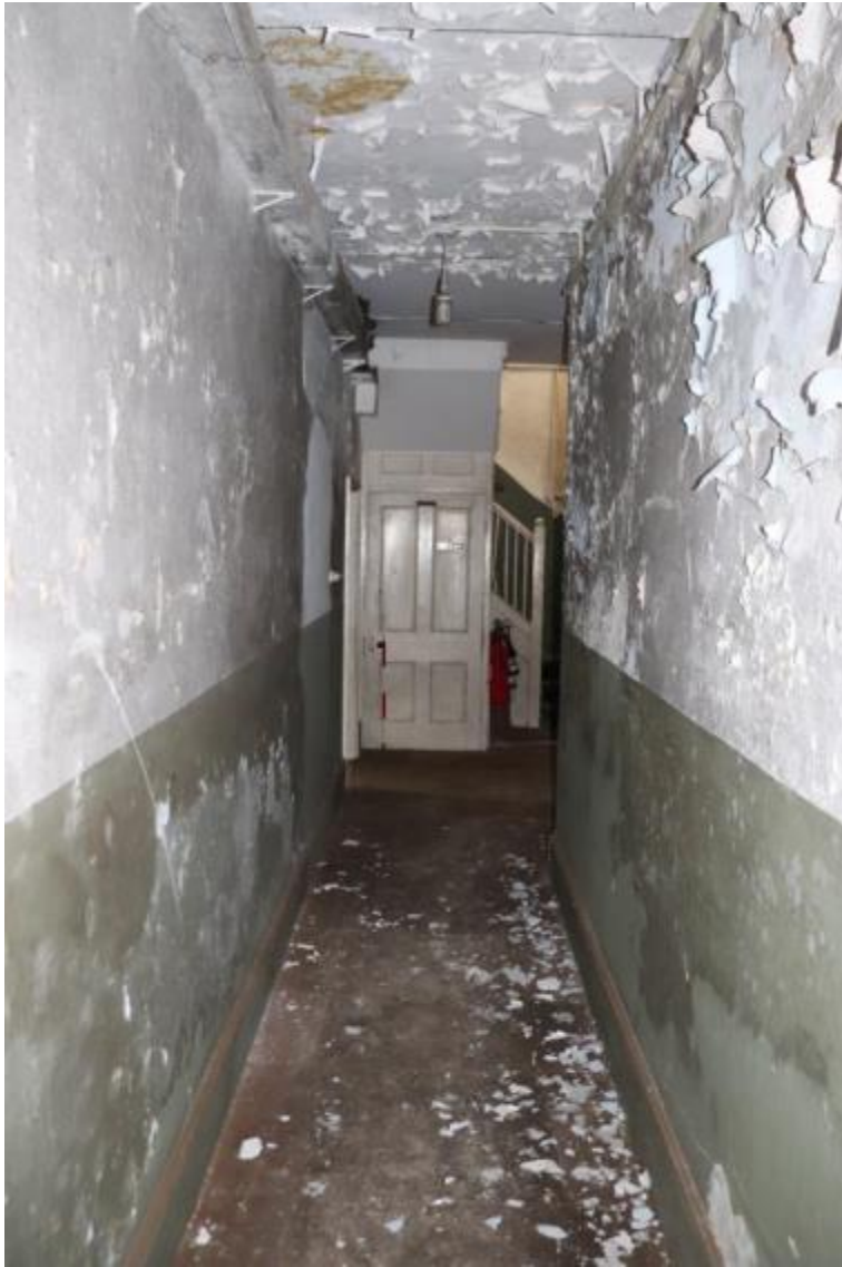
Plate 148 Phase 4 room G11, looking south-east, scale 1m
