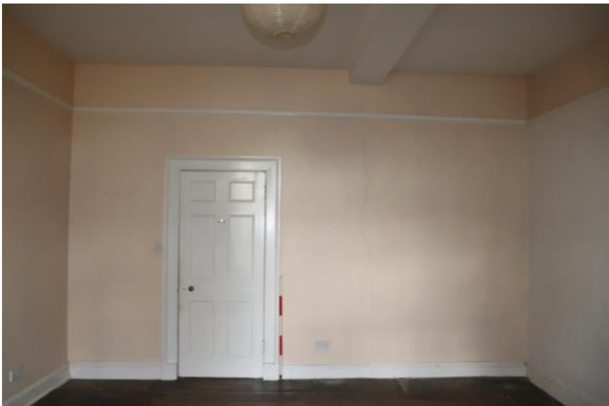
Plate 51 Room F2, looking south-east, scale 1m
