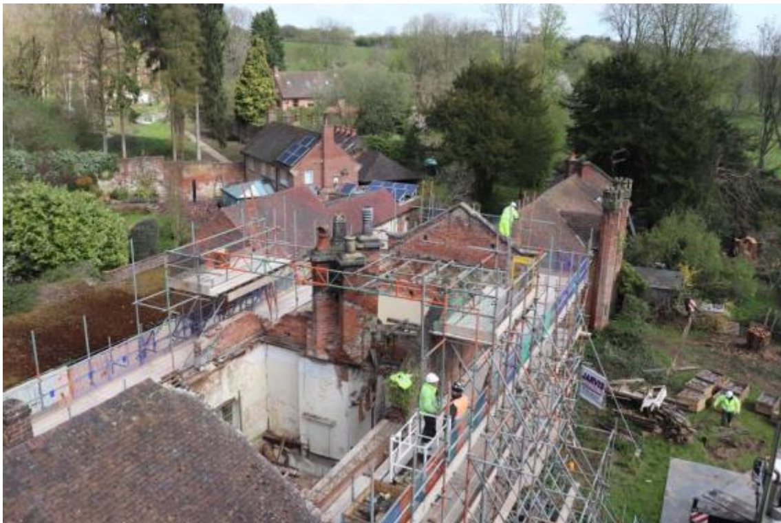
Plate 78 Phase 2 north-east to south-west aligned service wing, looking north
