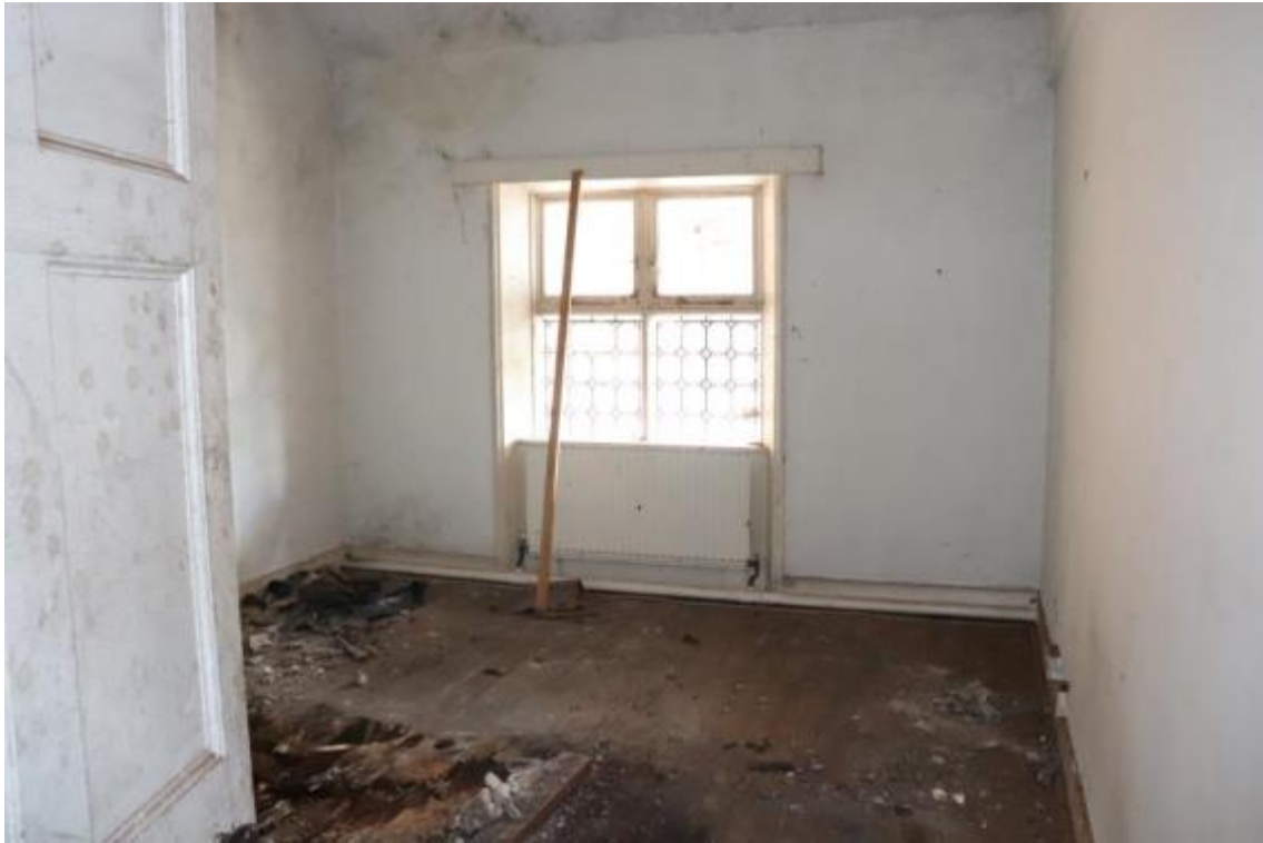
Plate 155 Phase 4 room F18, looking north-east, no scale
