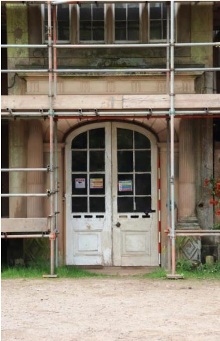
Plate 124 Phase 3 porch, looking south-west, scale 2m
