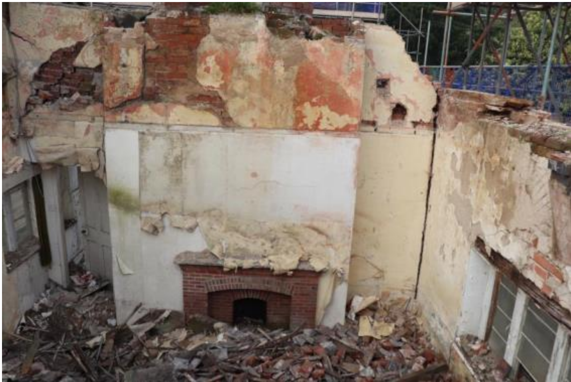
Plate 92 Phase 2 room F17, looking south-east, no scale
