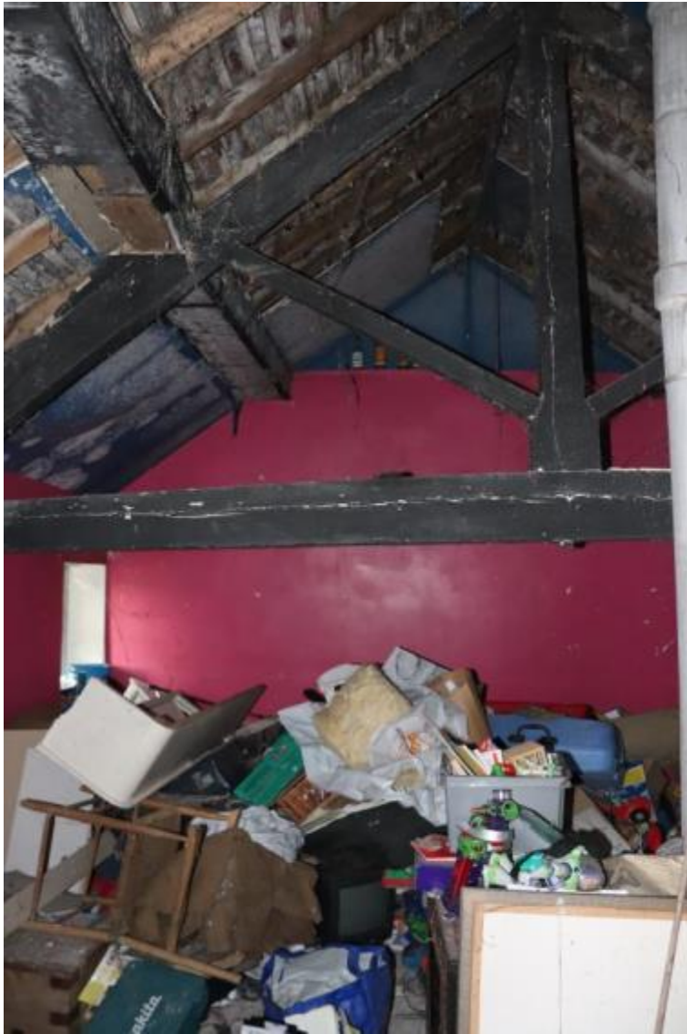
Plate 100 Phase 2 room F20a, looking south-west, no scale
