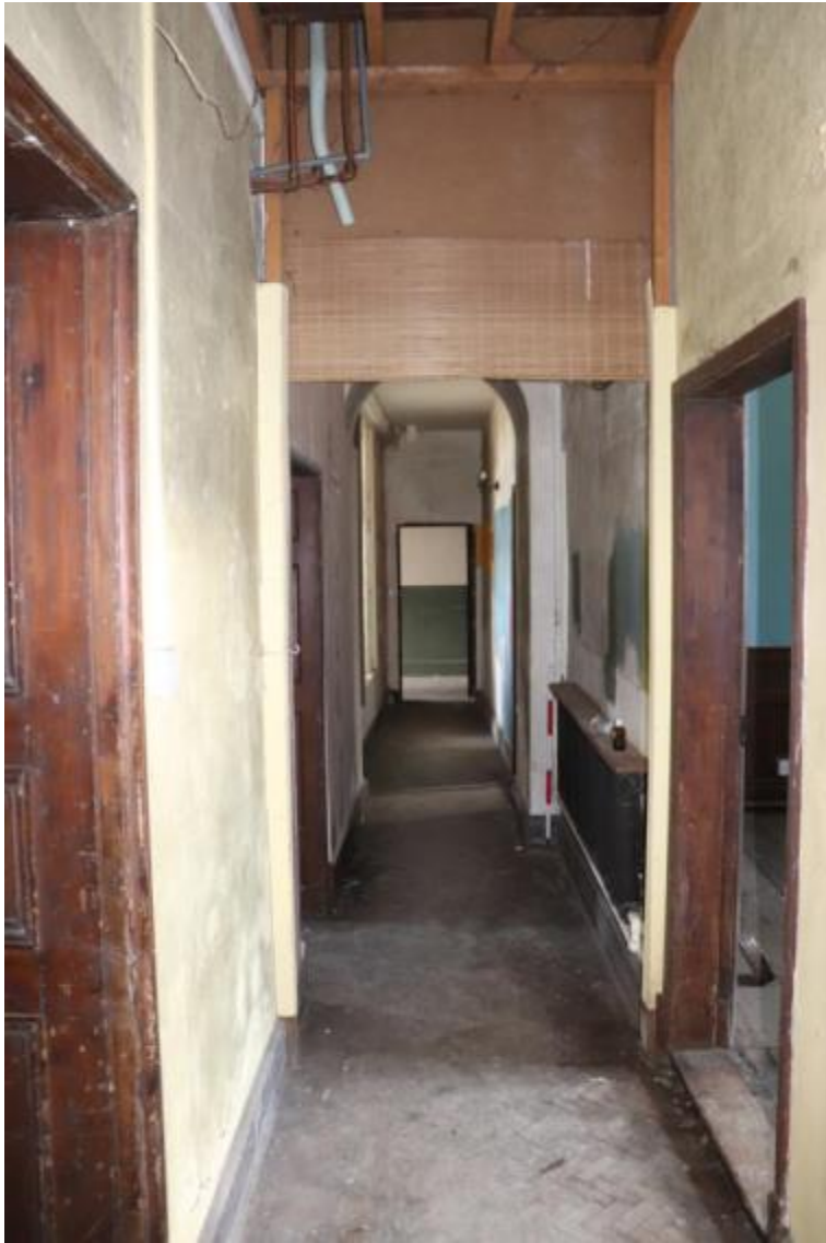
Plate 66 Phase 2 corridor G7b, looking south-east, scale 1m
