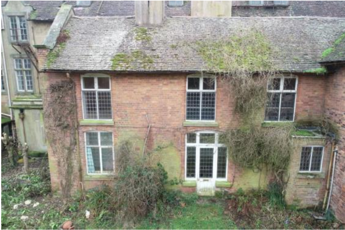
Plate 146 Phase 4 building exterior, looking south-west, no scale
