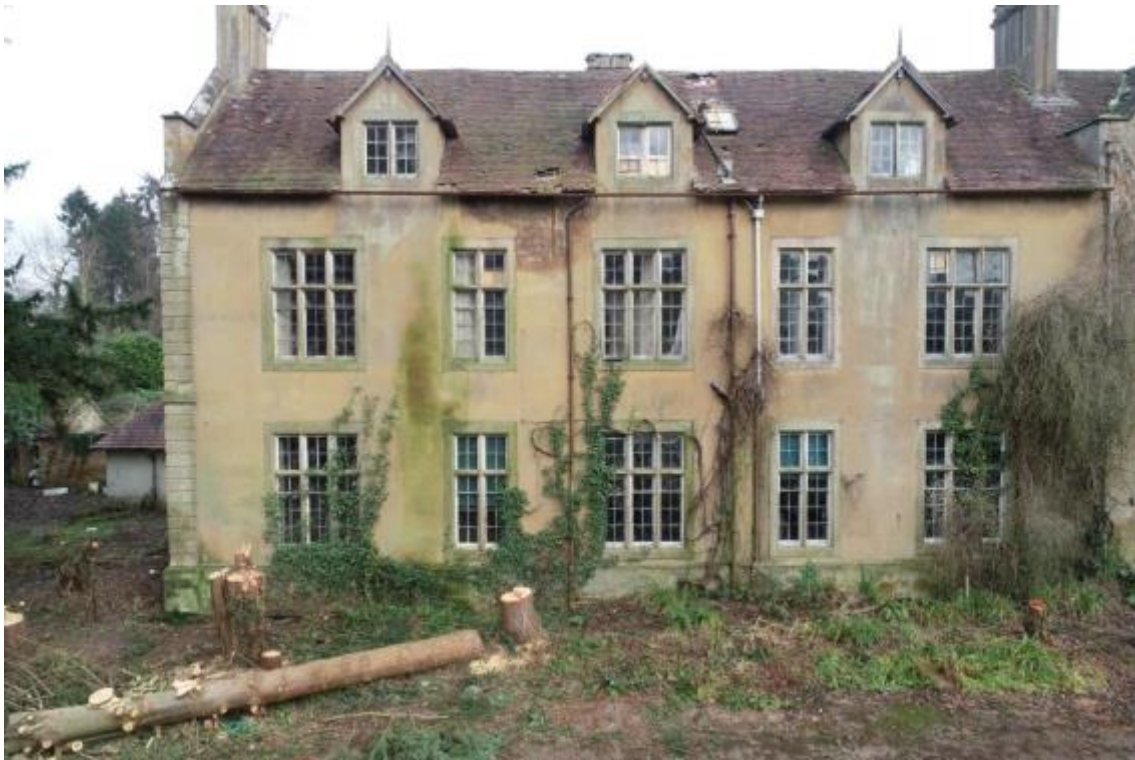
Plate 57 Phase 2 service element, looking north-east
