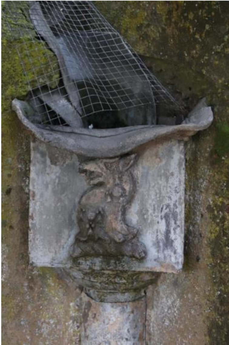
Plate 113 Phase 3 Lead drain pipe hopper detail, looking north, no scale
