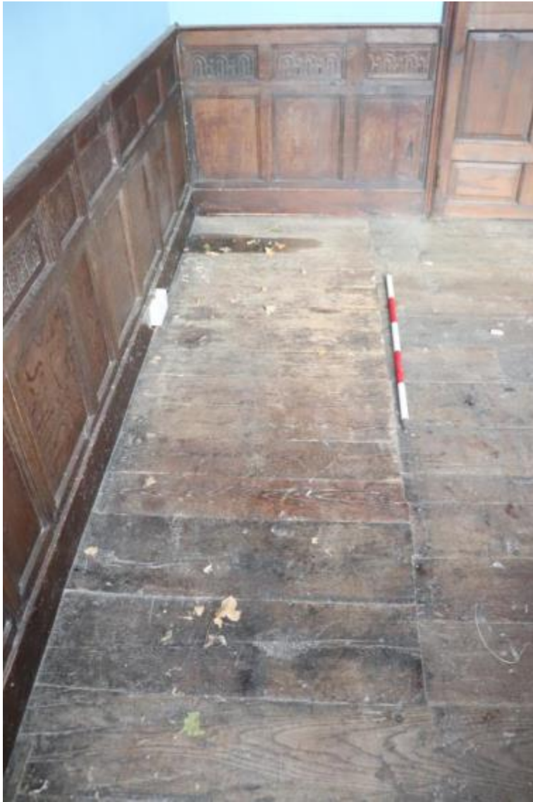
Plate 76 break in the floor boards over the stairs below; see Plate 75, looking north-east, scale 1m
