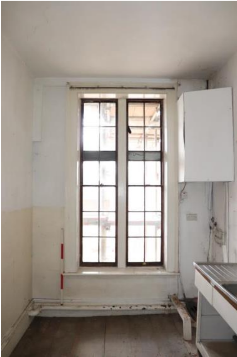
Plate 133 Room F9b, looking north-east, scale 1m
