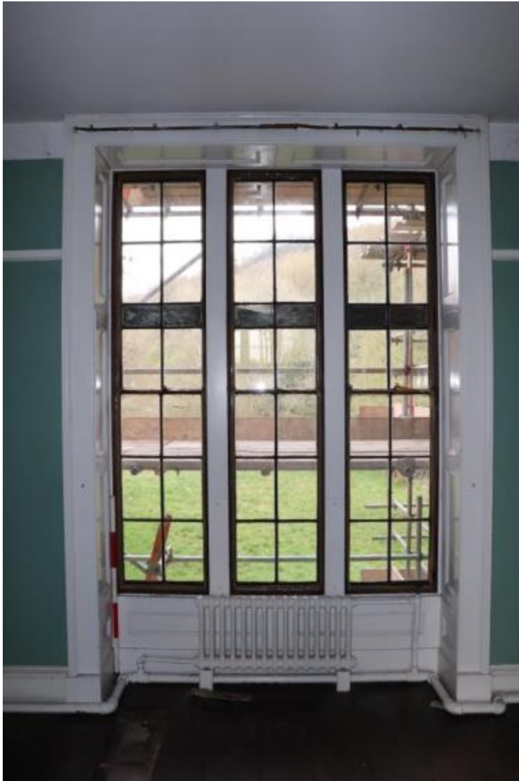
Plate 116 Phase 3 internal window, room F1, looking south-west, scale 1m
