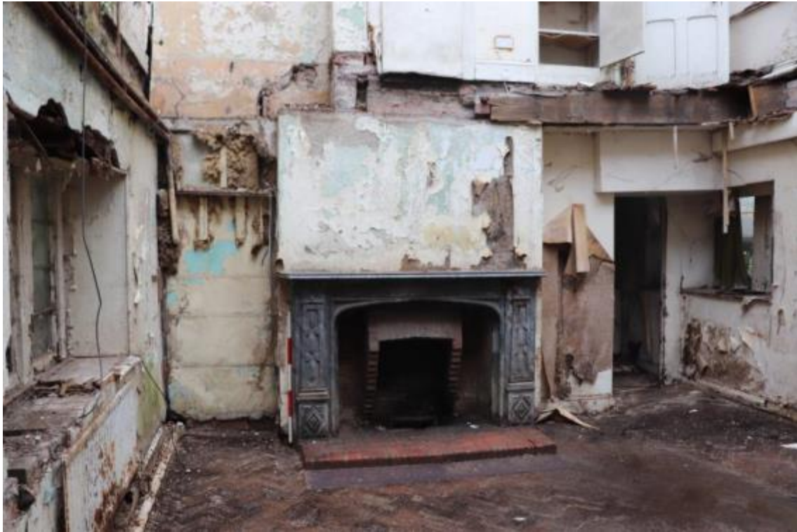
Plate 85 Phase 2 Room G16, looking north-east, scale 1m
