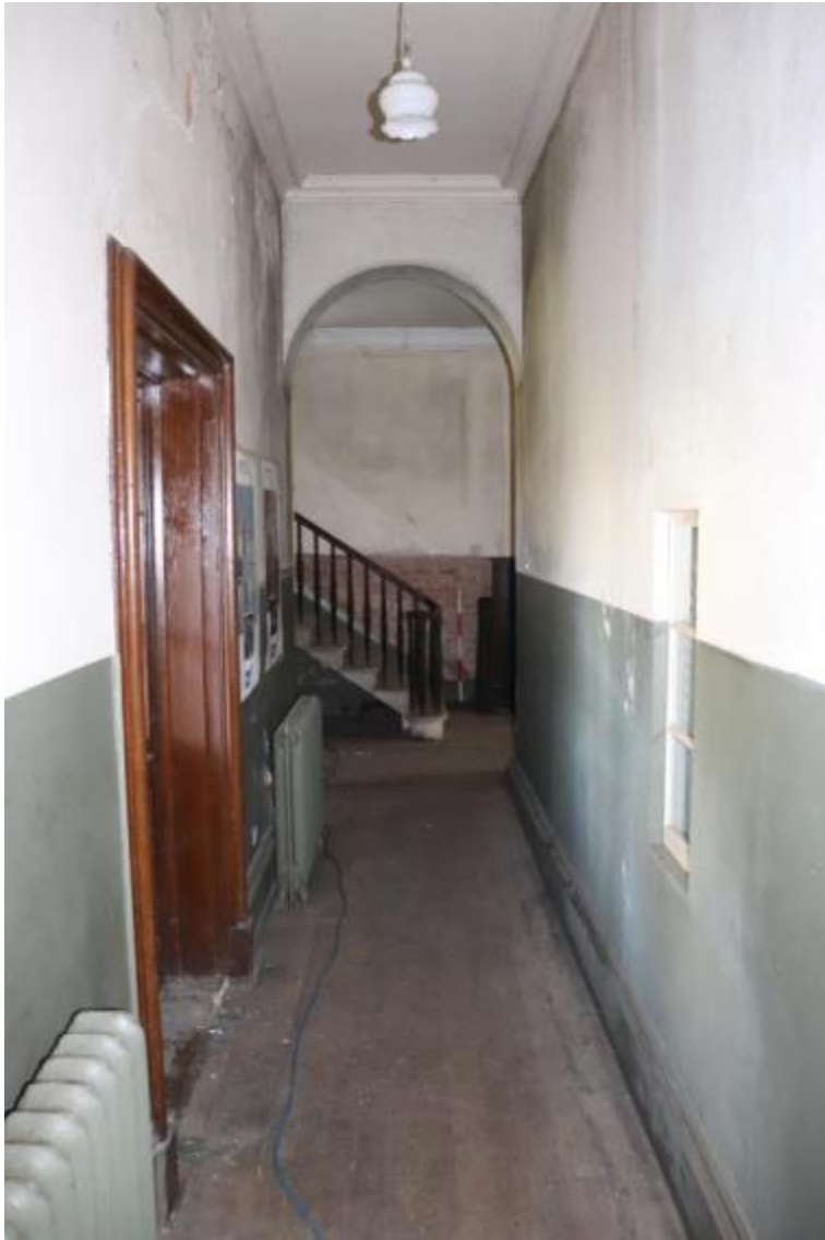
Plate 43 Corridor G3a inserted through the former position of the Phase 1 fireplace, looking north-west, scale 1m
