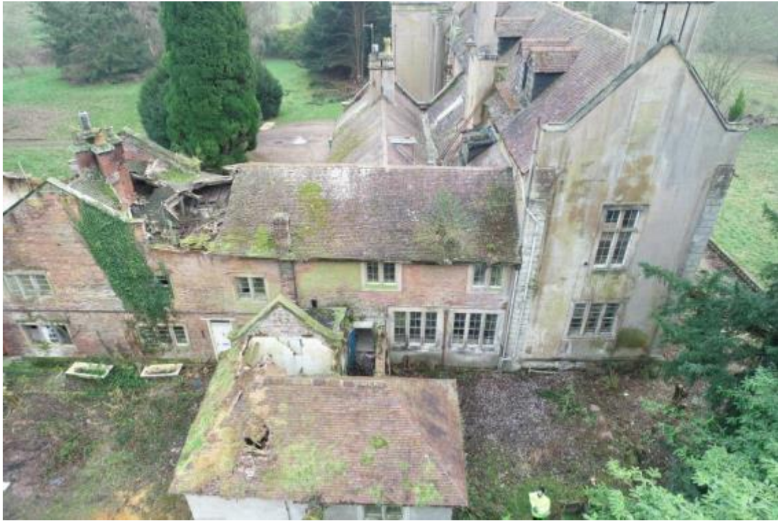
Plate 58 Phase 2 service element gable end, looking south-east
