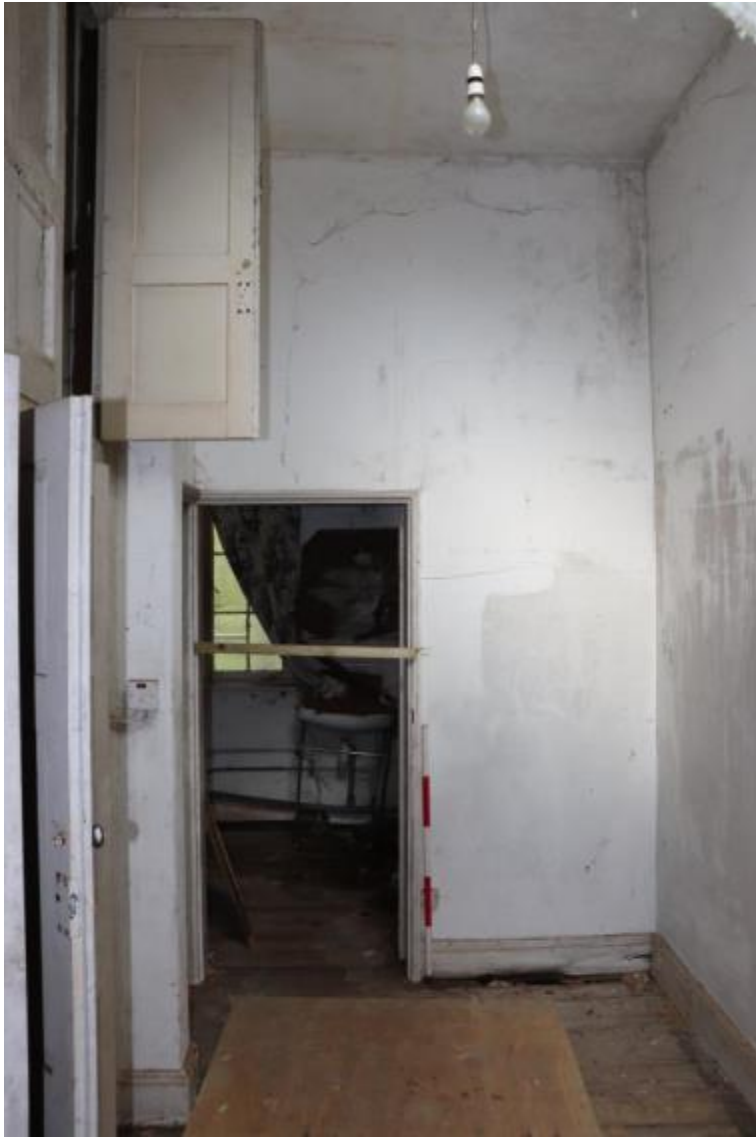
Plate 82 Phase 2 room F14d, looking north-west, scale 1m
