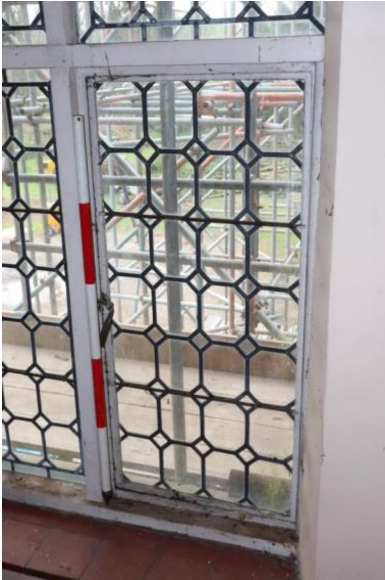
Plate 166 Phase 6 inserted metal frame casement windows within room F16, scale 1m, looking east
