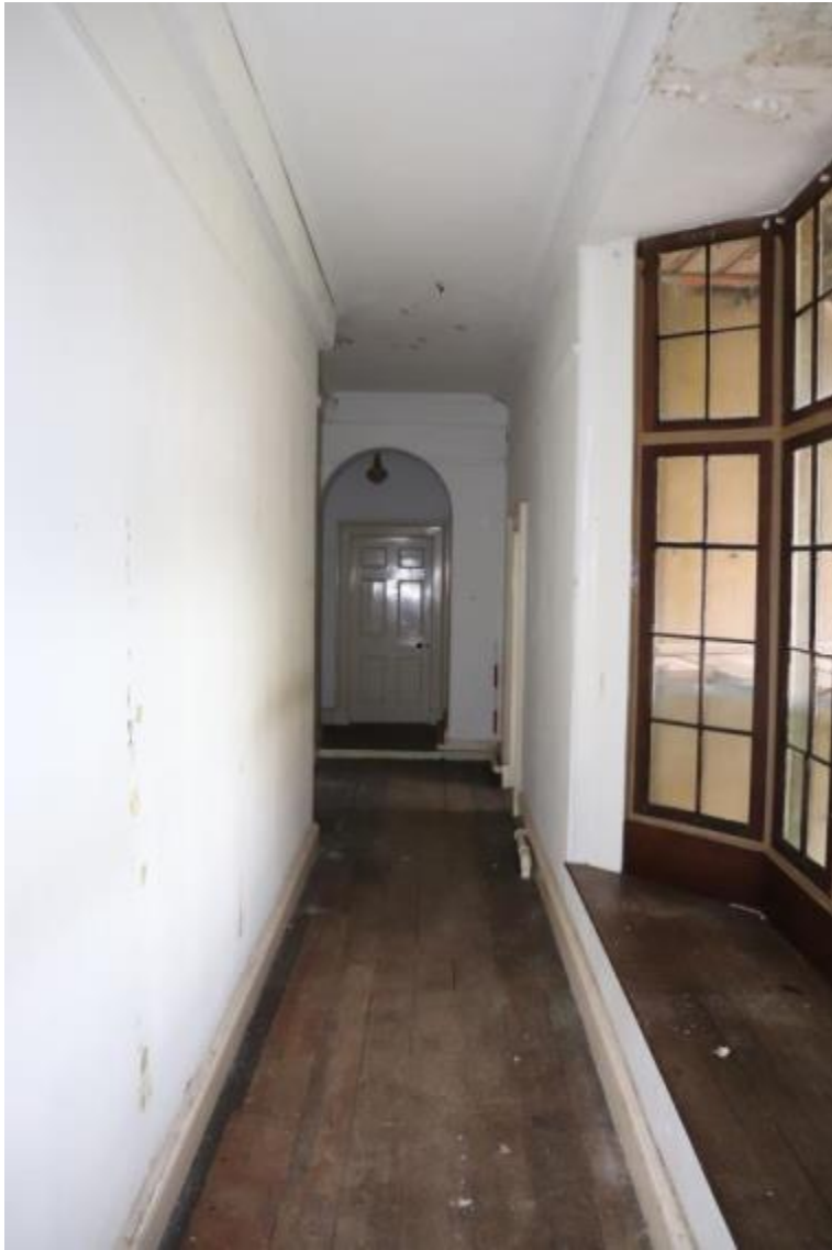
Plate 53 Room F4, looking south-east, scale 1m
