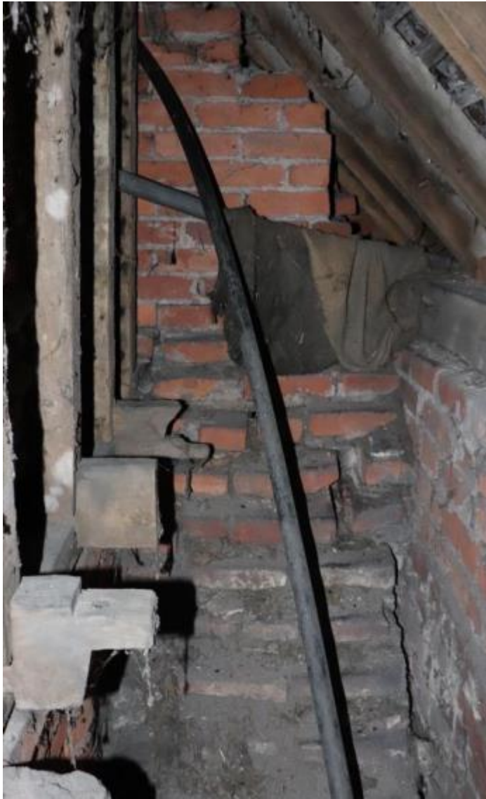
Plate 71 Phase 2 redundant chimney breast visible from within room S14b, looking north-west, no scale
