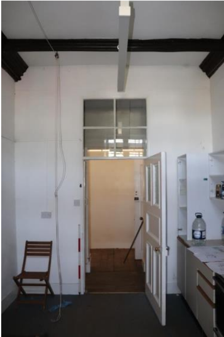
Plate 48 Room G2b, looking south-west, scale 1m
