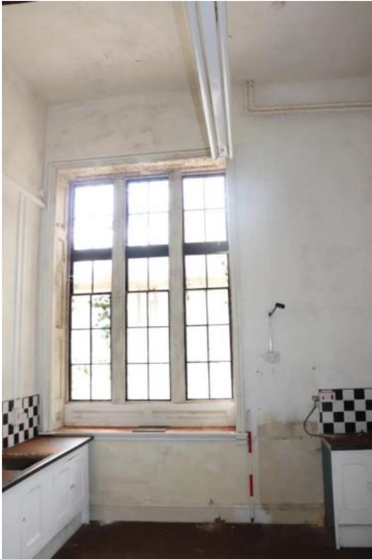
Plate 69 Phase 2 room G9a, former brewhouse, looking south-west, scale 1m
