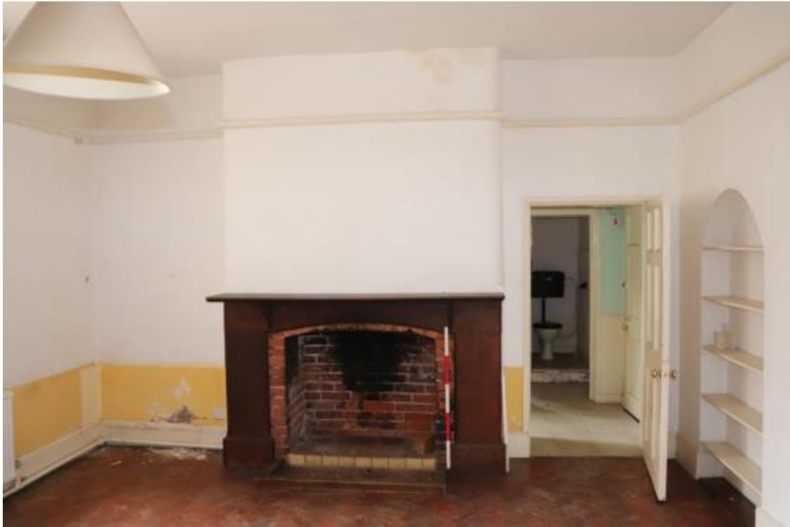
Plate 151 Phase 4 Room G13, looking south east, scale 1m
