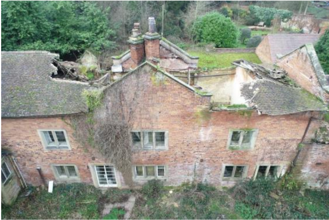
Plate 108 Phase 3 raised roof elements over earlier Phase 2 wing, looking north-west
