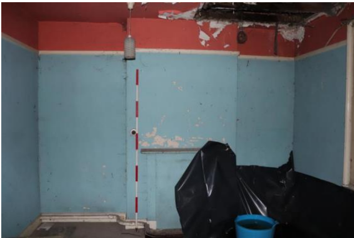
Plate 139 Room S2, looking south-east, scale 2m
