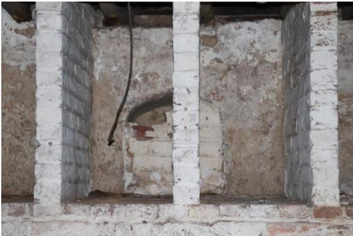
Plate 46 Phase 1 cellar with a blocked niche behind later shelving, looking south-east
