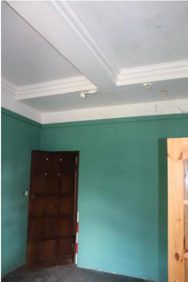
Plate 49 Room G5a, with mouldings on the ceiling potentially concealing Phase 1 beams, looking north, scale 1m
