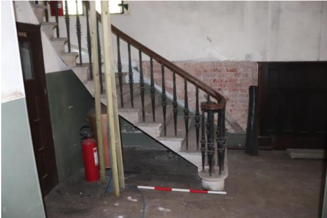
Plate 125 Phase 3 staircase, ground floor, looking east, scale 1m
