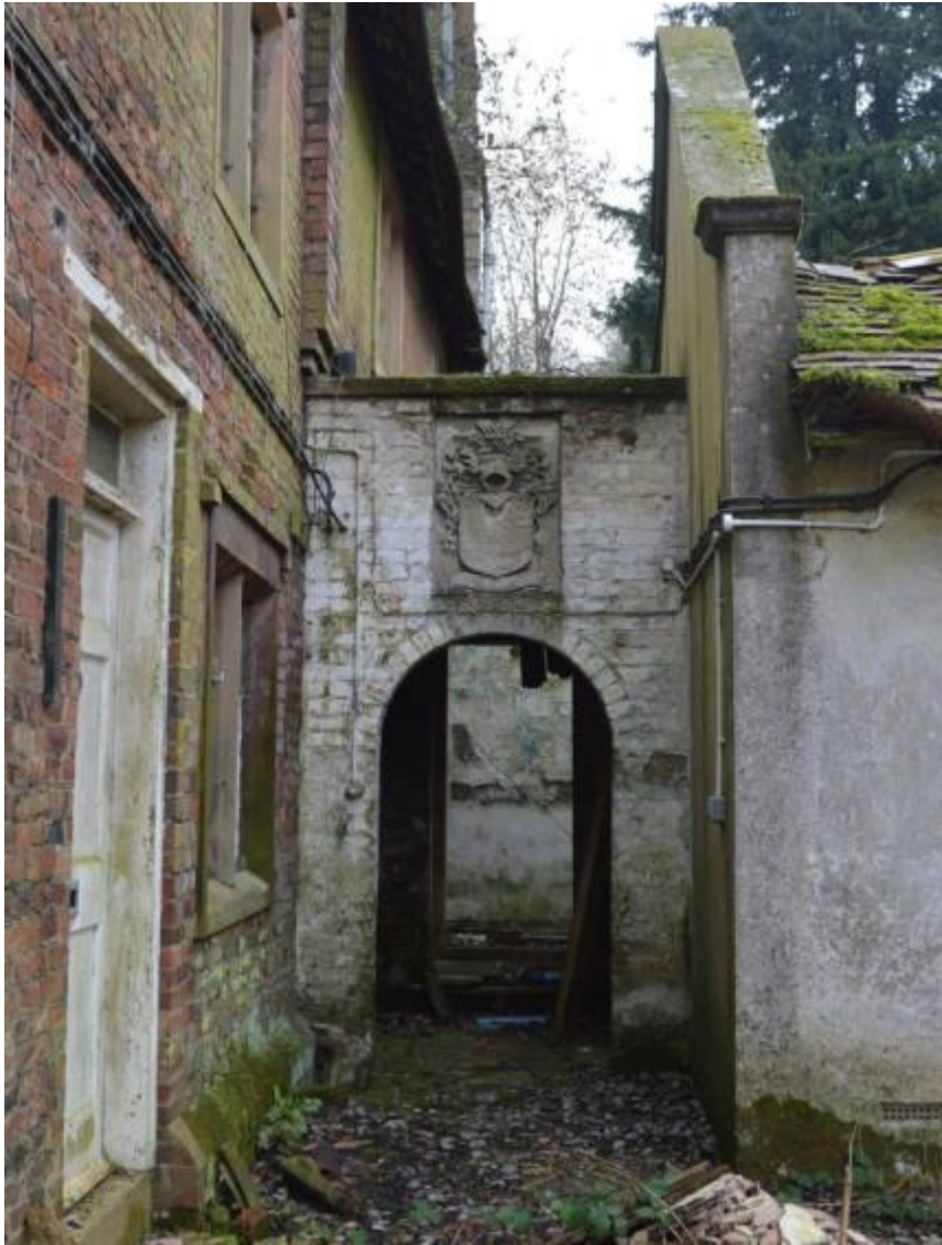
Plate 152 Phase 4 exterior extension, looking south-west, no scale
