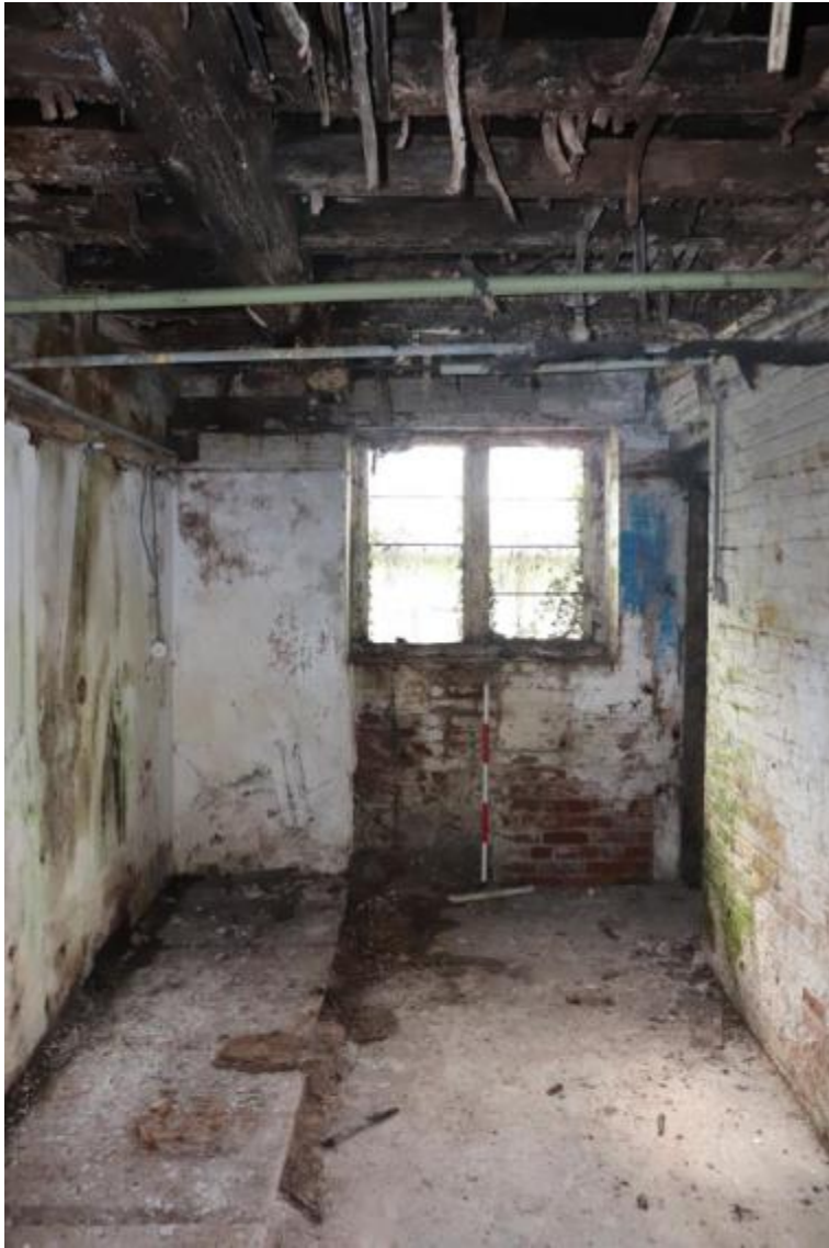
Plate 89 Phase 2 room G18, looking south-east, scale 1m
