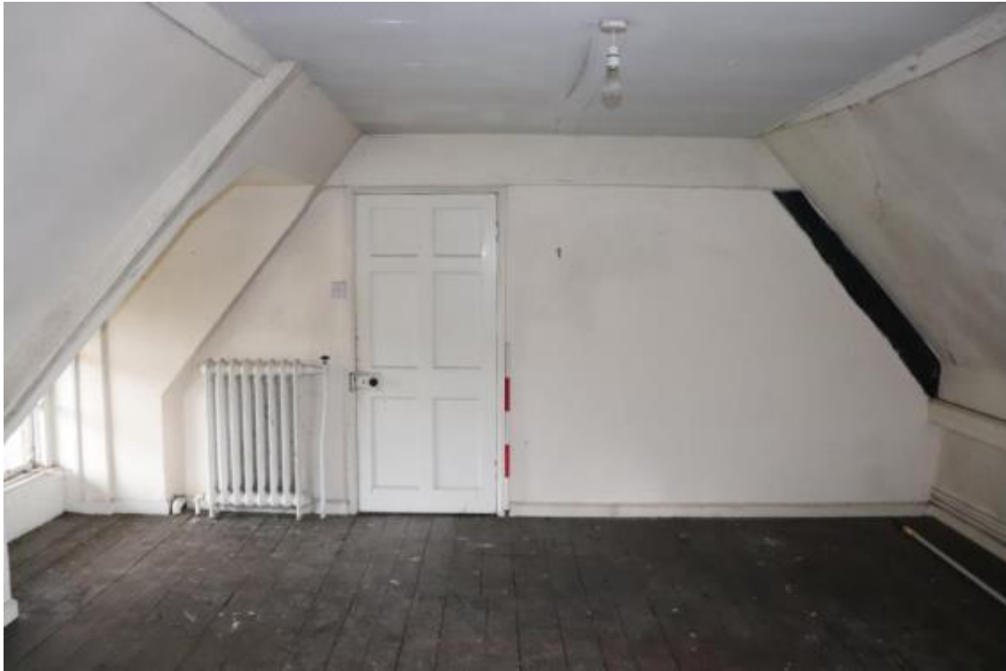
Plate 60 Phase 2 Room S11, looking north-west, scale 1m
