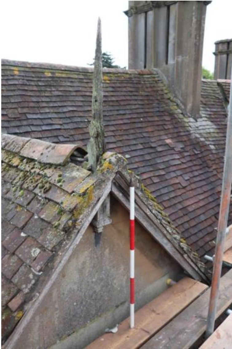
Plate 111 Phase 3 timber finial detail above inserted dormer window on the Phase 2 structure, looking north-east, scale 1m
