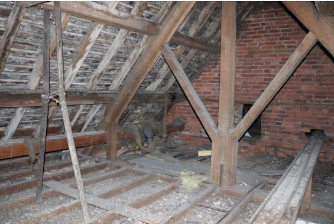
Plate 107 Phase 3 roof truss visible above room S10, looking south-east, no scale
