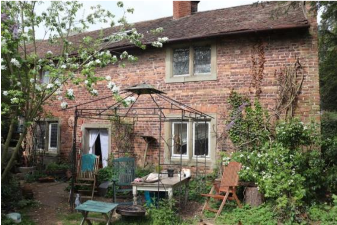
Plate 79 Phase 2 north-east to south-west aligned service wing, looking west
