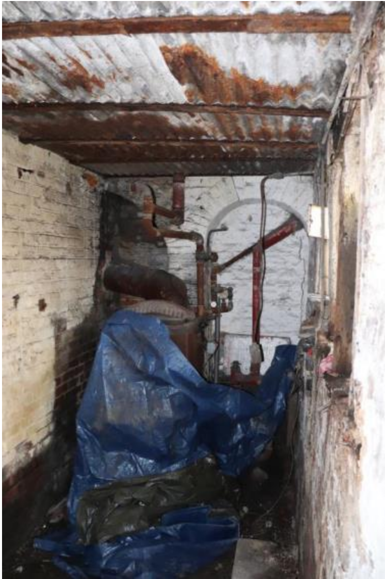
Plate 88 Phase 2 room G17b, looking south-west, no scale
