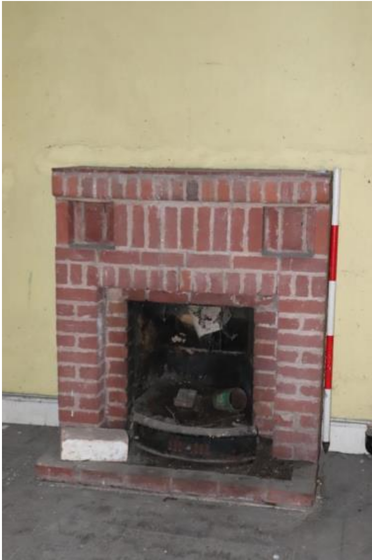
Plate 171 Phase 7 inserted fireplace room S10a, looking north-west, scale 1m
