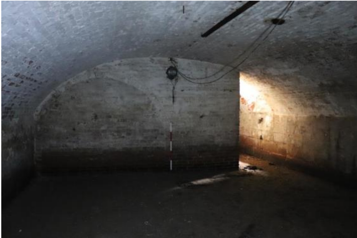
Plate 72 Phase 2 cellar, looking south-east, scale 1m
