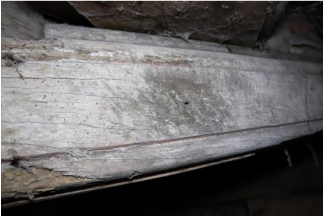
Plate 56 Probable Phase 1 beam reused within the southern turret, with hints of red paint remaining within the mouldings; see Figure 12 for profile
