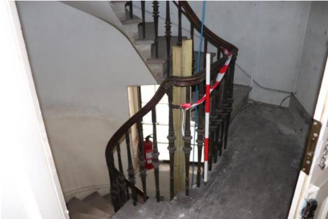
Plate 127 Phase 3 staircase, first floor, looking east, scale 1m
