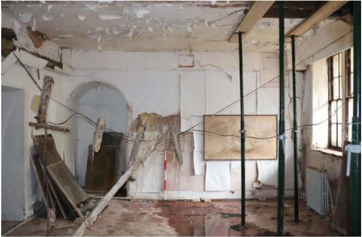
Plate 81 Phase 2 room G10, looking south-west, scale 1m
