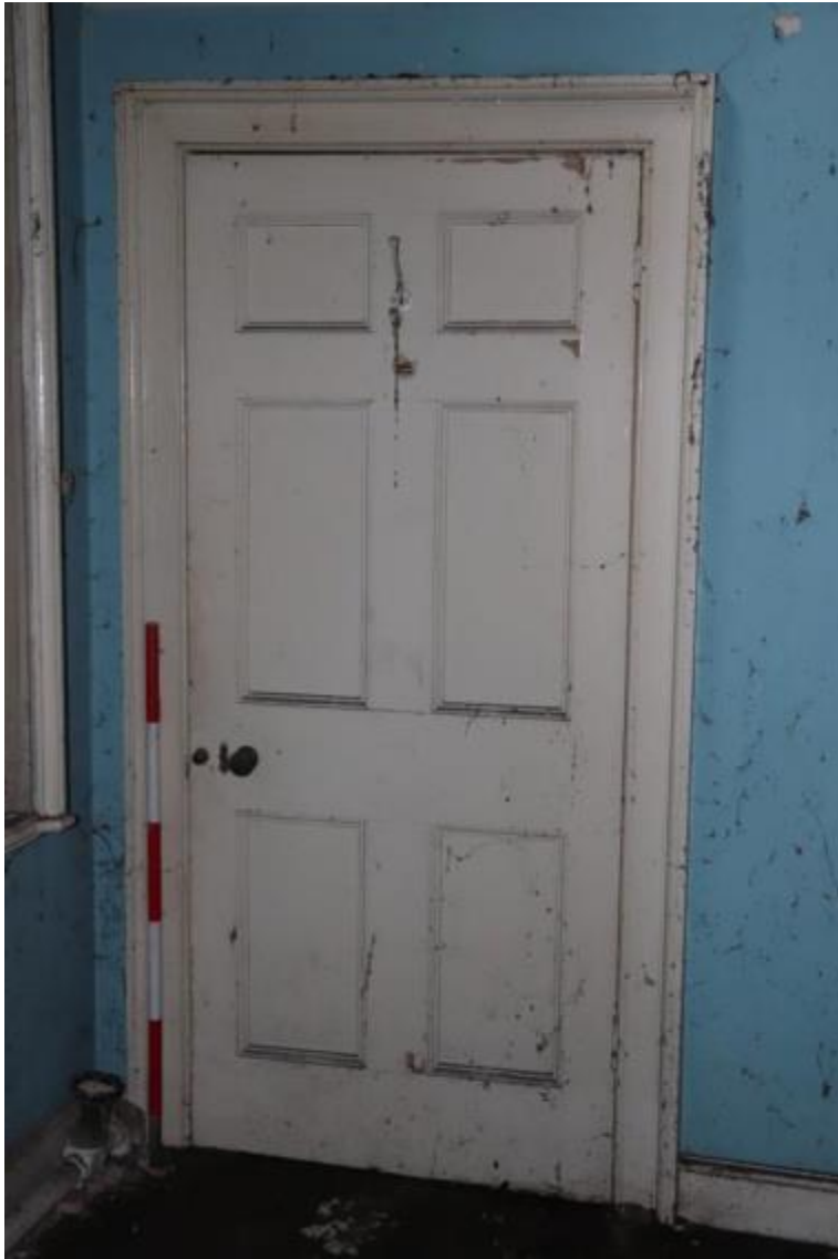
Plate 137 Typical Phase 3 second floor door, room S2, looking north-west, scale 1m
