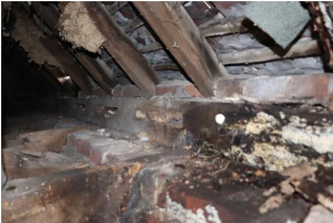
Plate 59 Phase 2 wall plate with regularly spaced mortices, looking north
