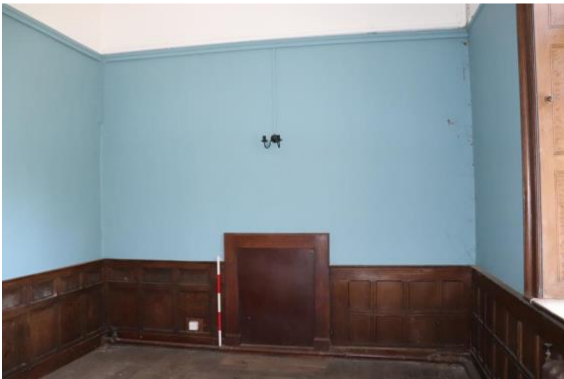
Plate 65 Phase 2 Room G7a, looking south-east, scale 1m
