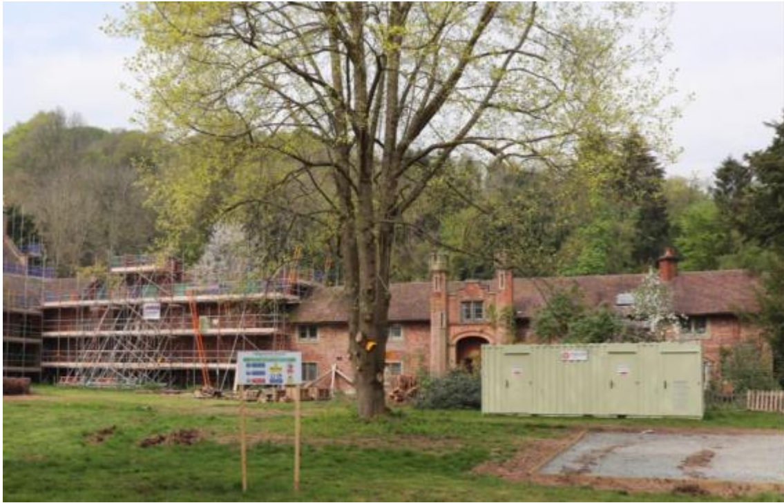
Plate 77 Phase 2 north-east to south-west aligned service wing, looking north-west
