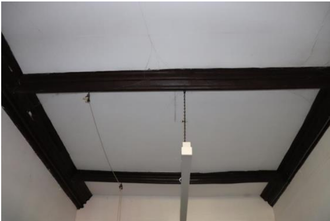
Plate 40 Phase 1 moulded ceilings beams within room G2c, looking north-east, no scale
