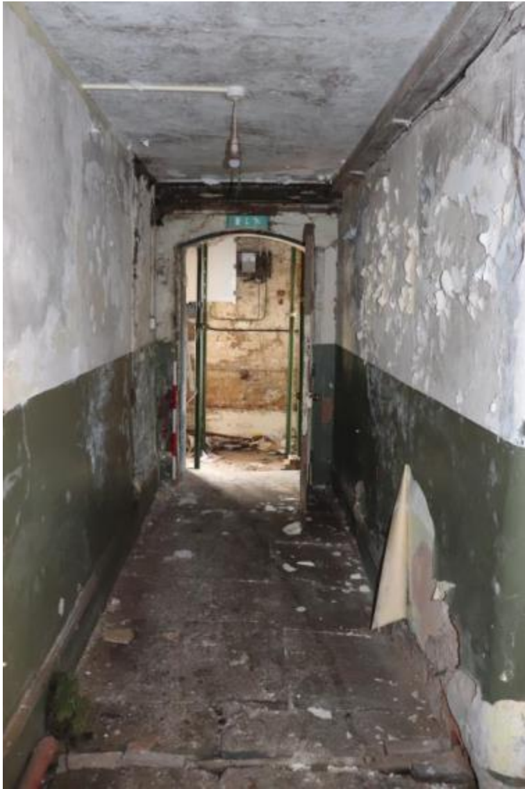
Plate 84 Phase 2 Room G14, looking south-east, scale 1m
