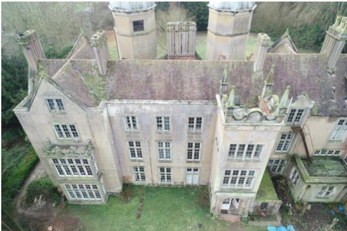
Plate 29 The house with the Phase 1 elements, rebuilt in Phase 3, on the left, and the Phases 2 and 4 elements to the right, looking south-west, no scale
