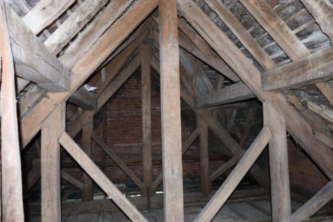
Plate 106 Phase 3 roof trusses visible above rooms S1-3, looking south-west, no scale
