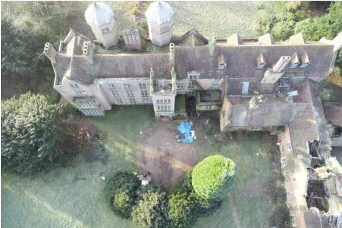
Plate 30 The house with the Phase 1 elements, rebuilt in Phase 3, on the left, and with the Phases 2 and 4 elements to the right, looking south-west, no scale
