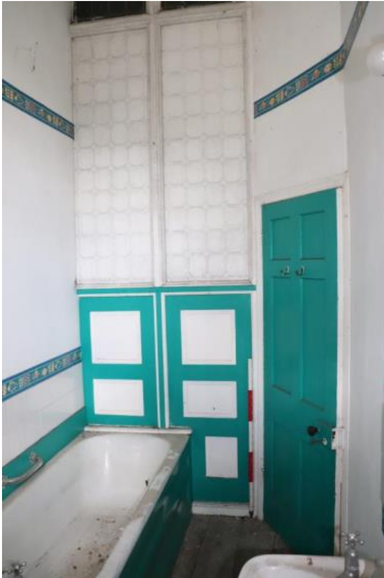
Plate 164 Phase 6 inserted partially glazed screen, room F11b, looking north-east, scale 1m
