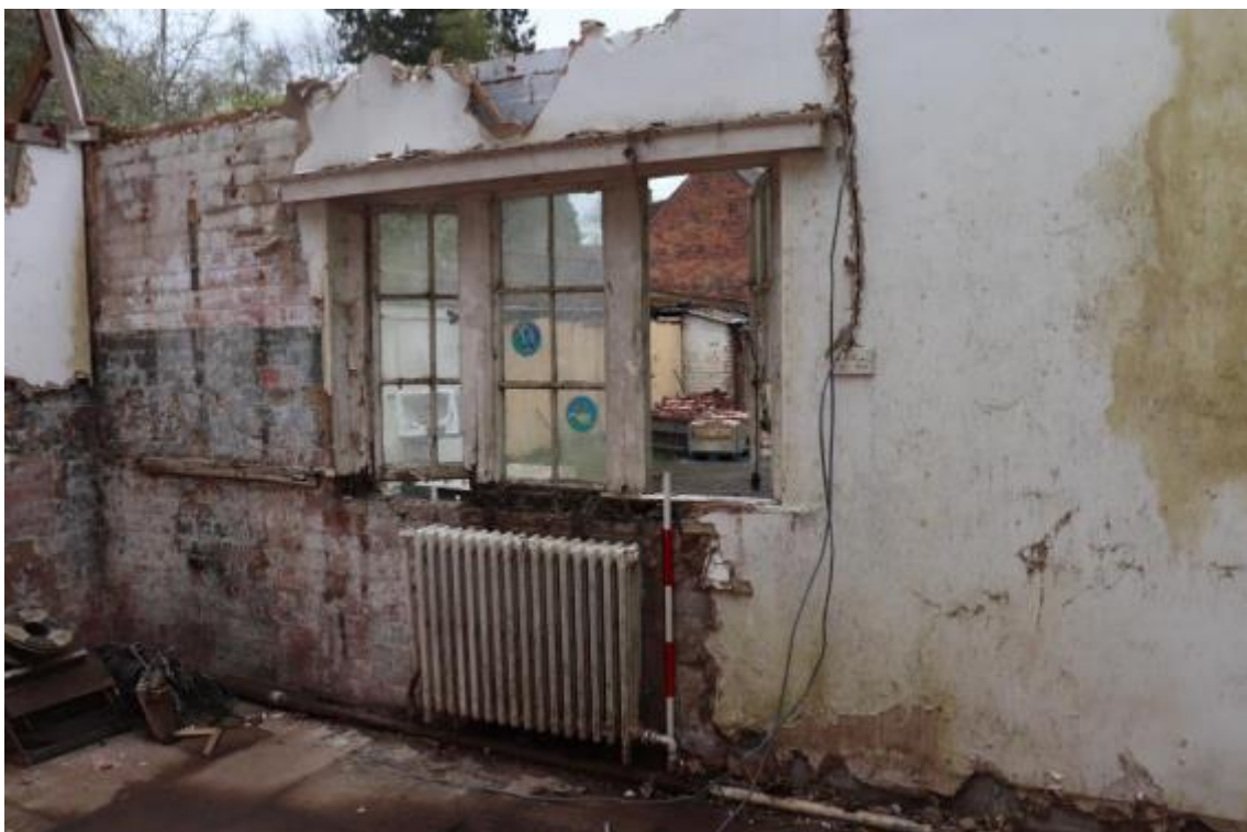
Plate 160 Phase 6 room G27, looking north, scale 1m
