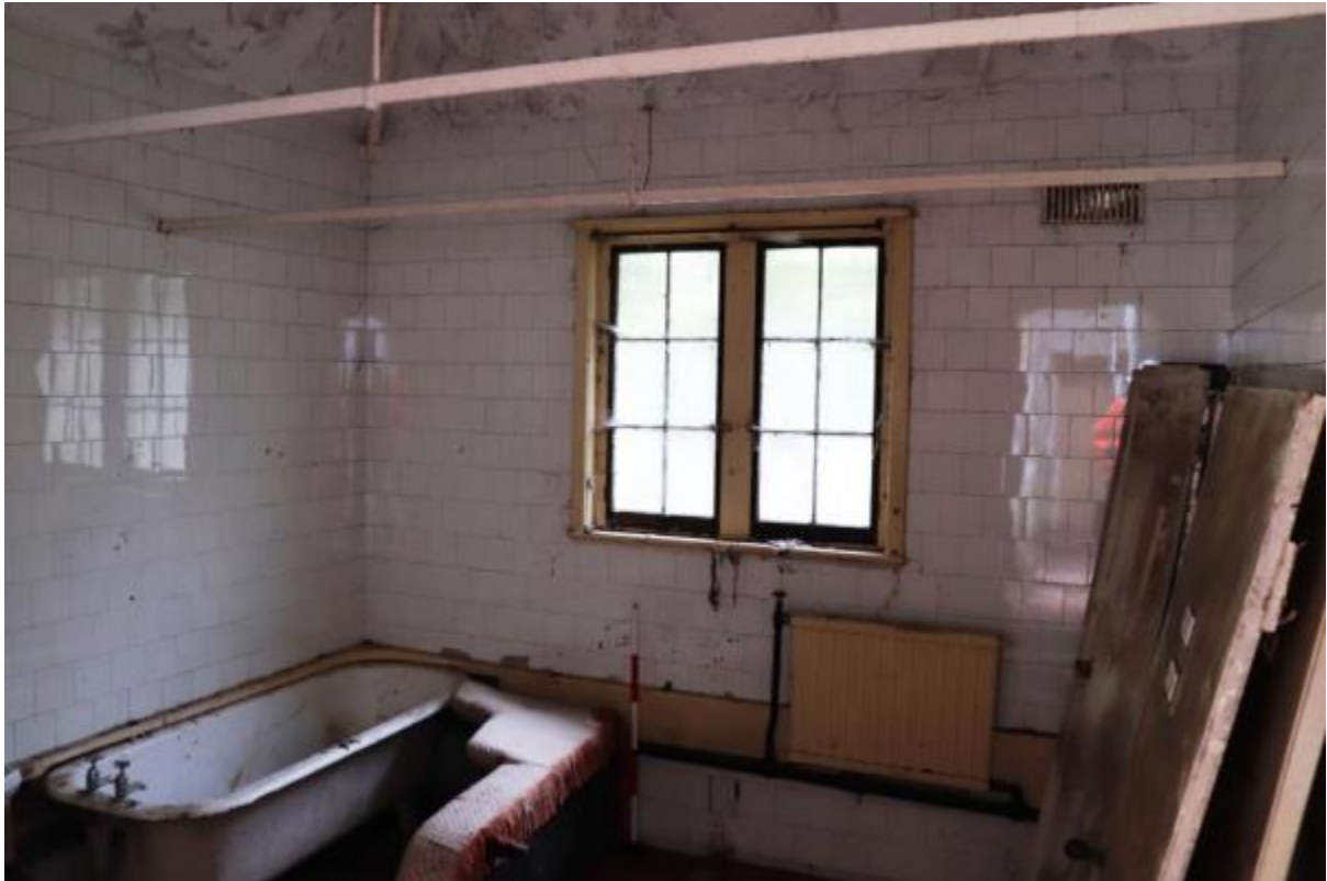
Plate 159 Phase 6 room G28, looking north-west, scale 1m
