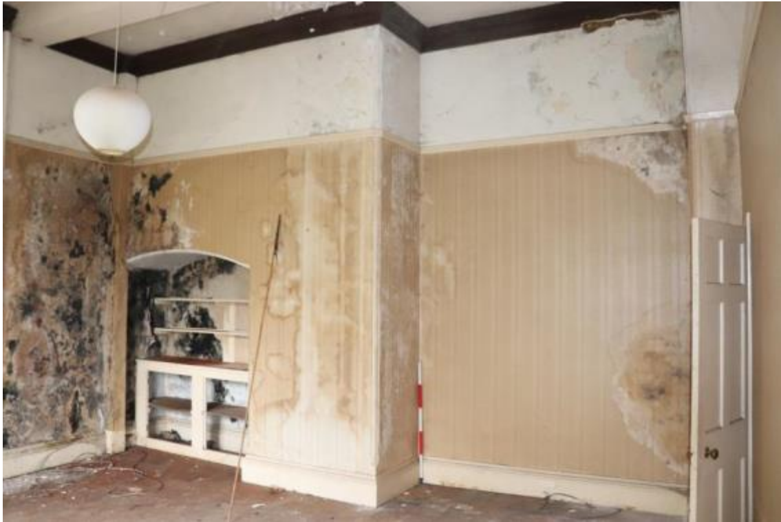
Plate 70 Phase 2 former chimney breast within room F13, looking north, scale 1m
