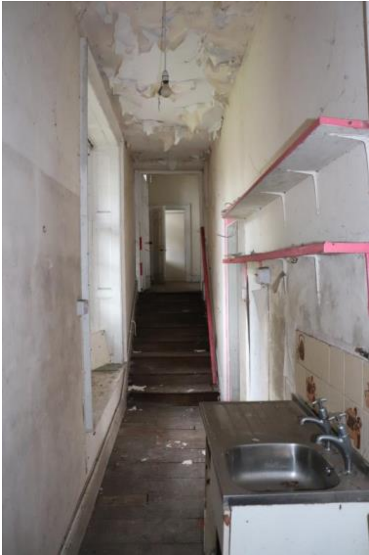
Plate 136 Phase 3 room F8, looking north-west, scale 1m
