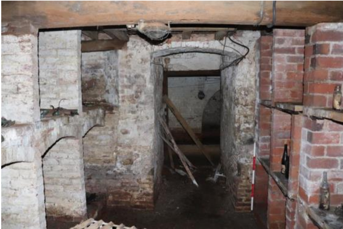
Plate 44 Phase 1 cellar and later inserted doorway, looking north-west, scale 1m
