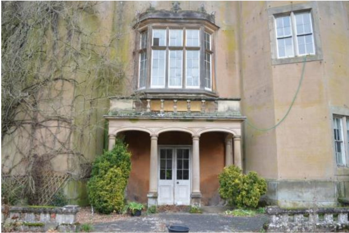
Plate 117 Phase 3 oriole window and Phase 5 porch below, looking north-east, no scale
