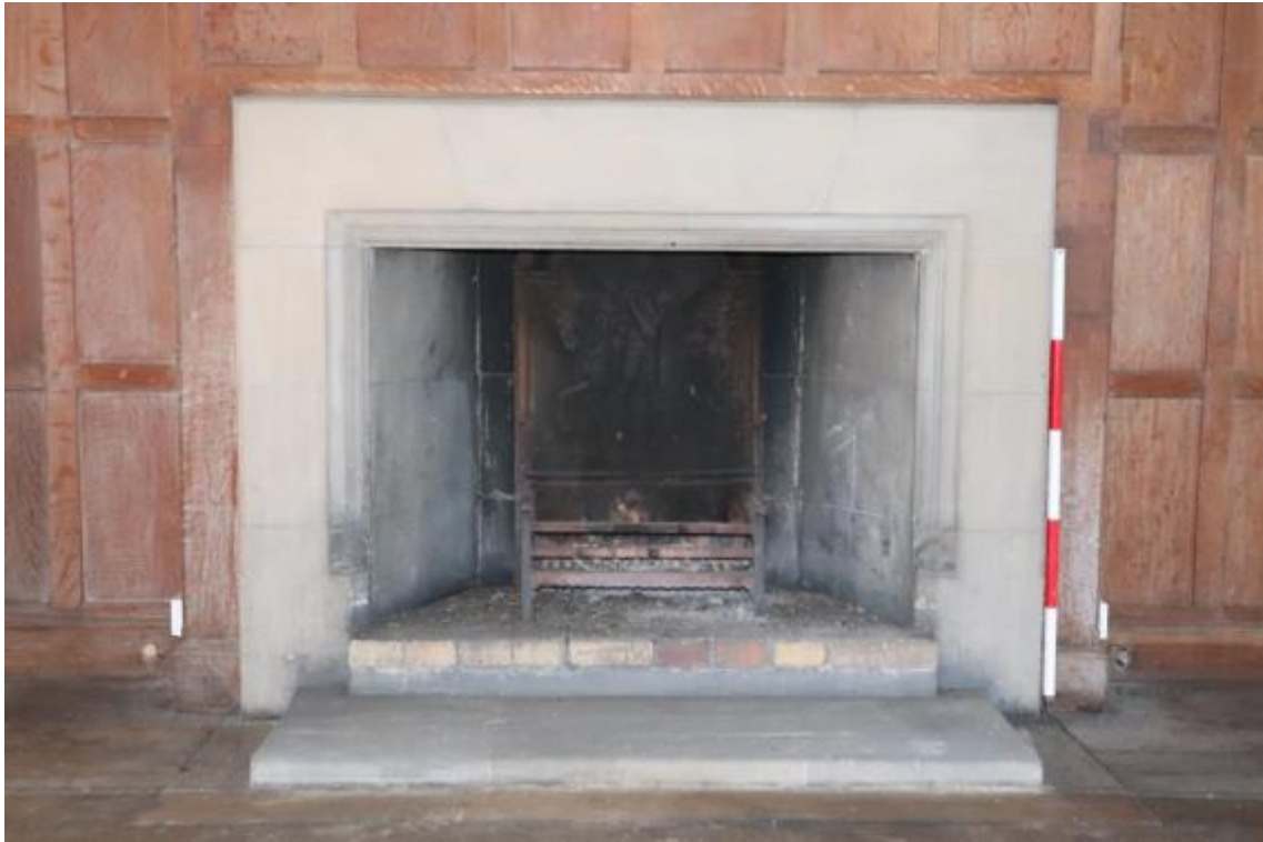
Plate 130 Room G1 inserted fireplace surround, looking north-west, scale 1m
