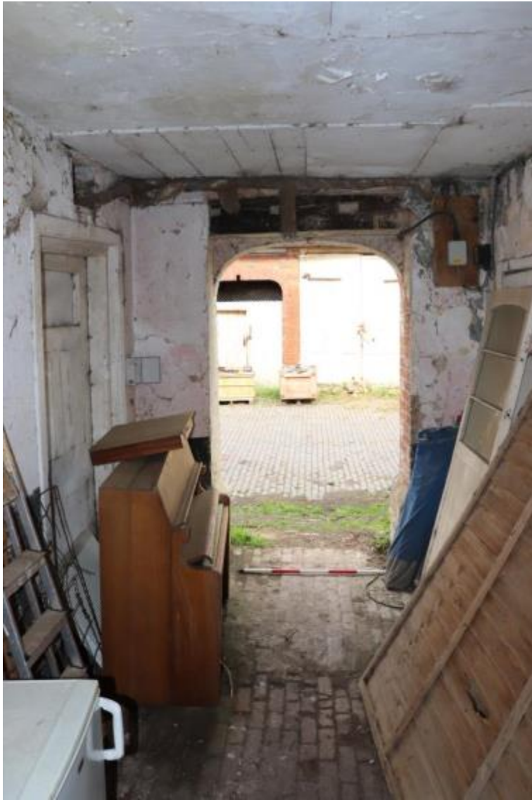
Plate 96 Phase 2 room G21, looking north-west, scale 1m
