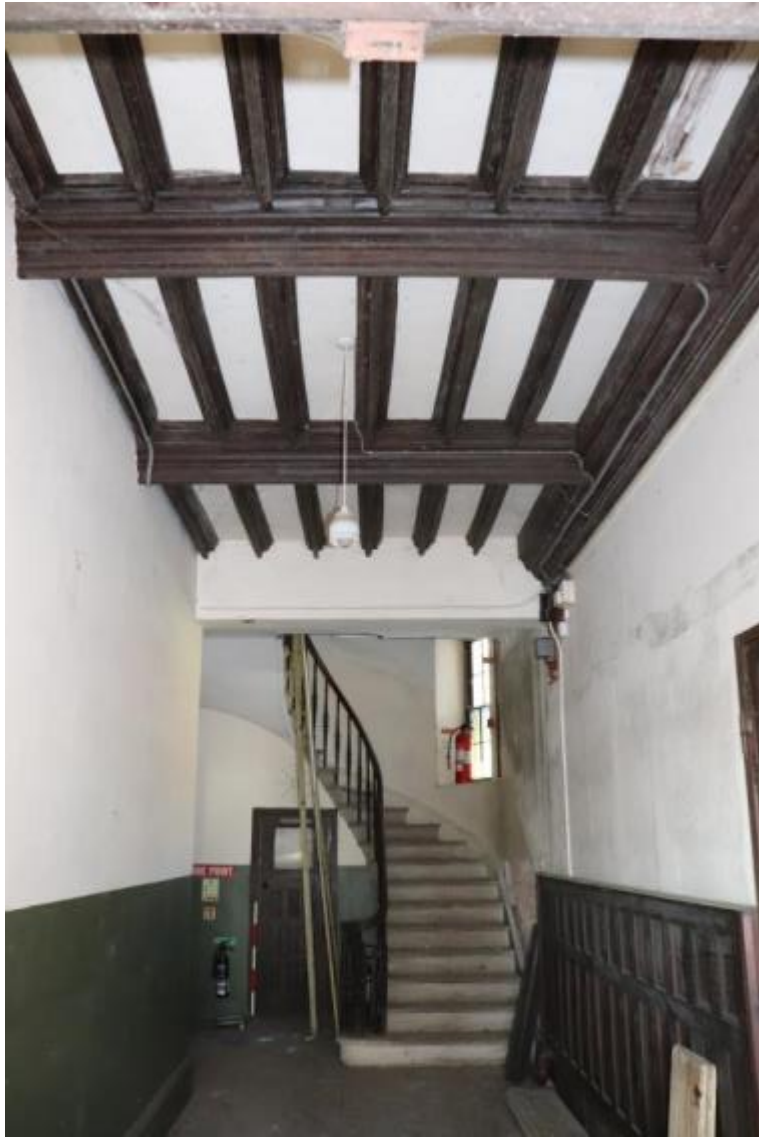
Plate 38 Phase 1 moulded ceiling structures within the house entrance, looking south-west, scale 1m
