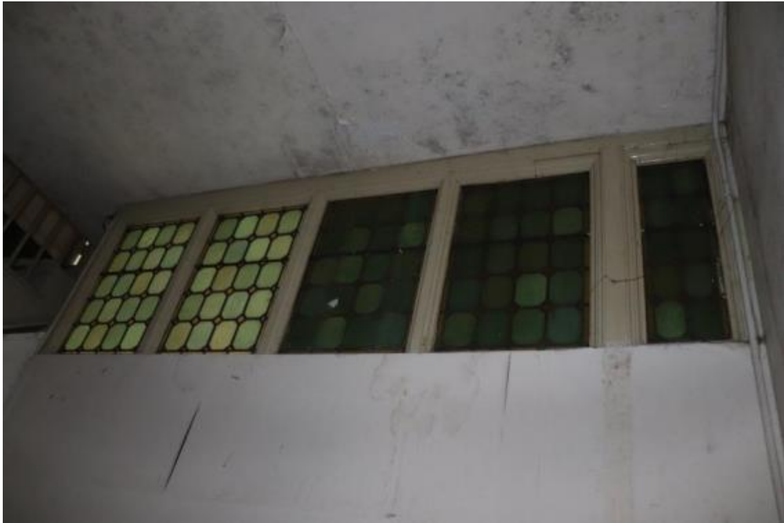
Plate 165 Phase 6 inserted partially glazed screen, room F15a, looking south-west, no scale
