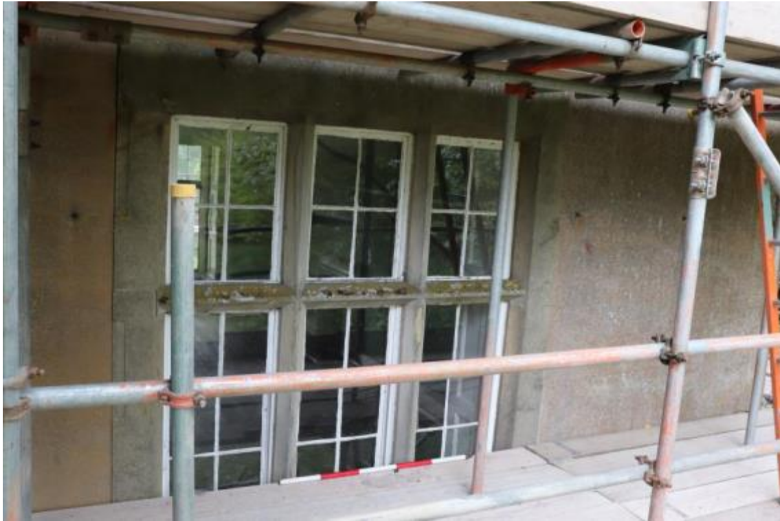
Plate 114 Typical Phase 3 Stone cross windows, looking south-west, scale 1m
