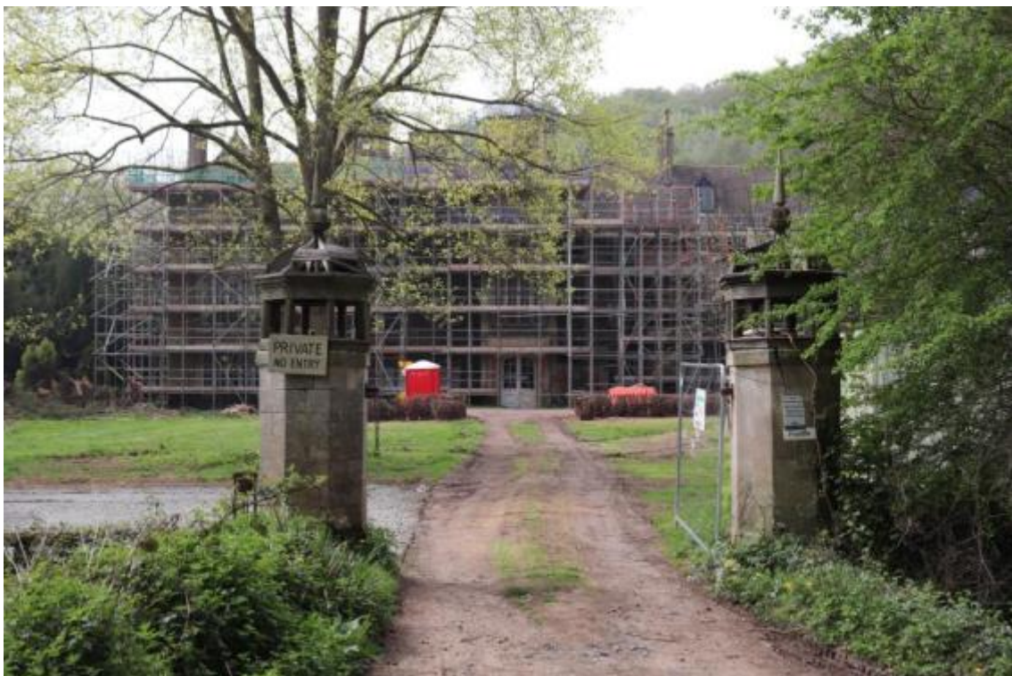
Plate 27 Ribbesford House entrance general appearance, looking south-west, no scale
