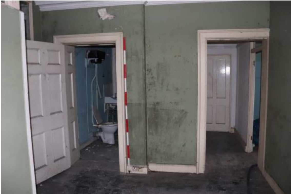
Plate 142 Room S8a, looking north-west, scale 2m
