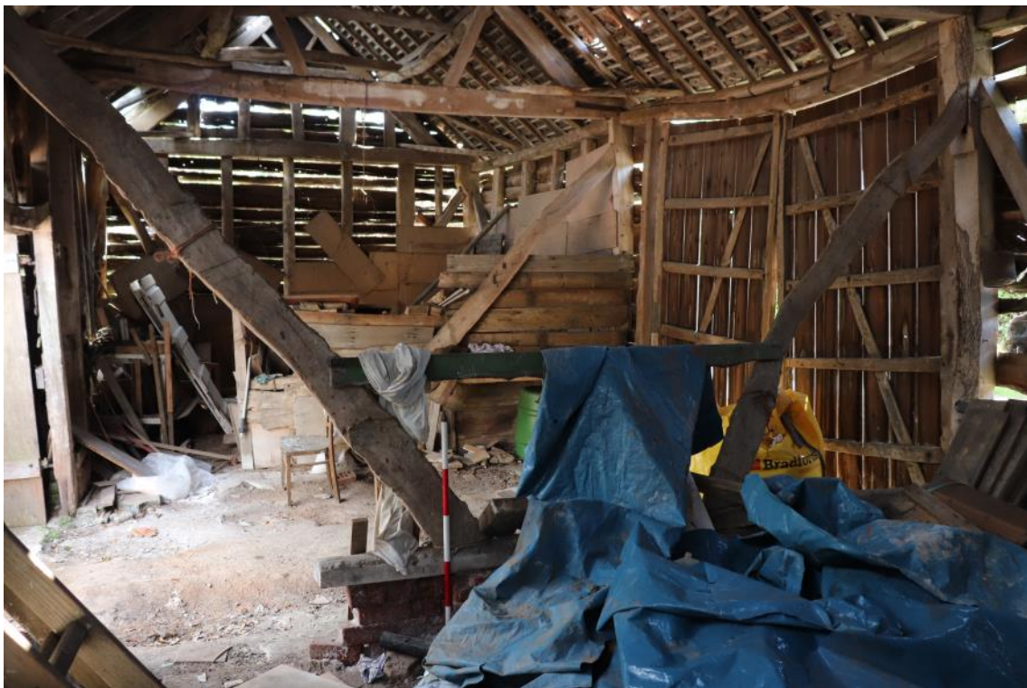
Plate 13 Phase 2, Truss 2, looking south, 1m scale
