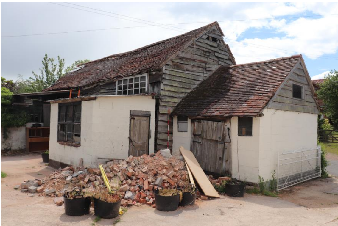
Plate 8 Phase 2 barn exterior with added bay to its north, looking south-west, 2m scale
