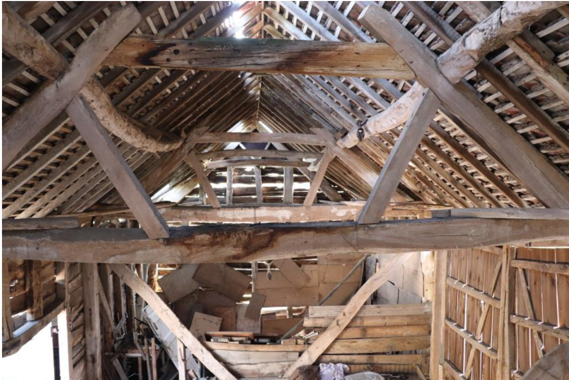
Plate 16 Phase 2 Trusses 2 and 3 above tie beam level, looking south, no scale
