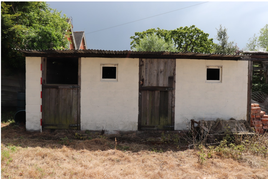
Plate 23 Phase 4 stabling, looking south, 2m scale
