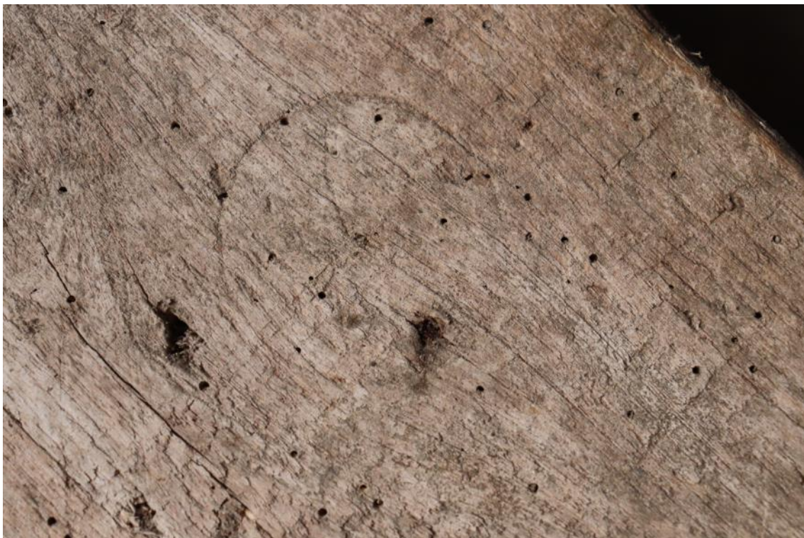
Plate 17 Daisy wheel on Truss 3, looking south, no scale
