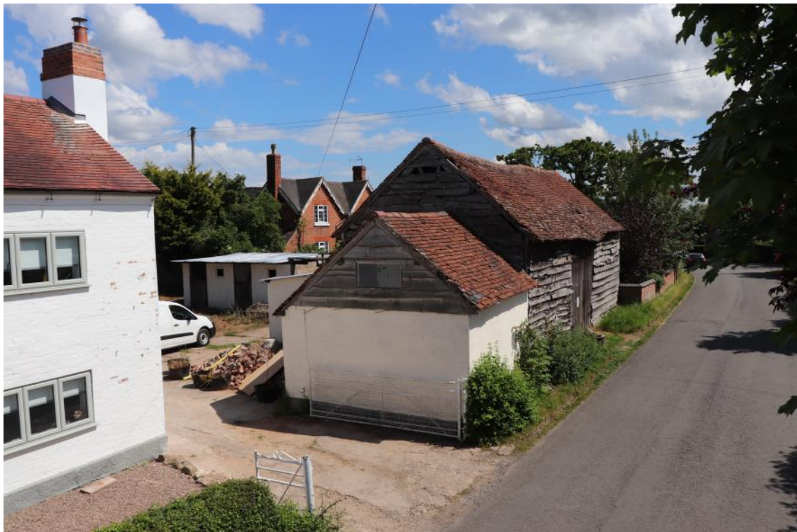
Plate 2 General view of the barn with Hilltop Farmhouse to the left, looking south-east, no scale
