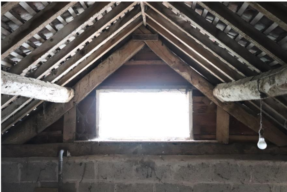
Plate 19 Phase 2 Truss 5, looking north, no scale
