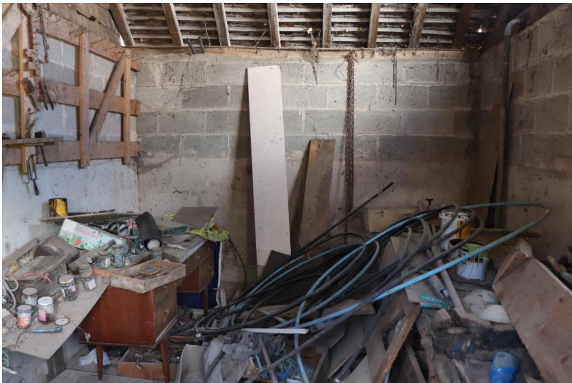
Plate 21 Phase 4 stabling rebuilt from Phase 2 added bay, looking west, no scale
