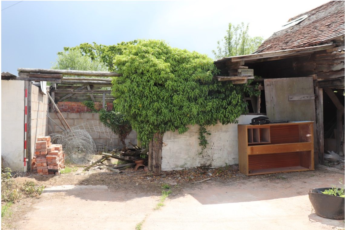
Plate 24 Phase 4 stabling, looking south, 2m scale
