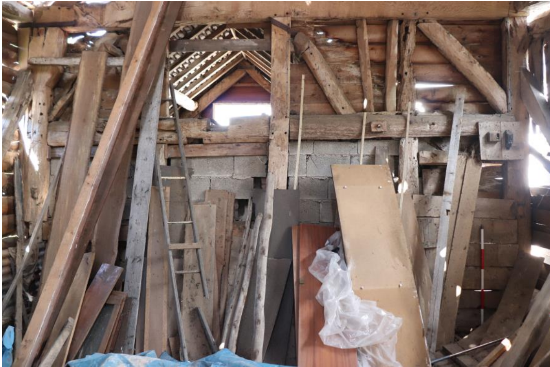
Plate 5 Phase 1 Truss 1, looking north, 1m scale
