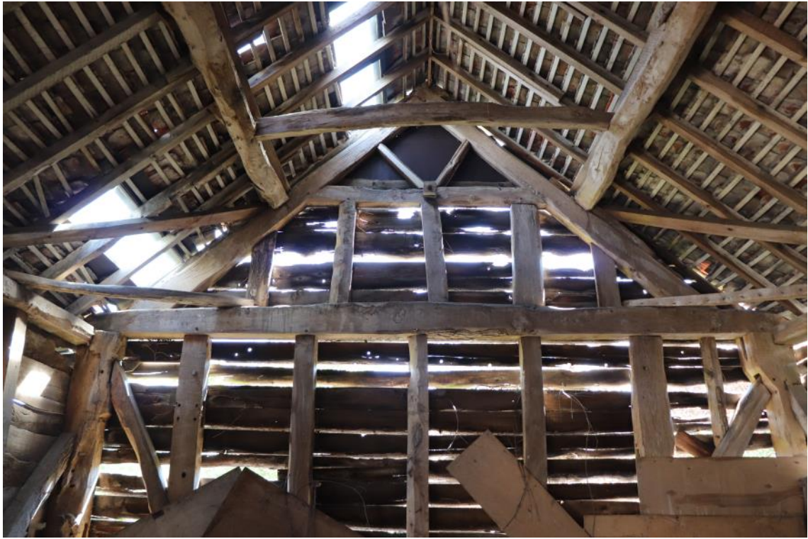
Plate 14 Phase 2, Truss 4, looking south, no scale
