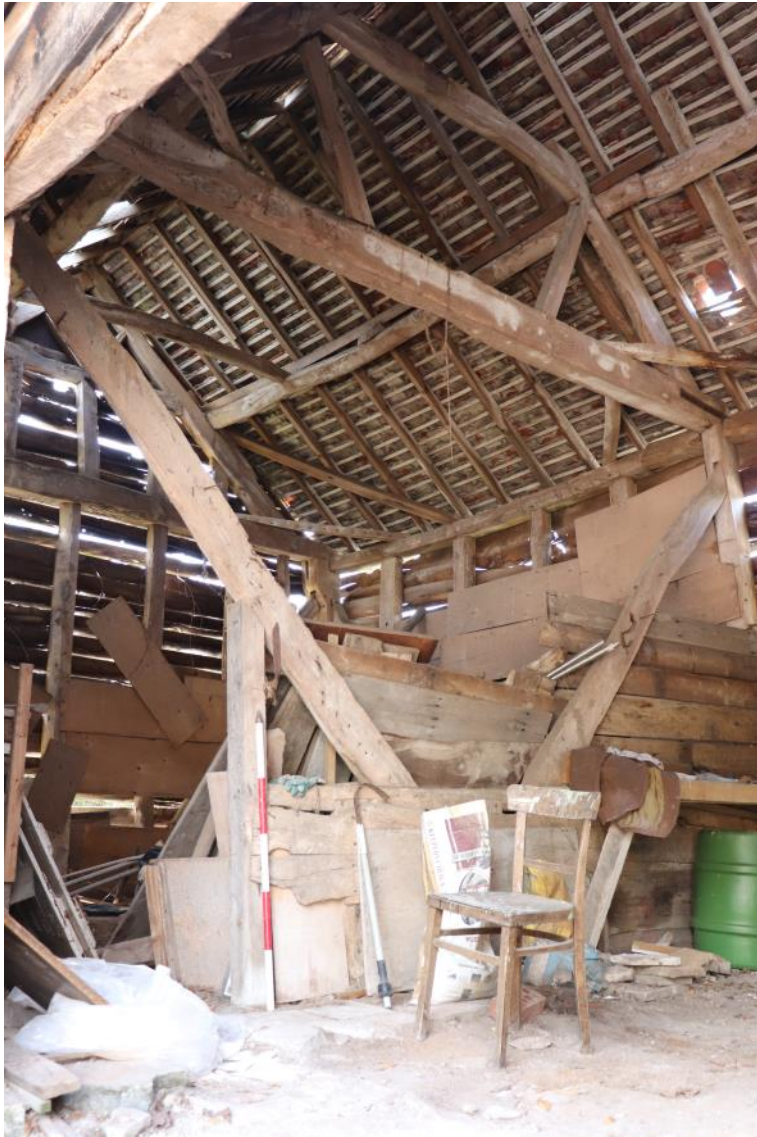
Plate 15 Phase 2, Truss 3, looking south-west, 1m scale
