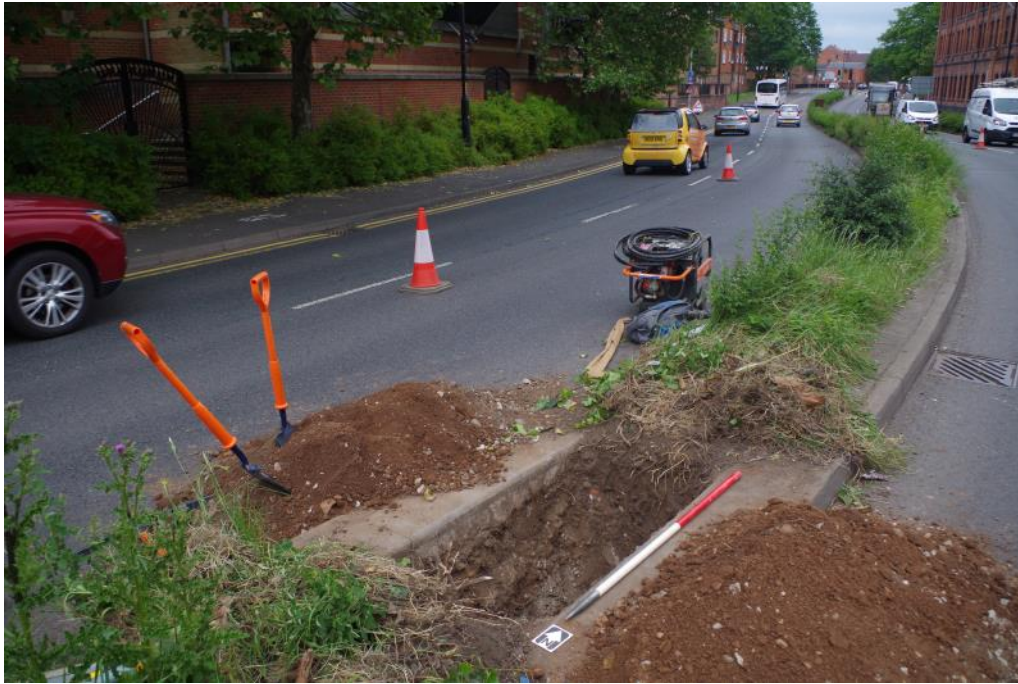
Plate 3: Trench 2 looking north-west, scale 1m
