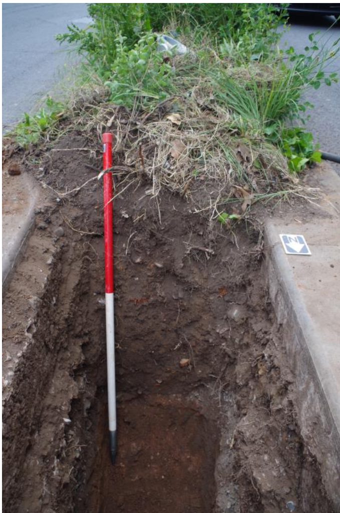
Plate 4: Trench 2 looking south, scale 1m
