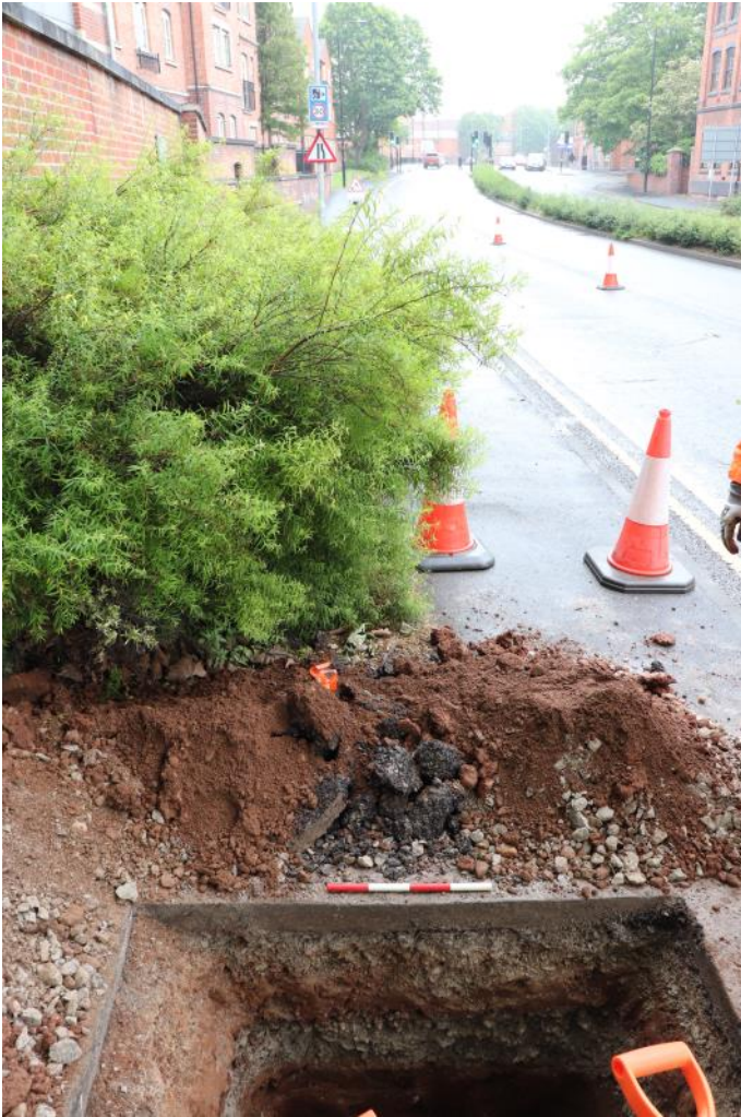
Plate 1: Trench 1 looking north, scale 0.5m
