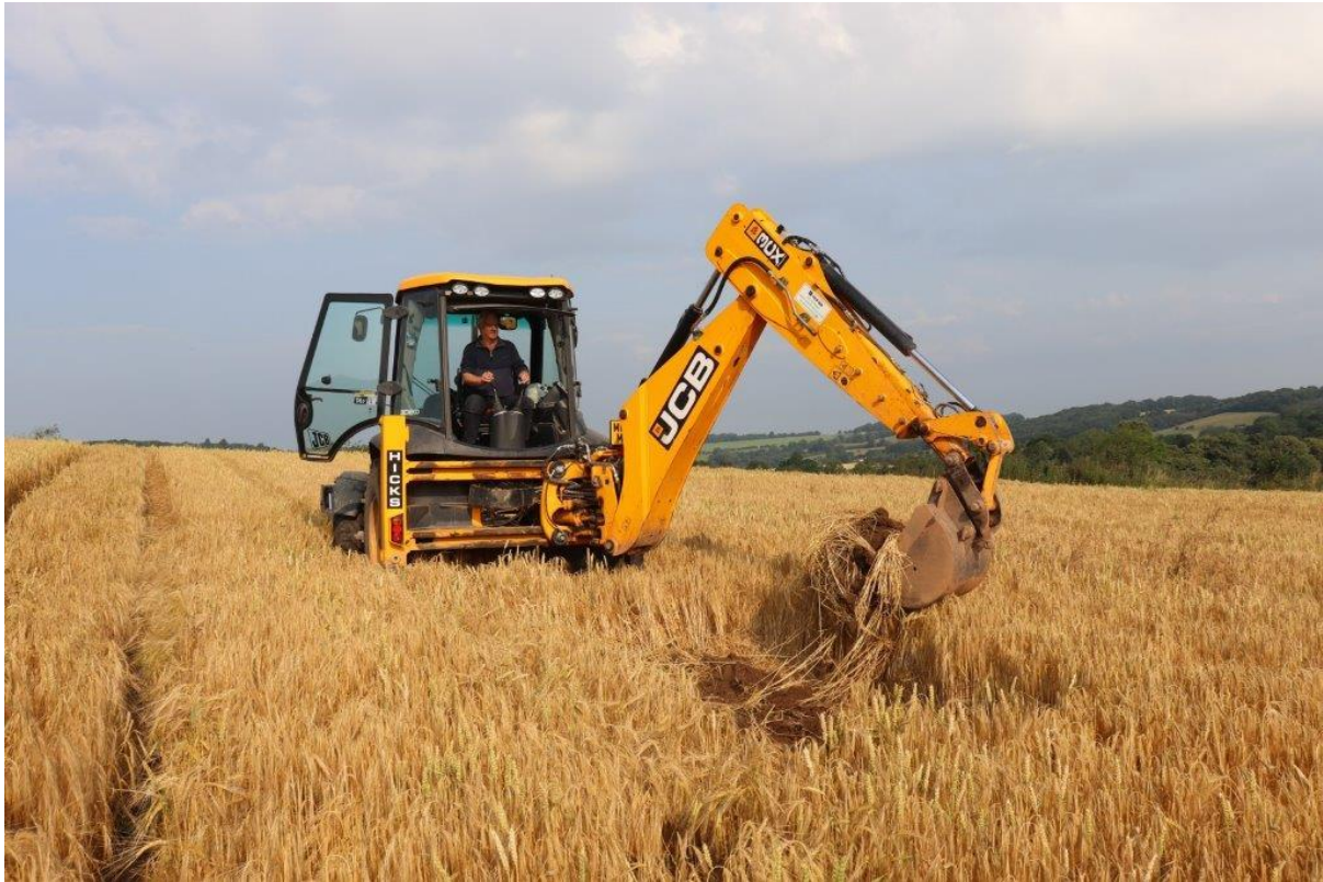
Plate 1: Opening Trial Hole in arable wheat field. View northwest.
