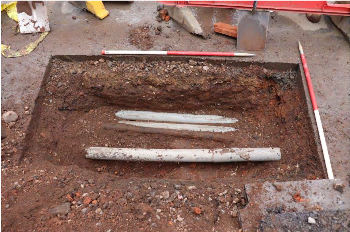
Plate 13: Trial Pit 10 showing modern services and backfill, view north, 2x 1m scales
