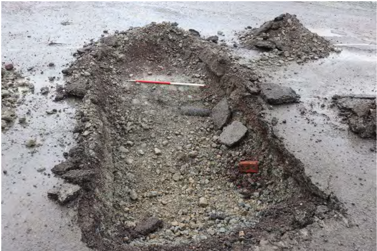
Plate 12: Trench 5, aborted due to presence of live service ducting, 1m scale
