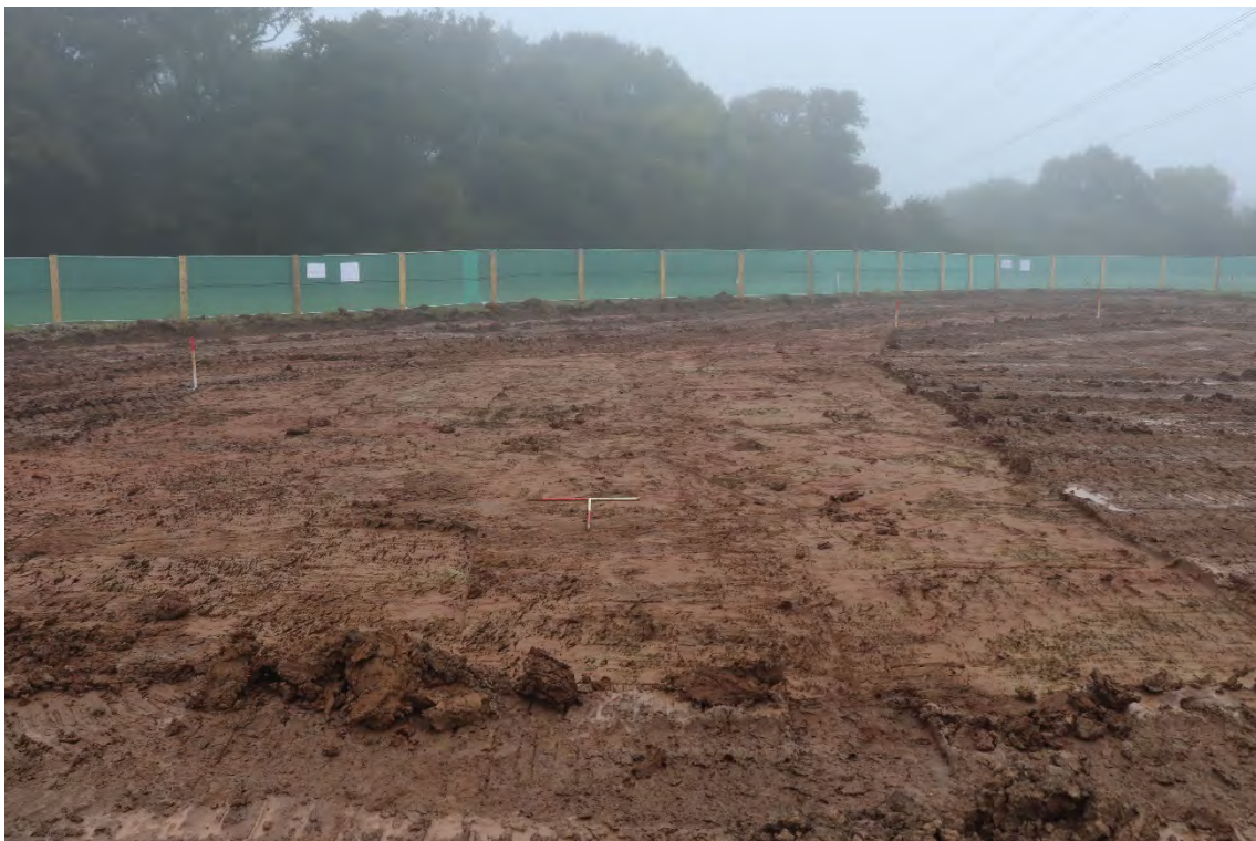
Plate 8 Tr 26, looking north-east, 2x1m scales
