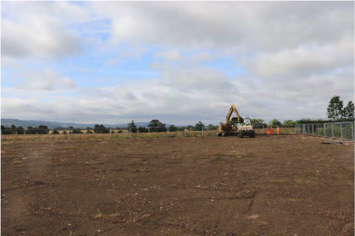
Plate 1: Trench 1 with vegetation stripped, prior to excavations, view south-west, no scales
