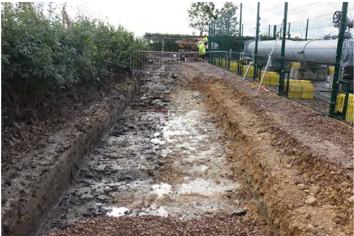
Plate 10: Trench 4 perimeter fence, view south-west, 1m scales
