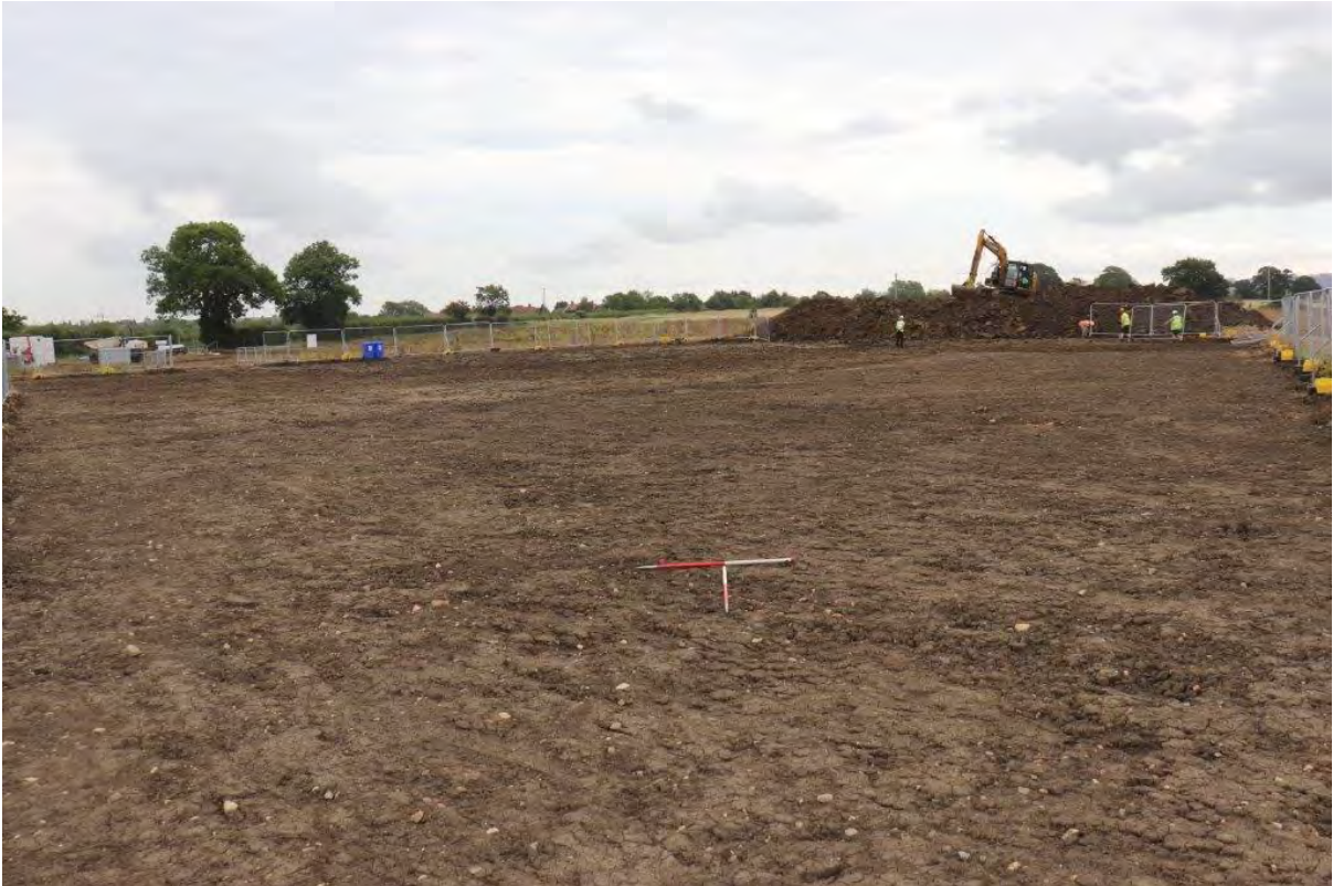
Plate 2: Trench 1 following topsoil strip, view south-east, 1m scales
