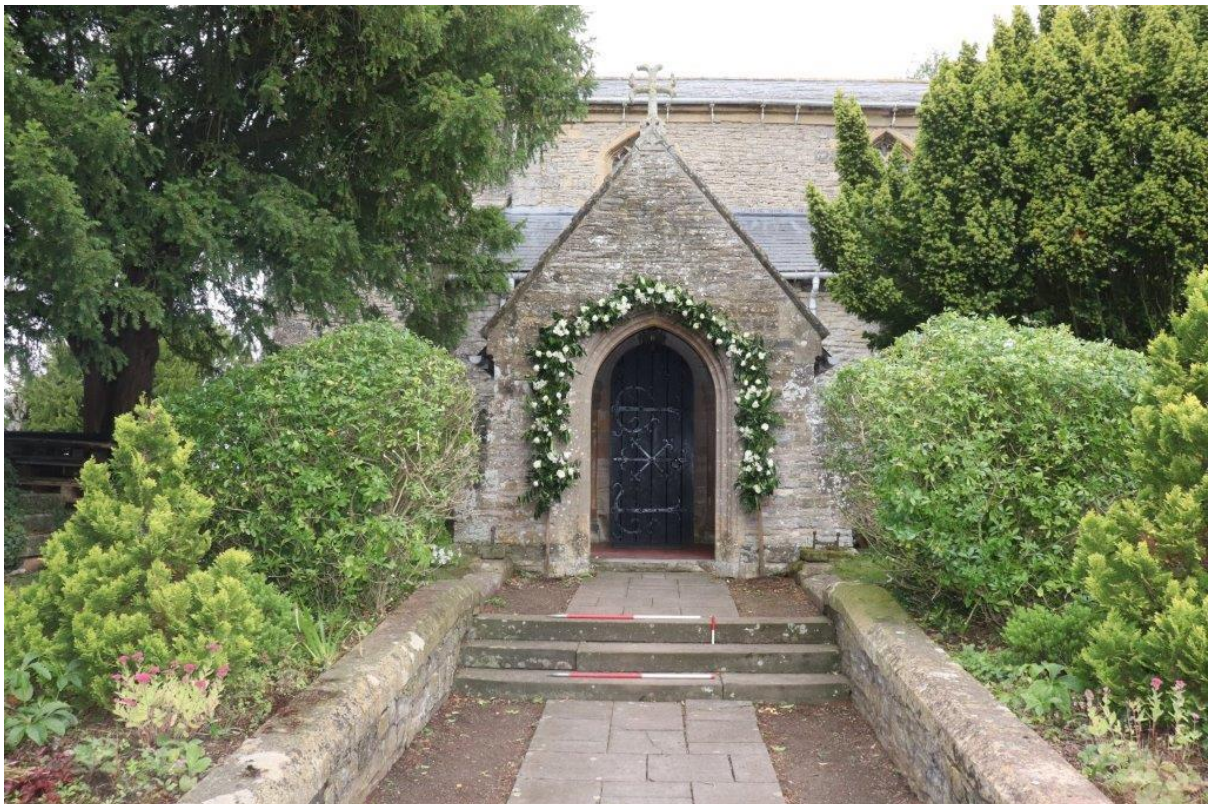
Plate 4: Church entrance and porch. 1m scales and 0.2m, view north
