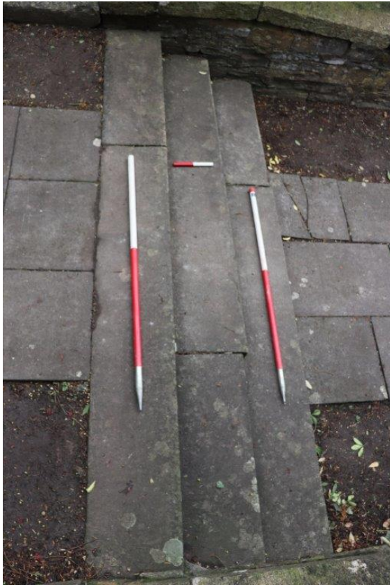
Plate 9: York stone steps and concrete paving slabs, view east from above. 2 x 1m scales and 0.2m. View west
