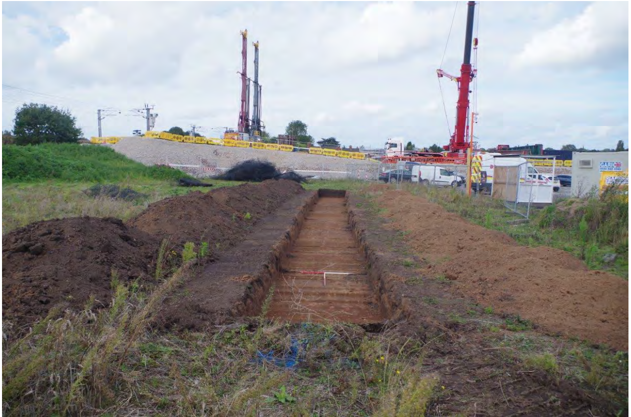
Plate 5: Trench 23, looking north (1m scales)
