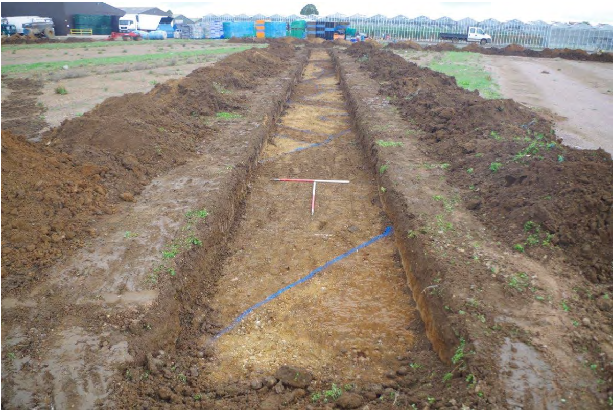
Plate 1 Trench 3 looking north (1m scales)
