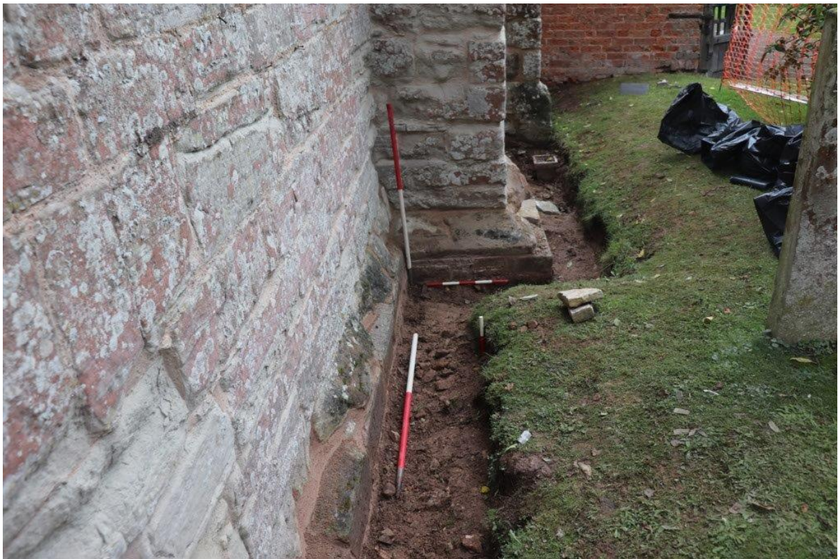
Plate 10: Trench along southern wall of church, looking East towards the porch. 1m and 0.5m scales visible
