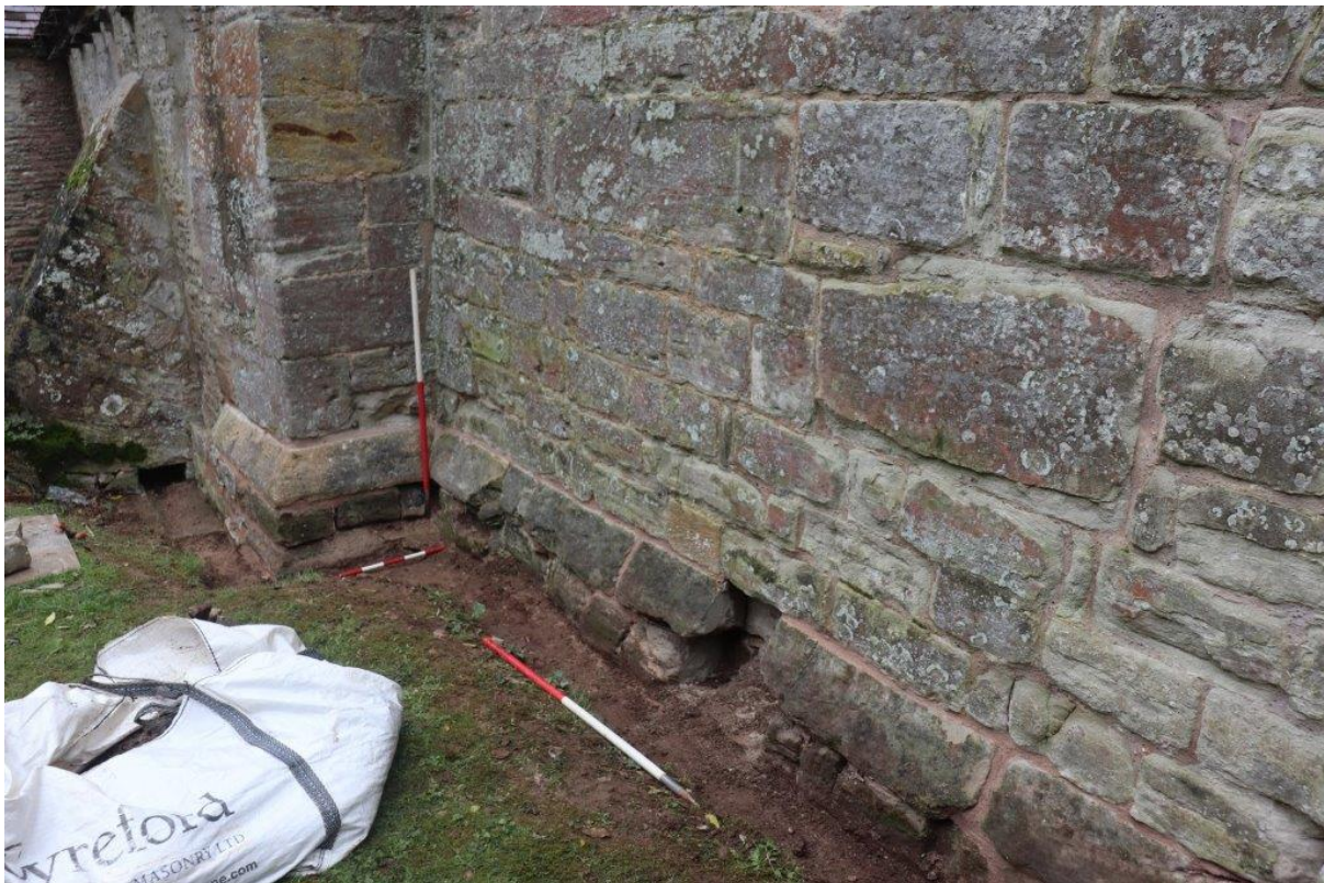
Plate 6: Northwest corner of church. 1m and 0.5m scales. Looking southeast
