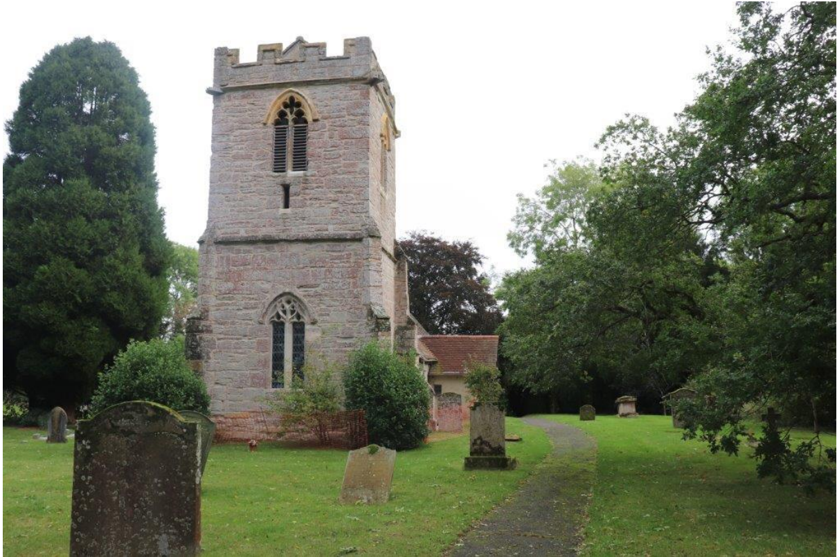
Plate 7: The church bell tower and porch looking East
