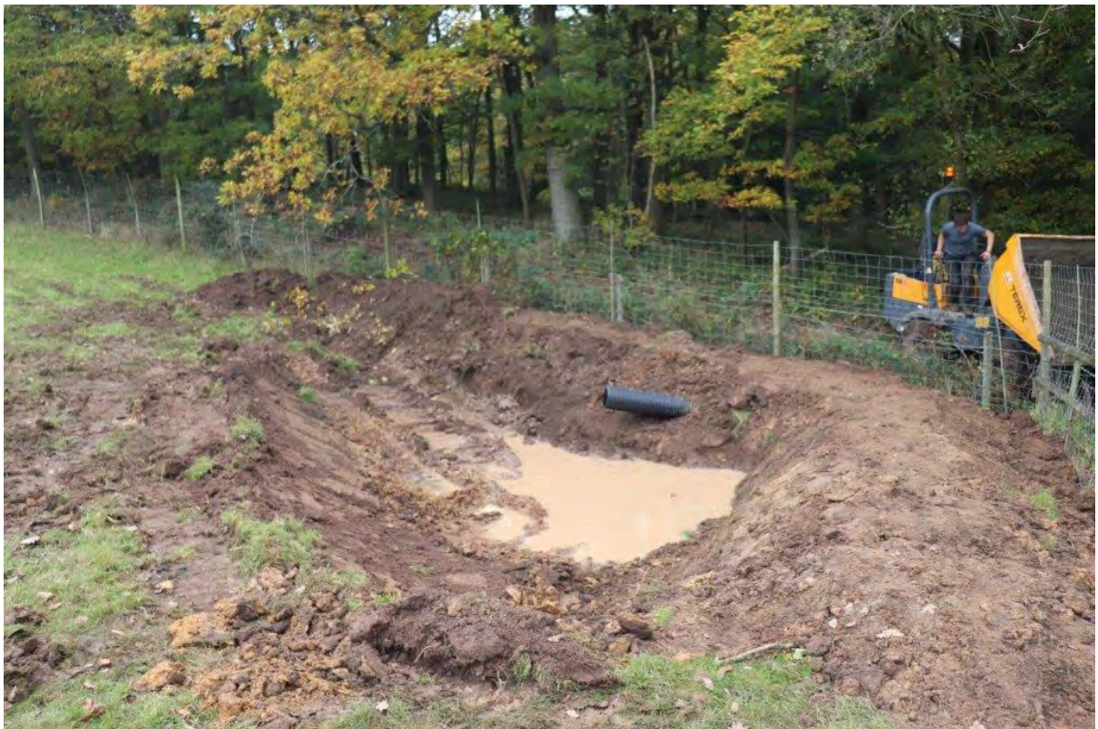
Plate 4: Pond as fully excavated, with graded edges and sealed spoil bunds, view west, no scale
