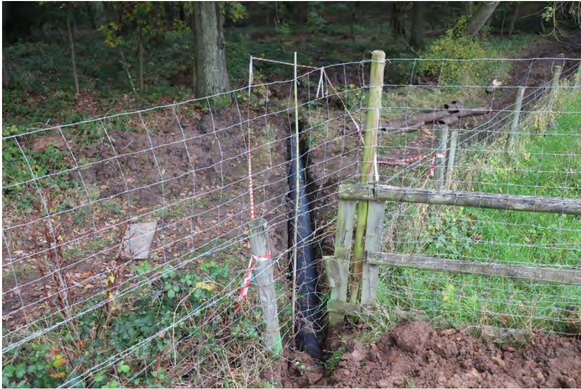
Plate 5: Replaced land drain across forestry track, view north-west from pond excavation bund, no scale
