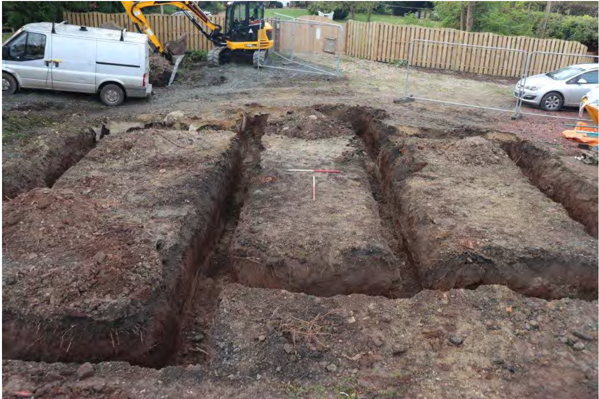
Plate 3: House footings following excavation (Trench 1), view south, 2x 1m scales
