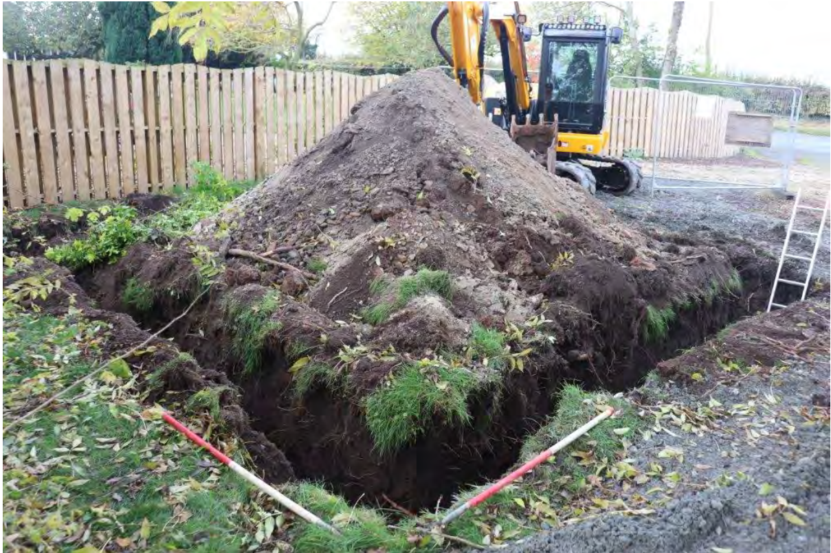
Plate 5: Garage foundations following excavation (Trench 2), view south-west, 1m scales
