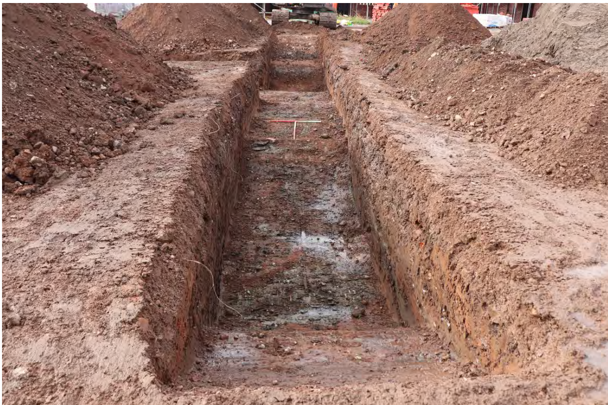
Plate 2 Trench looking west, 2x 1m scales
