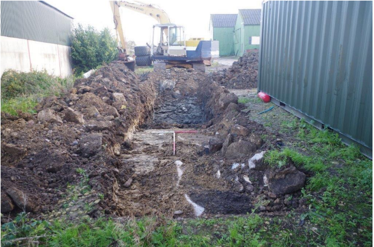
Plate 1: Trench 1, looking east (1m scales)
