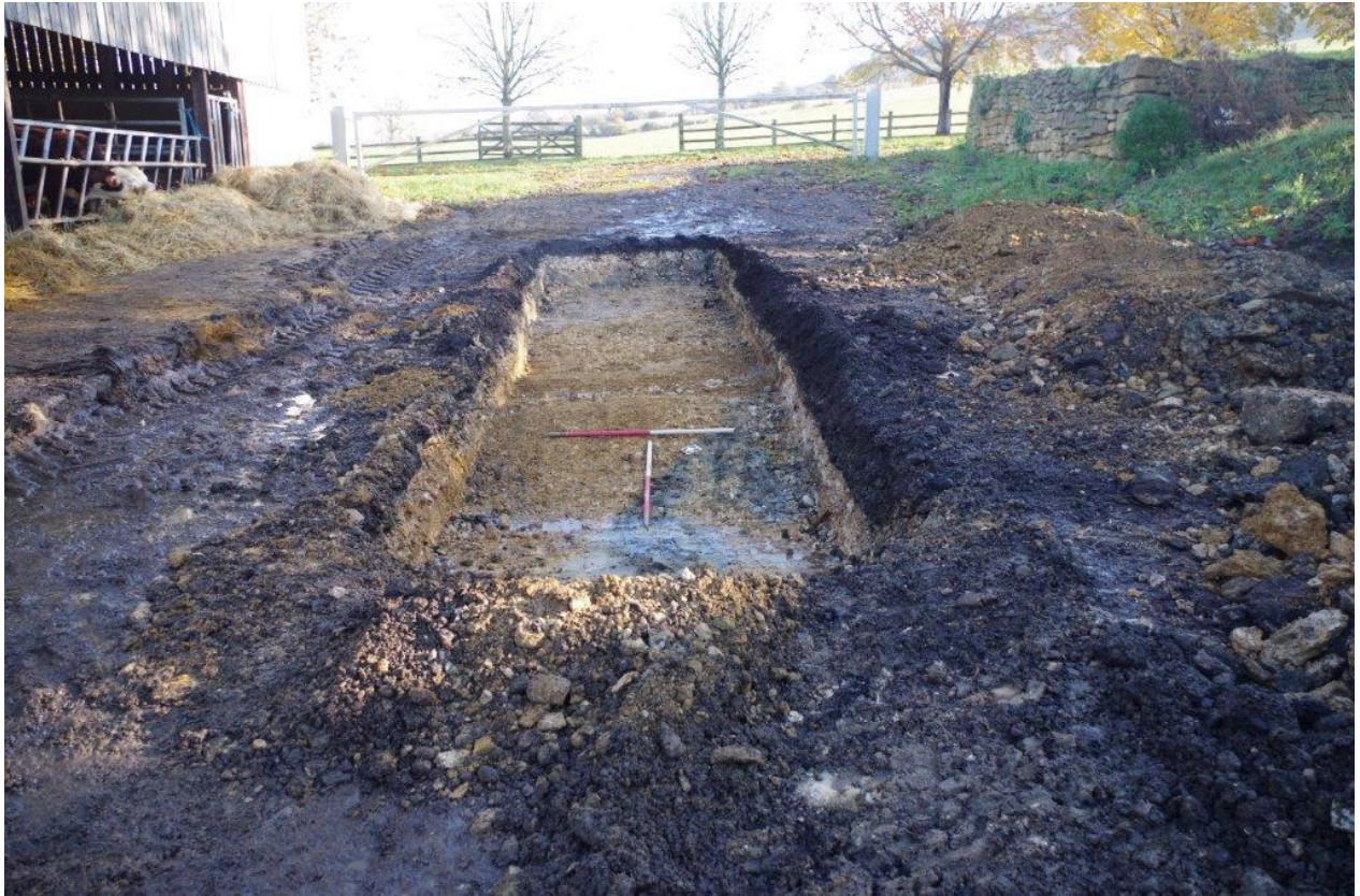
Plate 3: Trench 2, looking east (1m scales)
