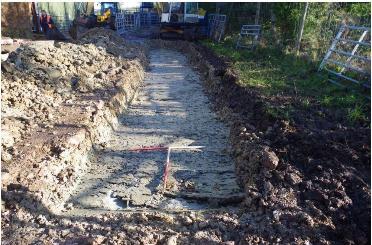
Plate 4: Trench 3, looking east (1m scales)
