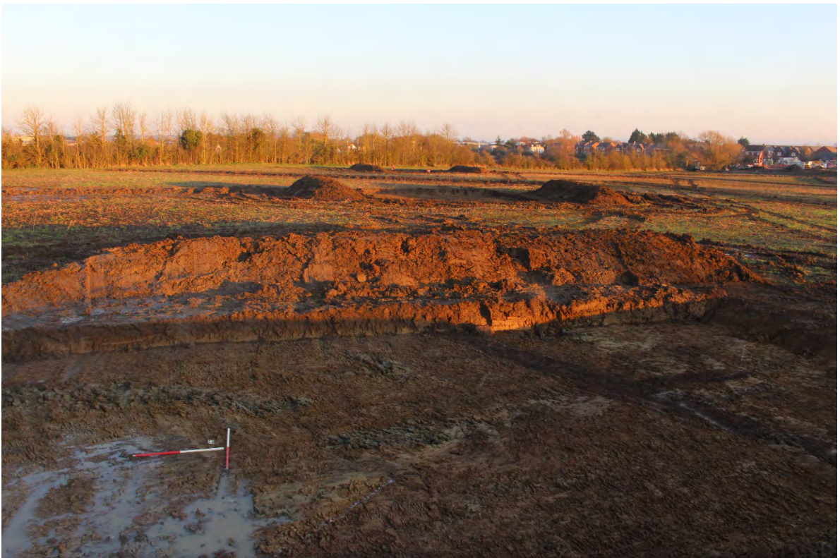
Plate 2: Excavation areas open, general view facing east, 2x 1m scales
