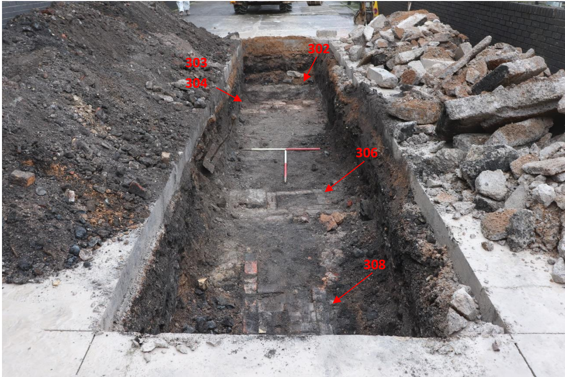
Plate 5: Trench 3 looking north-west, showing some of the identified features
