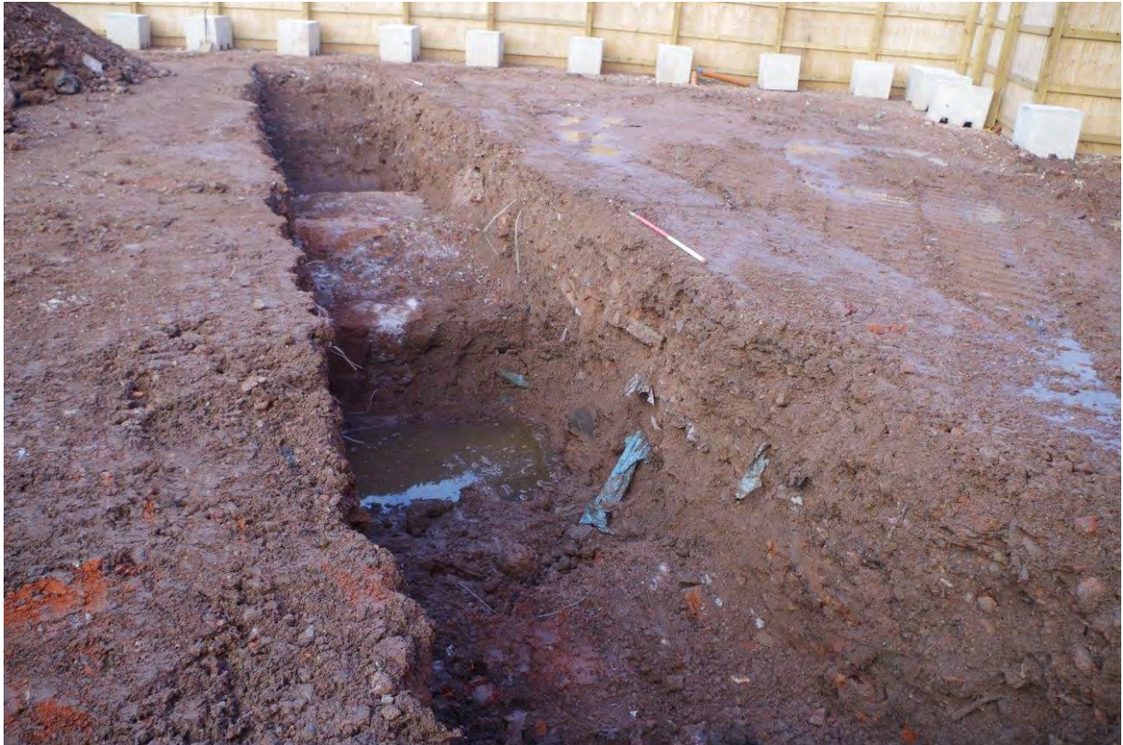
Plate 1: Sondage in Trench 1 showing demolition material; 1m scale, view north
