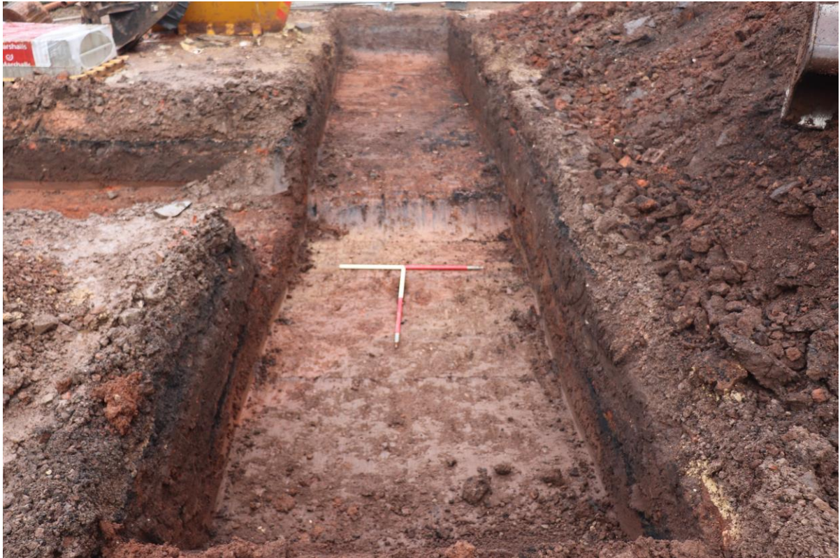
Plate 1: Trench 1 facing north, showing soil (105) in foreground and cut [103] in distance, 2 x 1m scales
