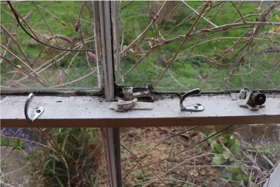
Plate 10 The house ground floor south-west room original and inserted sash fittings
