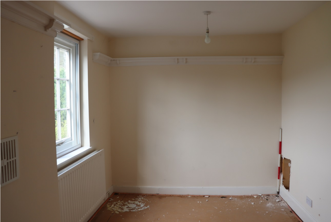
Plate 27 The house first floor, north-west room, looking north, scale 1m
