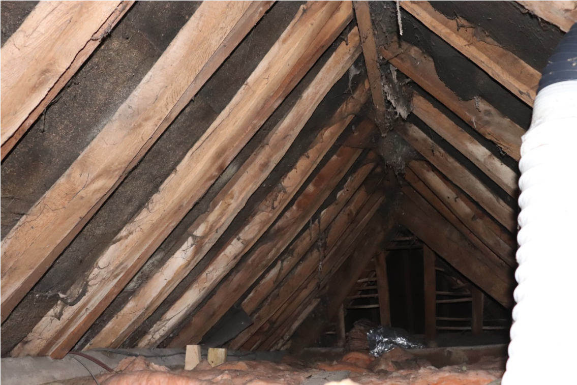
Plate 32 The house second floor, roof structure
