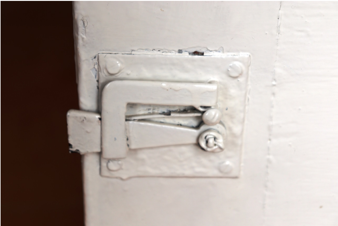
Plate 23 The house first floor with original thin 2 panel door and rear latch, south-east room
