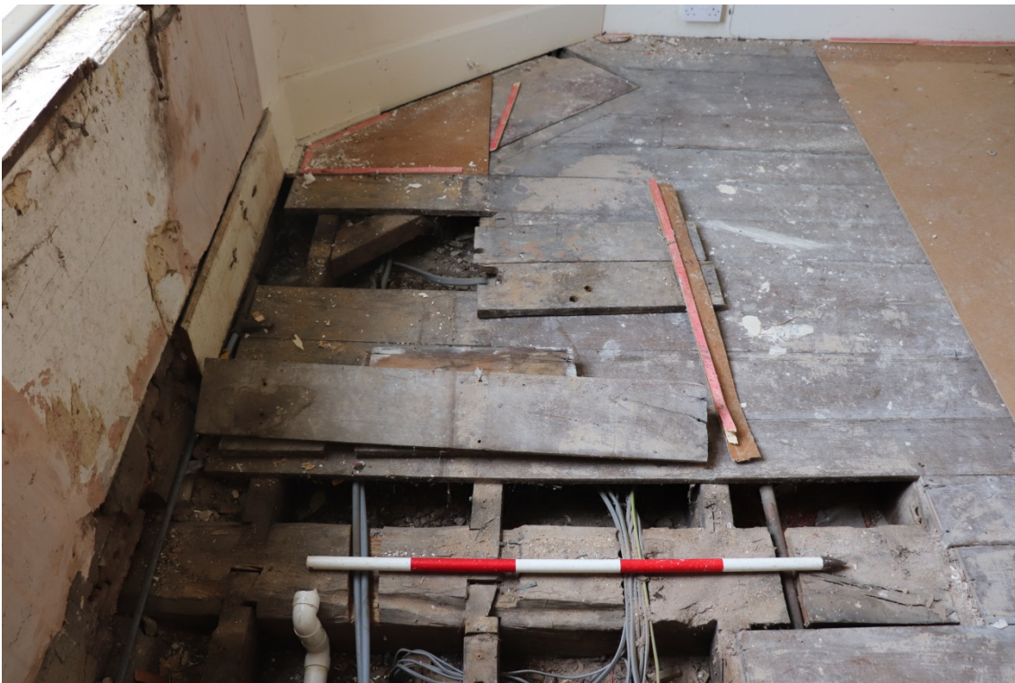
Plate 26 The house first floor joists, north-east room, looking south, scale 1m
