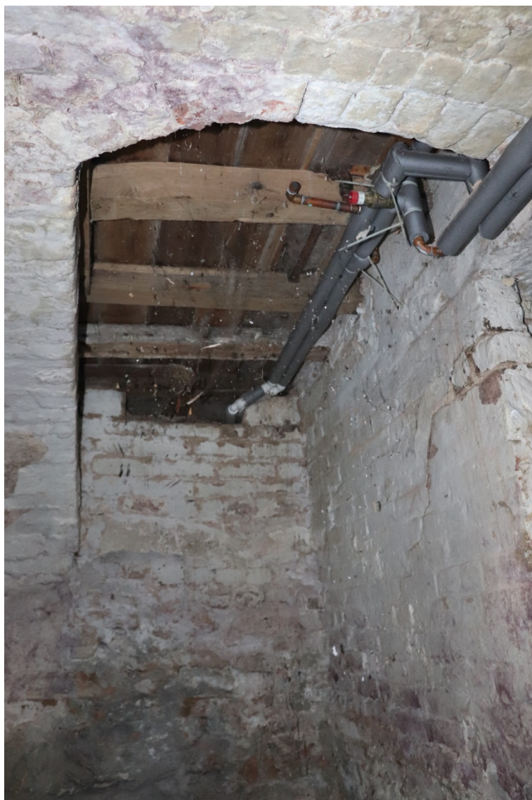
Plate 20 The house cellar former stairs position, looking south, scale 1m
