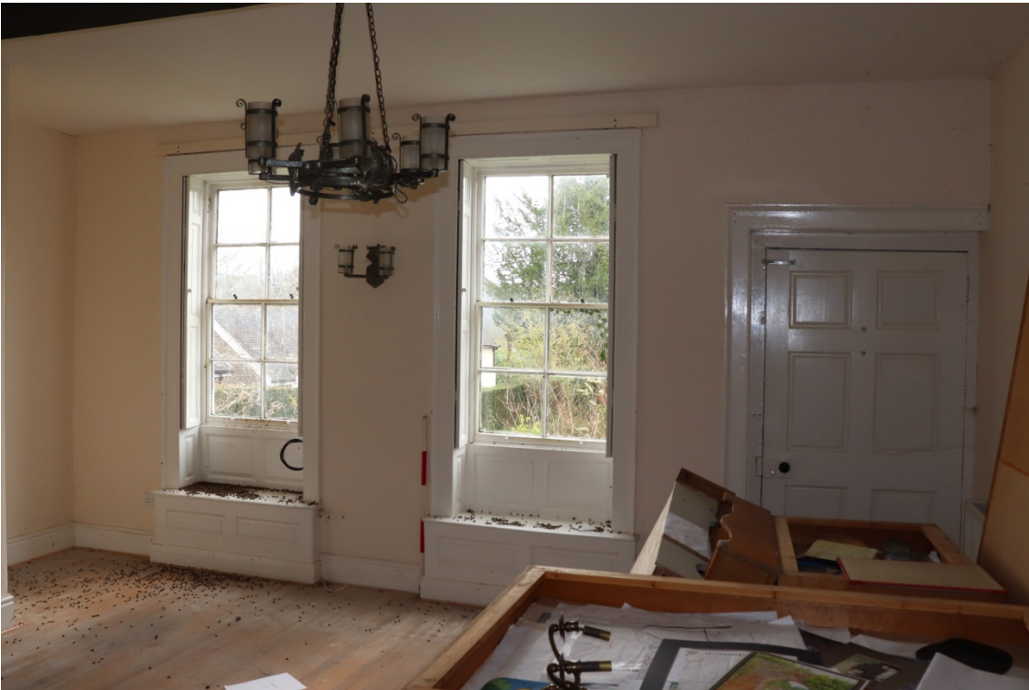
Plate 7 The house ground floor south-east room, looking south, scale 1m
