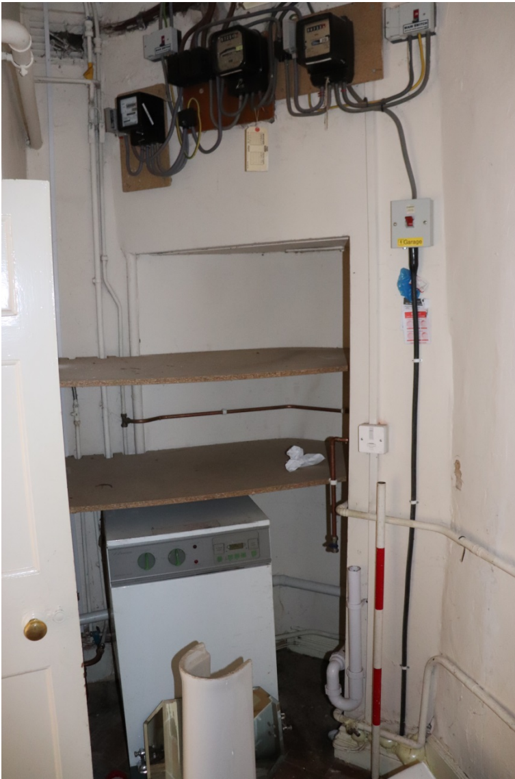
Plate 13 The house ground floor north-east room , looking south-east, scale 1m
