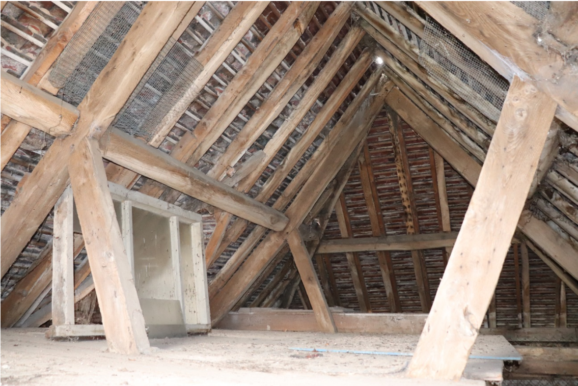
Plate 37 The garage, looking west
