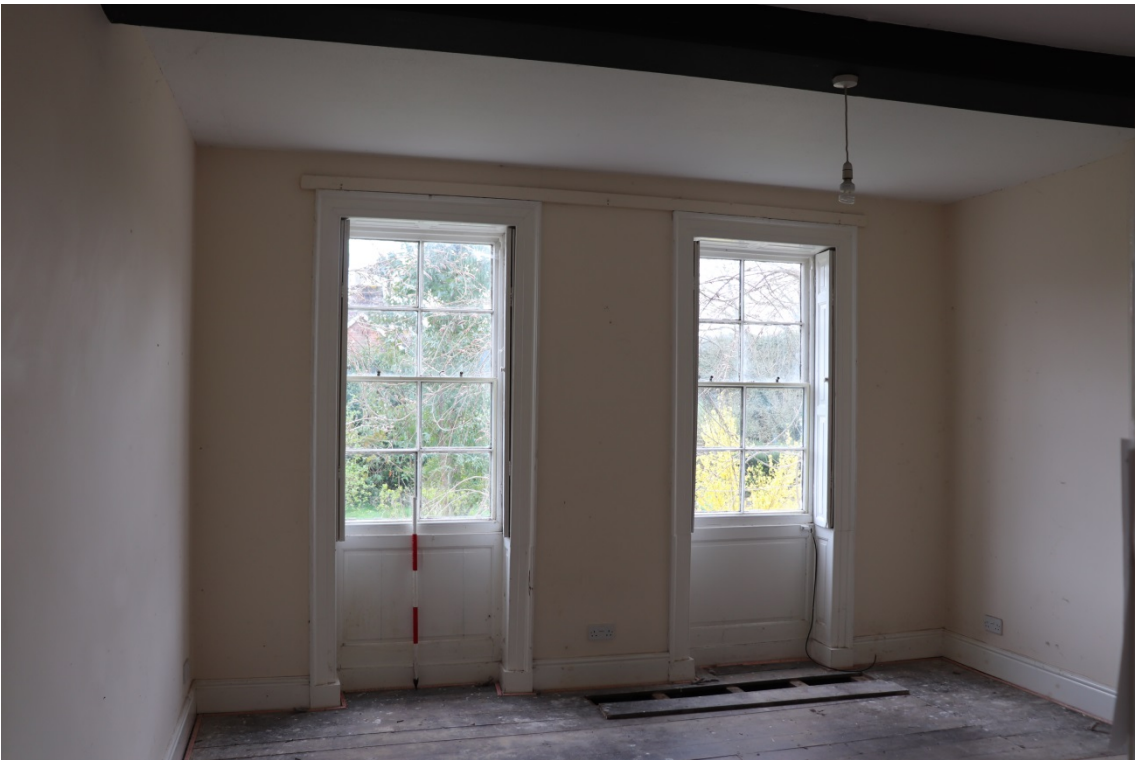
Plate 9 The house ground floor south-west room , looking south, scale 1m
