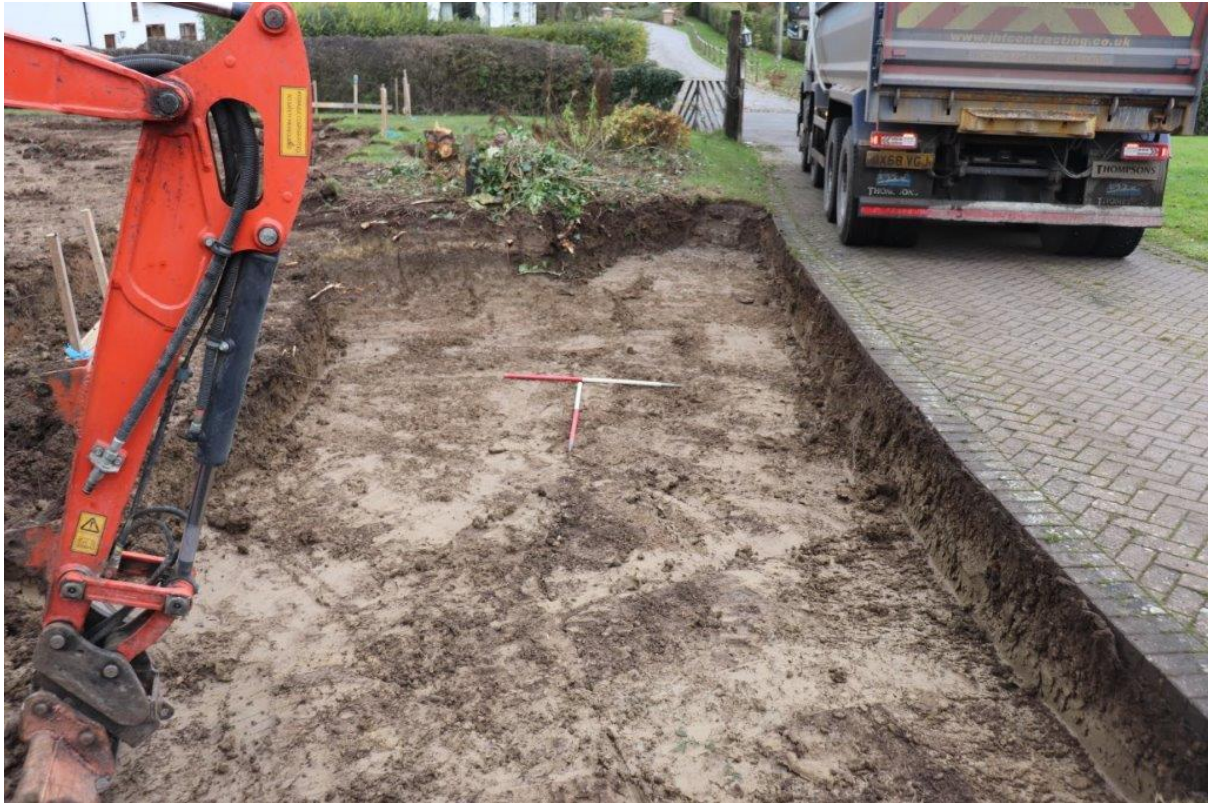
Plate 7: Access area to Trench 1, looking north with 1m scales.
