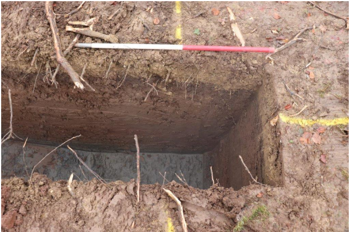
Plate 4: Example of sample section of footings trench. Looking west with 1m scale
