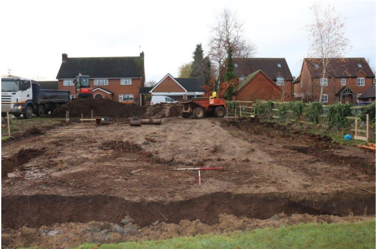
Plate 5: House footings, looking south towards existing house and garage.
