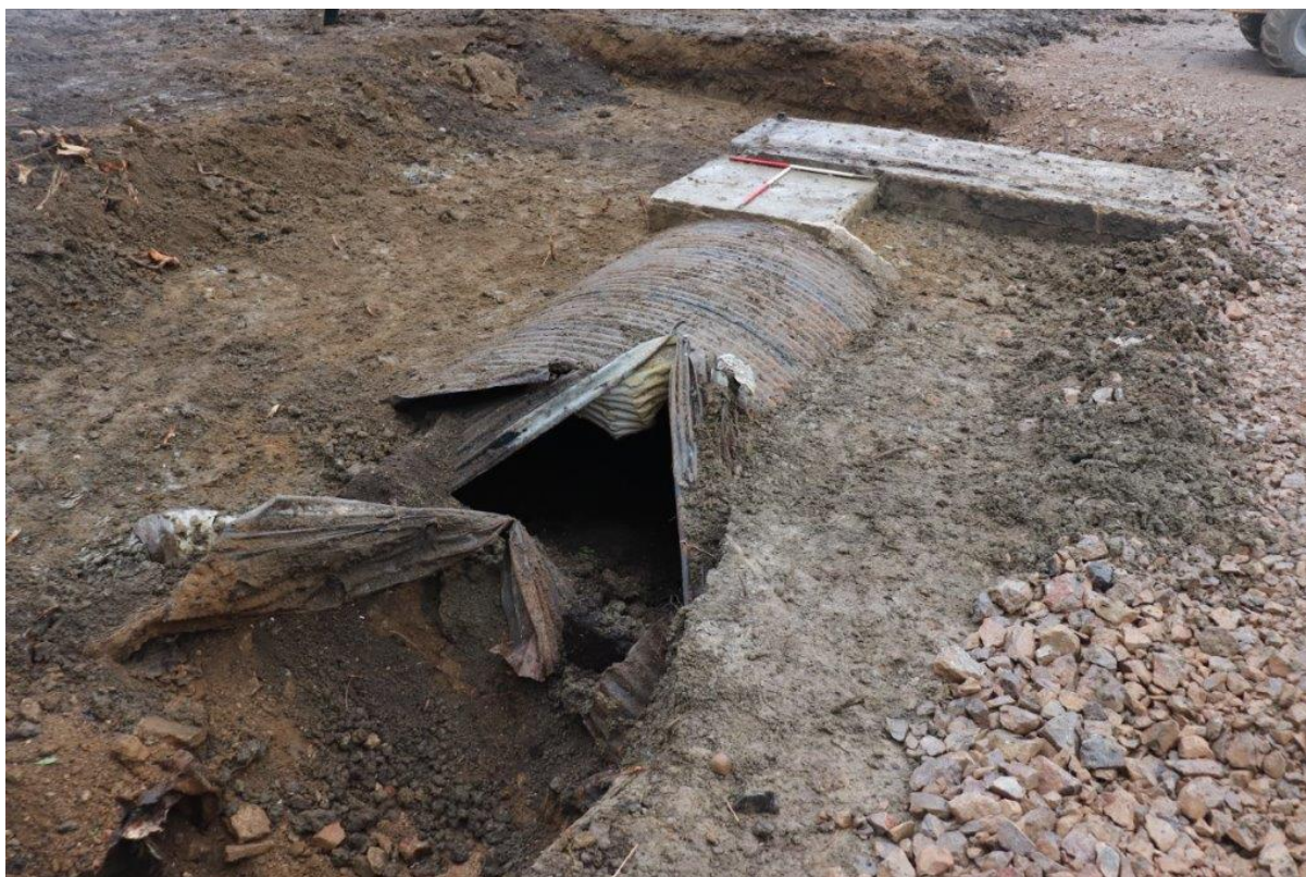
Plate 8: Air-raid shelter when first exposed, showing corrugated roof and concrete entrance. 1m scales looking northeast
