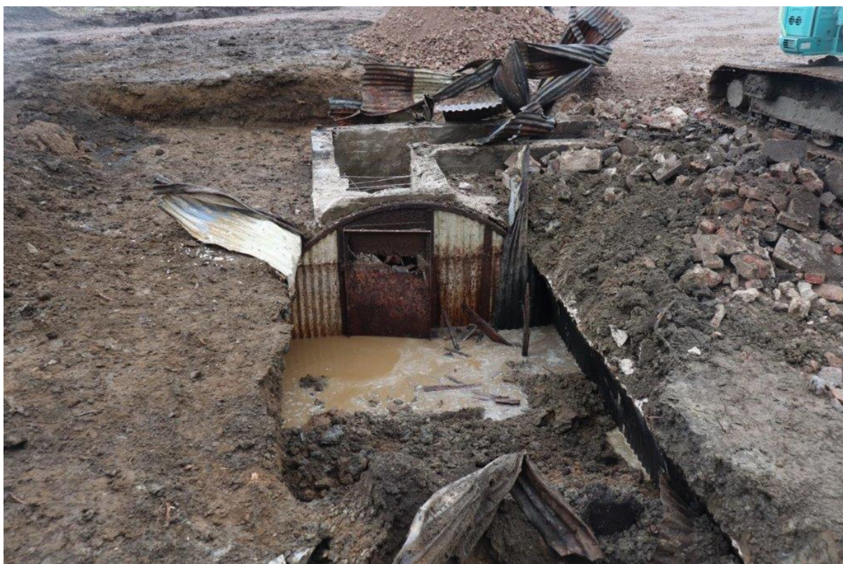
Plate 13: Air-raid shelter when first exposed, showing corrugated roof and concrete entrance looking east
