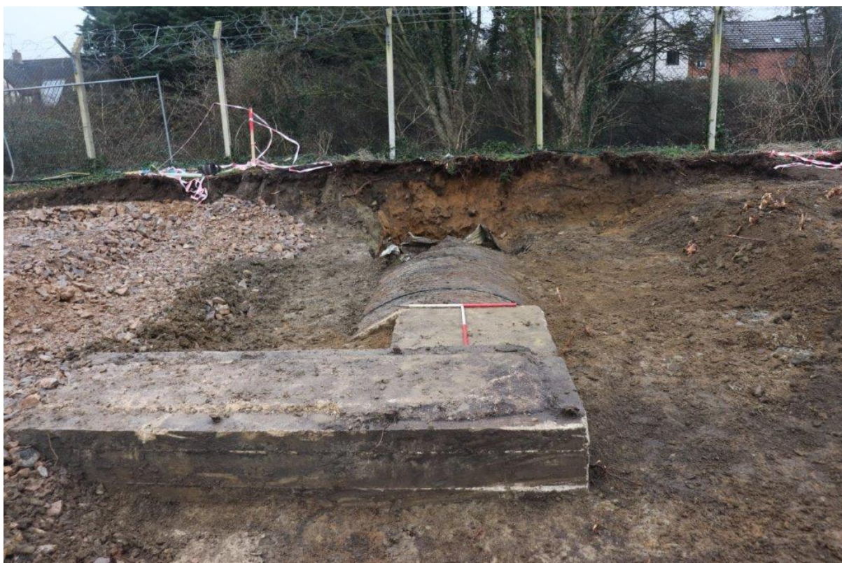
Plate 9: Air-raid shelter when first exposed, showing corrugated roof and concrete entrance. 1m scales looking west
