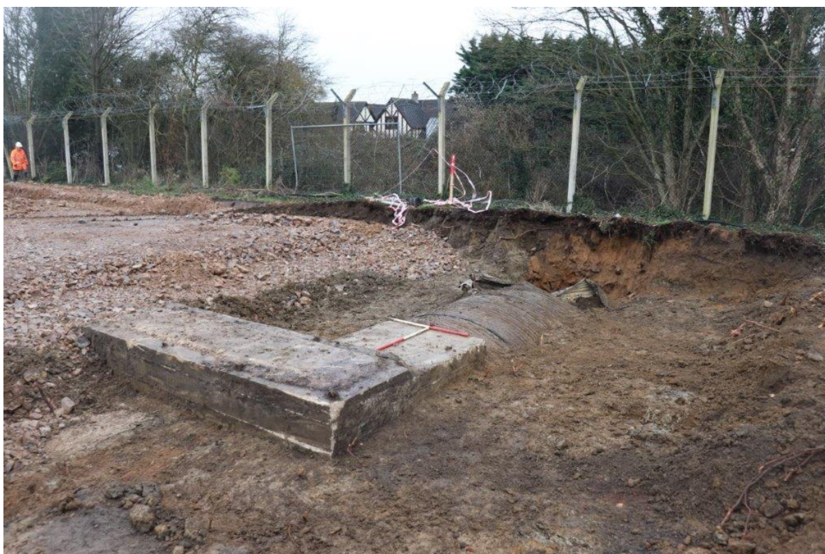
Plate 10: Air-raid shelter when first exposed, showing corrugated roof and concrete entrance. 1m scales looking southwest
