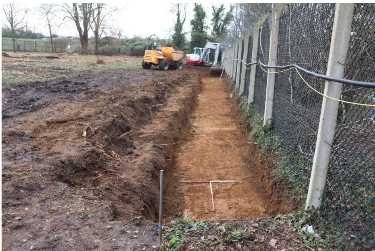
Plate 3: Trench for Gabion wall onto natural firm sand and gravels, 1m scales looking south
