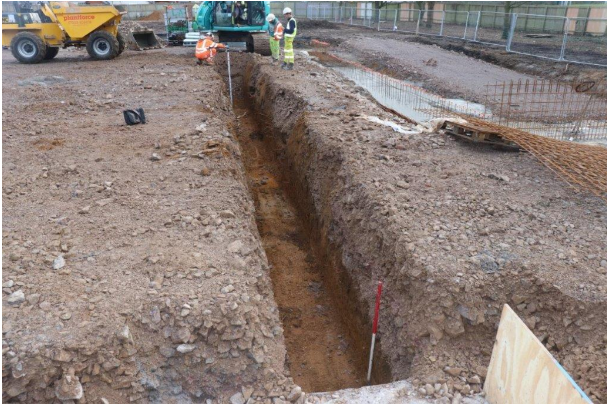
Plate 15: Example of foundation trench excavated through ballast with subsoil and natural below. 1m scale looking north
