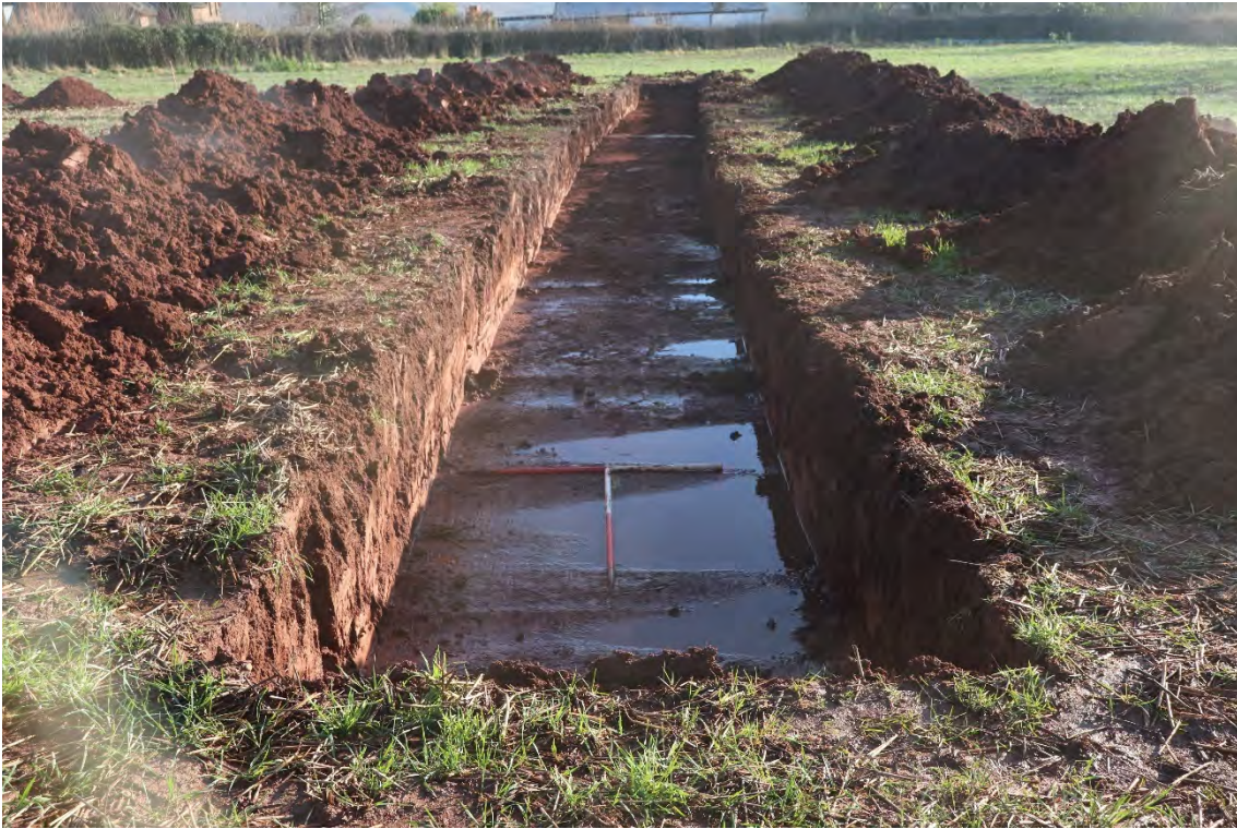
Plate 1: Trench 1 looking south-west; 2x 1m scales
