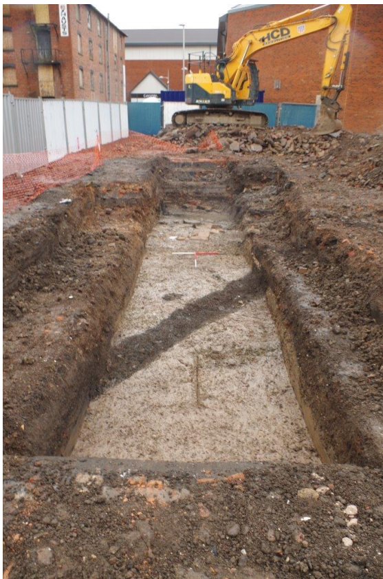
Plate 2 Trench 2, looking north (1m scales)
