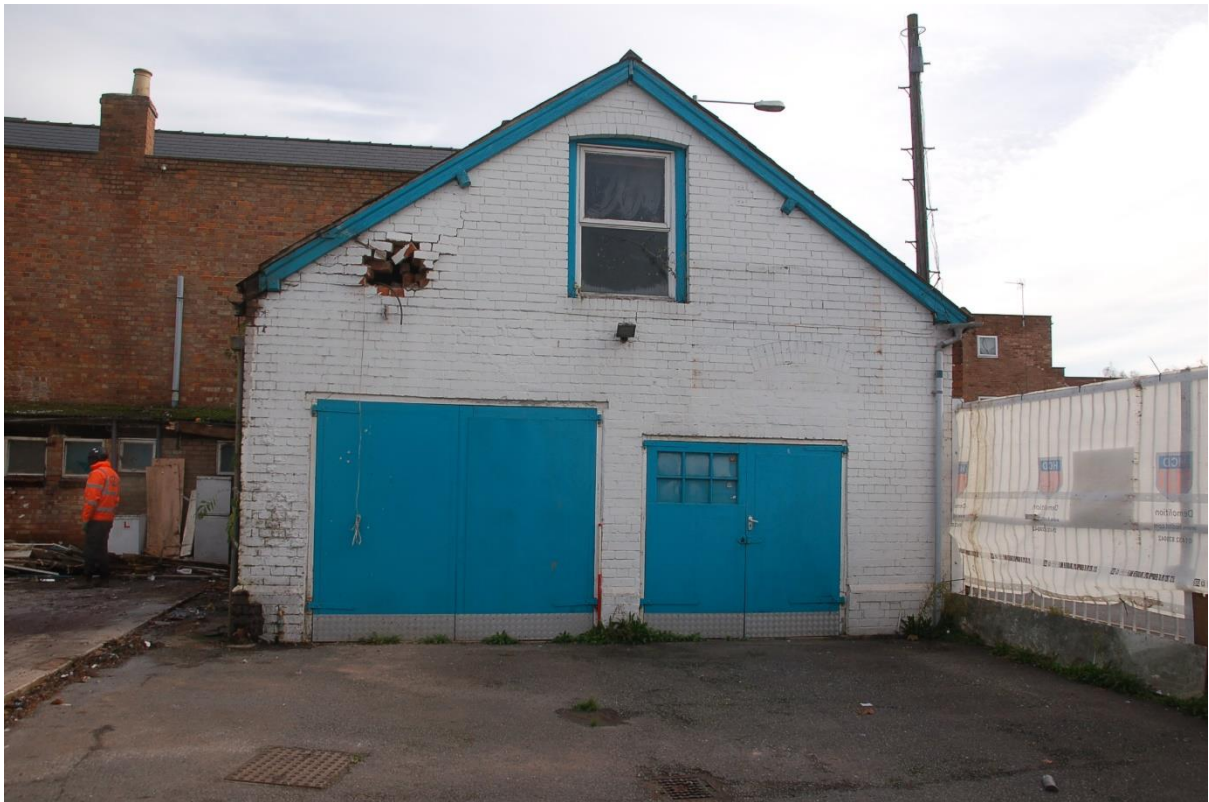
Plate 19 Stables D, looking east
