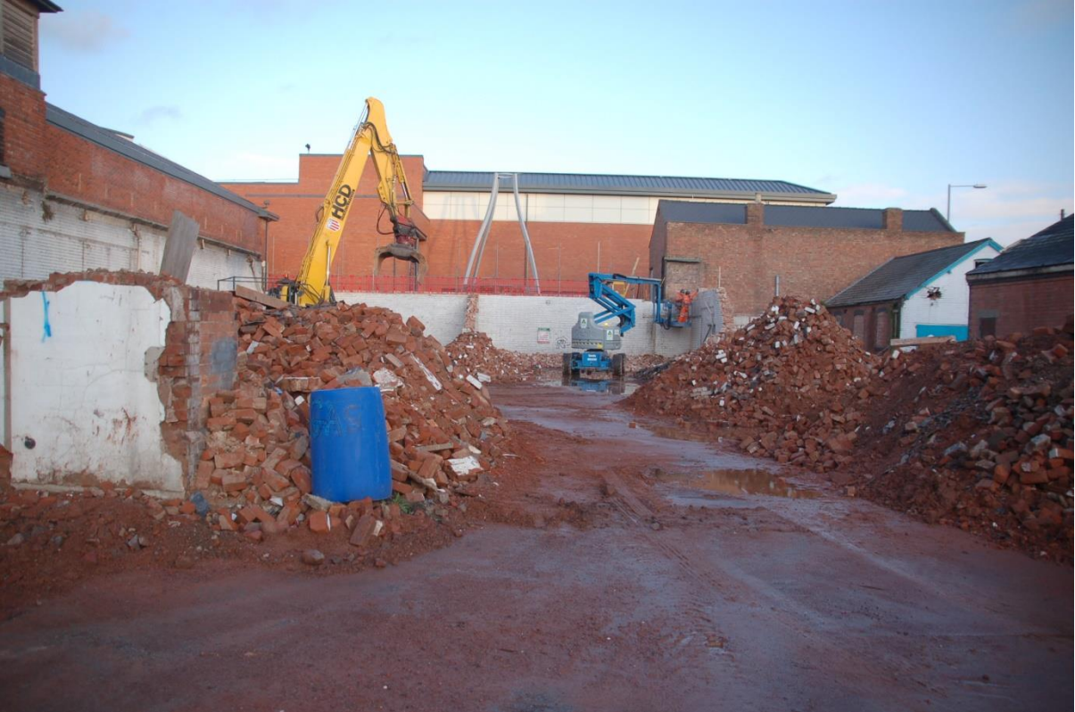
Plate 22 Final stage of monitored demolition, looking east
