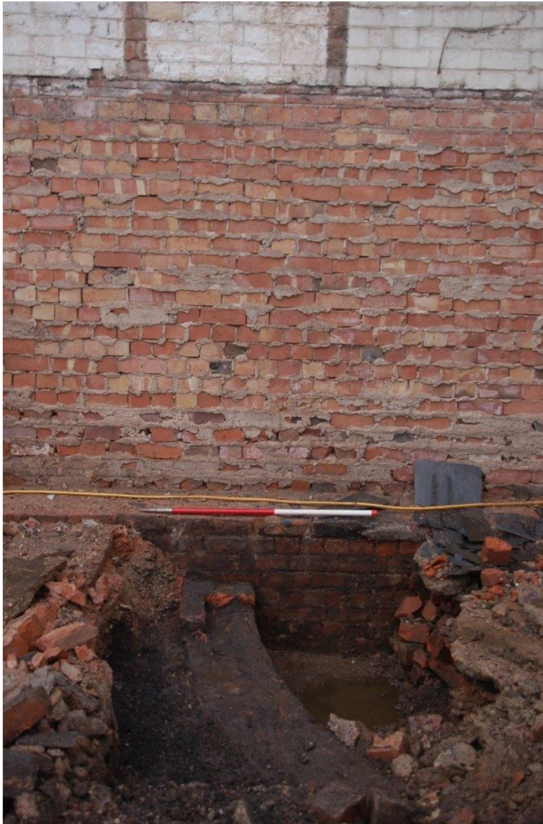
Plate 15 Test Pit 9 showing brick structure 905. Looking east, 1m scale
