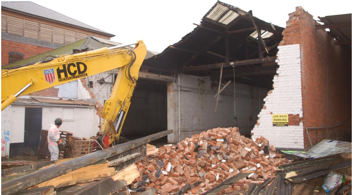
Plate 16 Acidifying shed B2 during early stages of demolition, looking north-east
