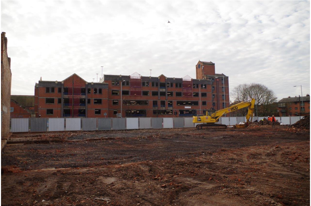
Plate 1 General view of the site, looking south
