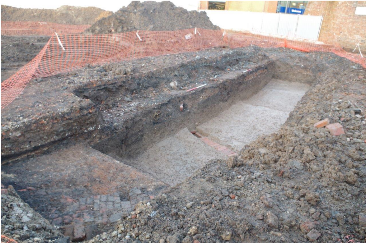
Plate 11 Trench 5, looking north-east. 1m scales
