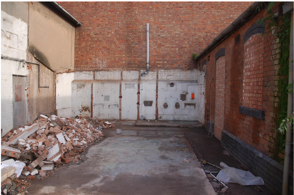
Plate 21 Removal of toilet block, looking east
