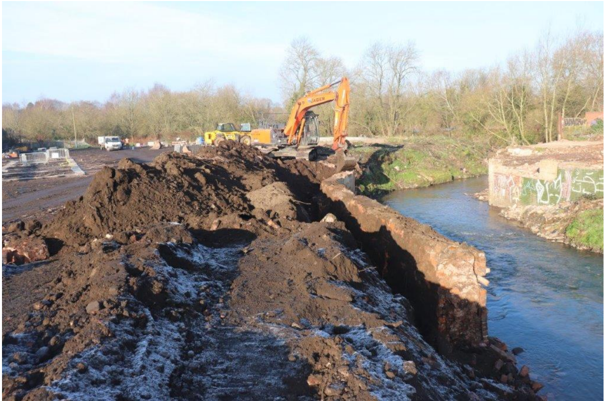
Plate 9: Trench excavated behind retaining wall in west of site, view north-west
