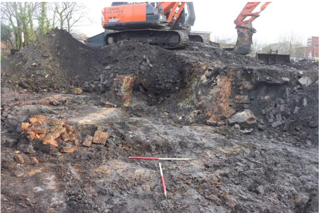
Plate 2: Brick walls of mid-20 th century cellars in the centre of the site, view south-east, 1m scales
