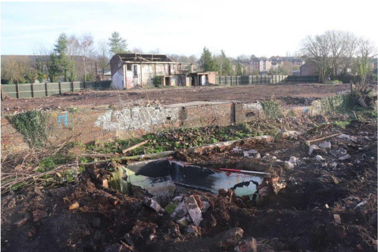
Plate 4: Modern drainage chamber on surface, view north-west, 1m scale
