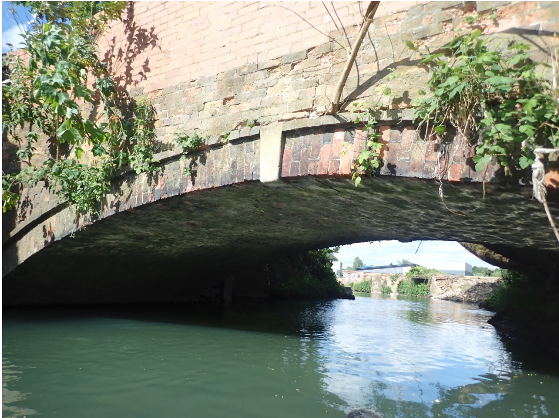
Plate 21: Eastern face of the bridge from river level, showing brick edgings and keystone, view west
