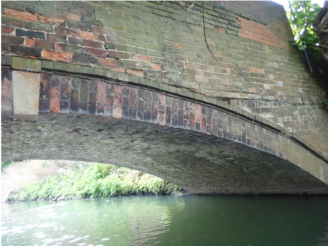
Plate 19: The underside and west face of the bridge, view south-east
