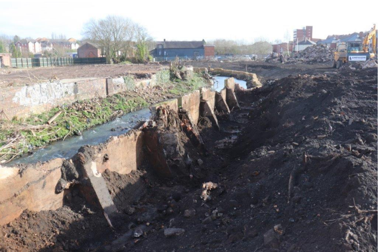
Plate 6: The trench excavated behind the retaining wall before wall removal, view east
