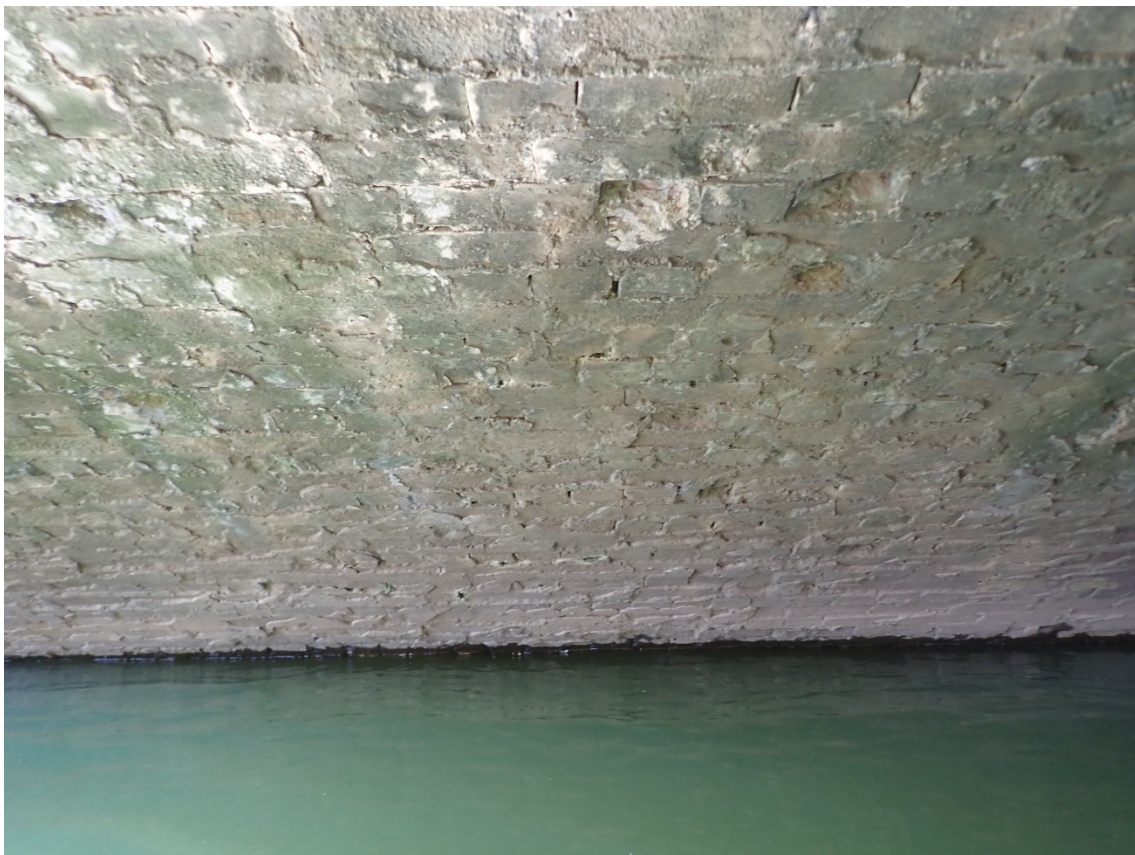
Plate 20: The arched brick underside of the bridge, view south
