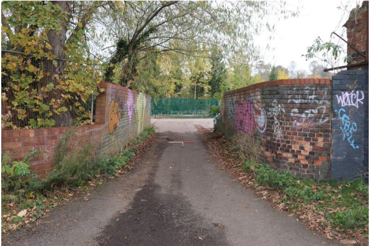
Plate 13: View north of bridge Bradley Road towards Canal Street, 1m scales
