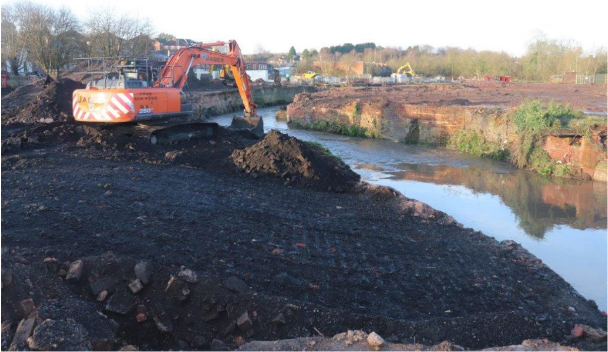
Plate 1: The site along river edge as works started, view west
