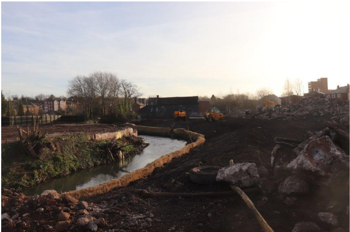
Plate 8: The bank profiled following wall removal, view east
