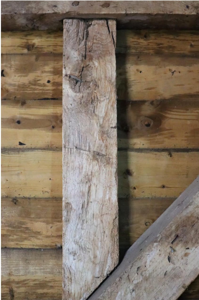
Plate 4 Timber with a notch mark cut aligned at 90° to the timber with a short bladed axe, most likely a felling axe, no scale
