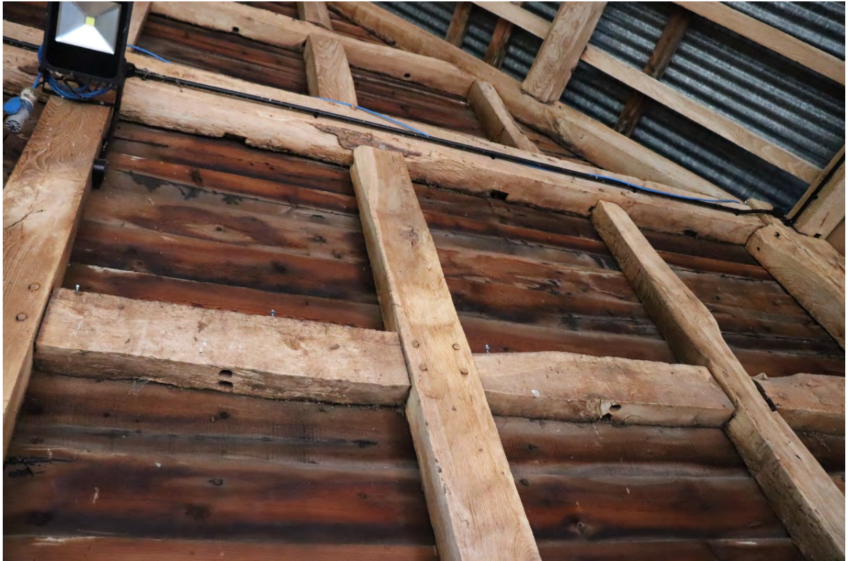
Plate 12 Single and double pegholes as well as small lapped joints central to each panel. Note no such corresponding features at the edge of the panels, as would typically be the case, no scale
