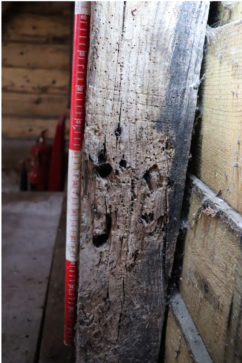
Plate 11 Reused timber next to a redundant pegged mortice joint, with the “III” mark being redundant carpenters marks, looking north-east
