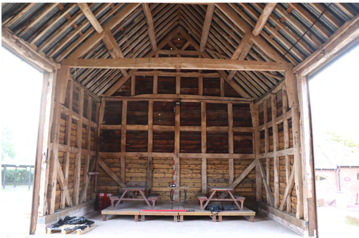
Plate 10 Interior end and intermediary cross frames, looking south-east, 2m scale
