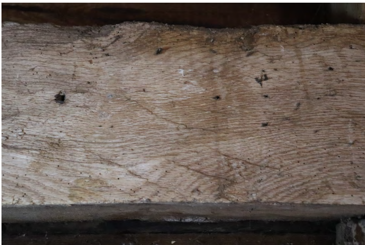
Plate 5 Timber with shallow curved cut marks typical of a side axe, no scale
