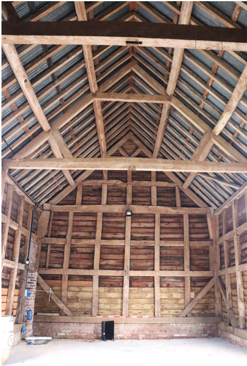
Plate 9 Interior end and intermediary cross frames, looking north-west, 2m scale
