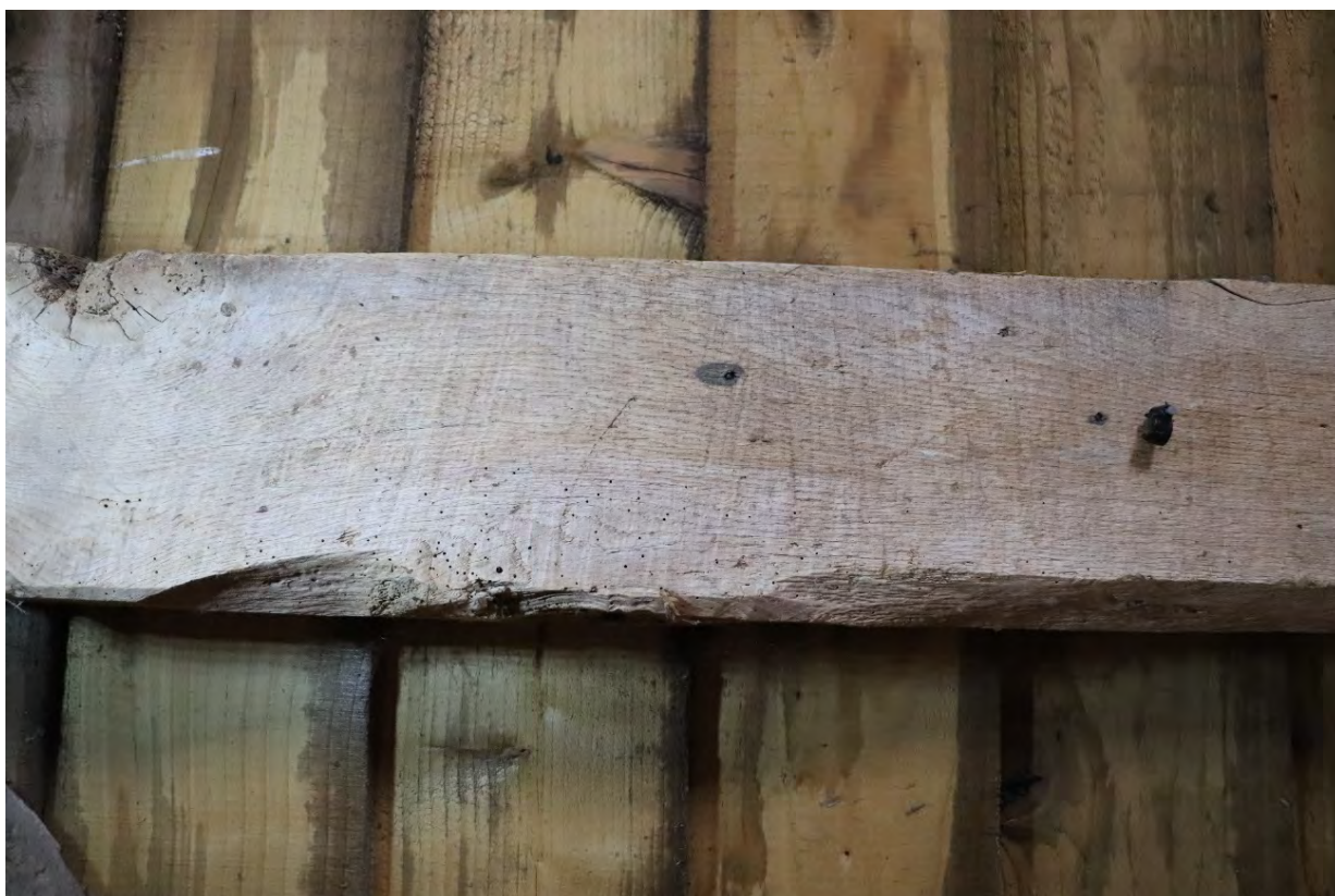
Plate 7 Timber with slightly off 90 degree fairly irregular saw marks, typical of pit or double trestle sawing, no scale
