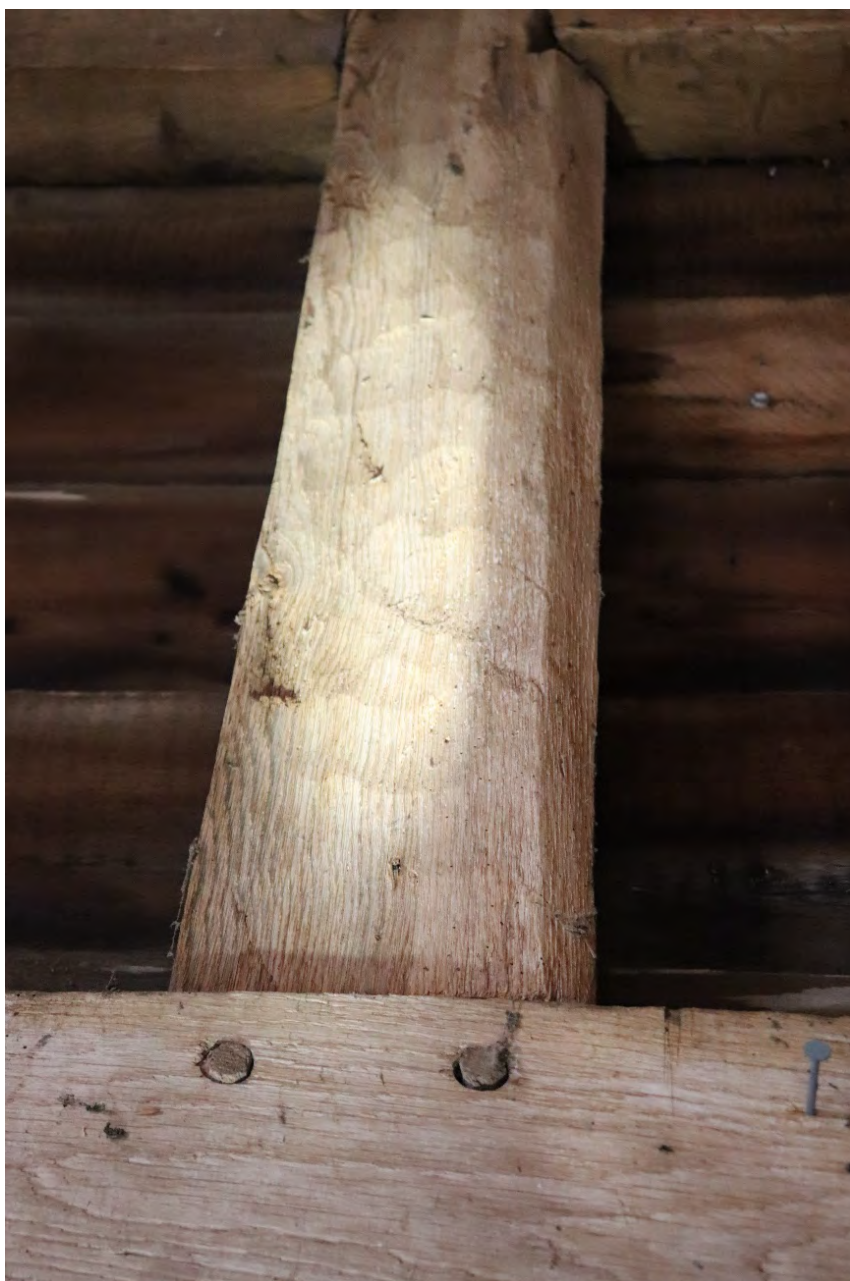
Plate 6 Timber with shallow scalloped marks, typical of an adze, no scale
