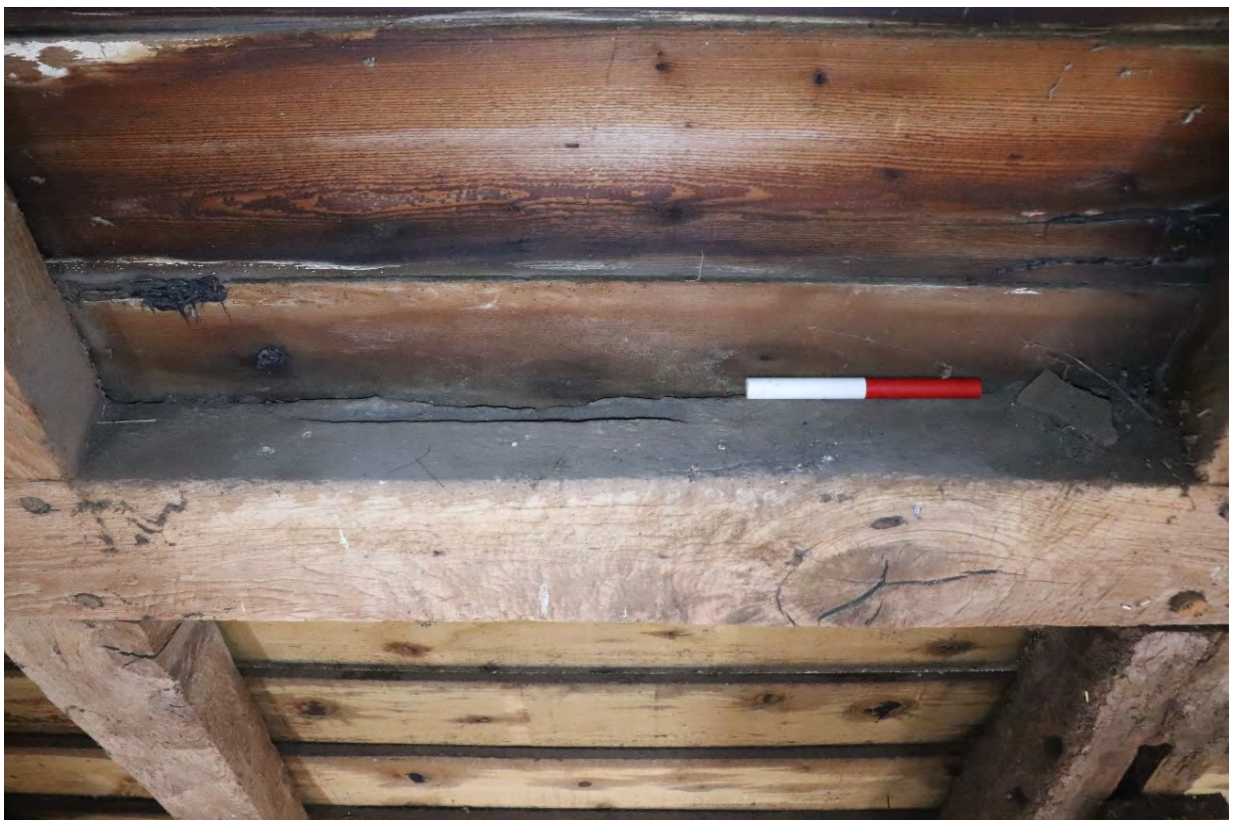
Plate 13 Groove with vertical stop closest to the 0.20m scale that runs out at opposing end
