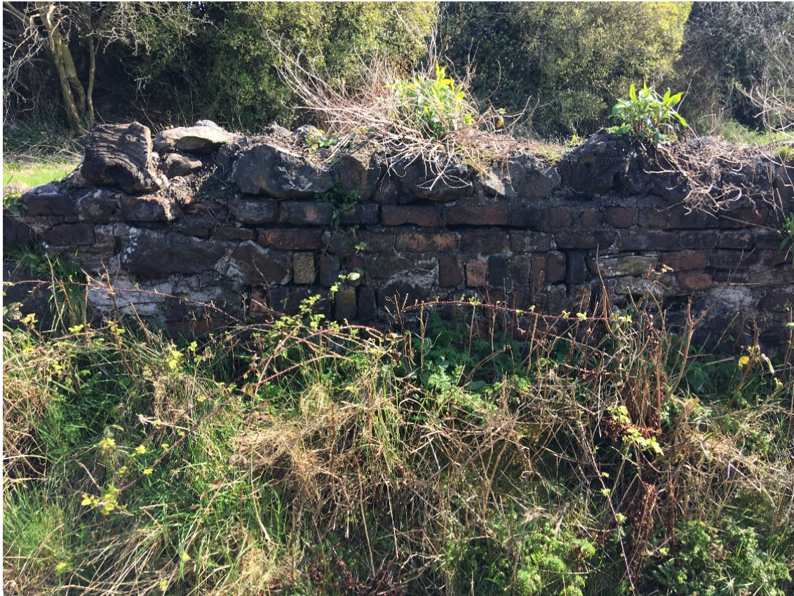
Plate 4 The wall, looking south-east
