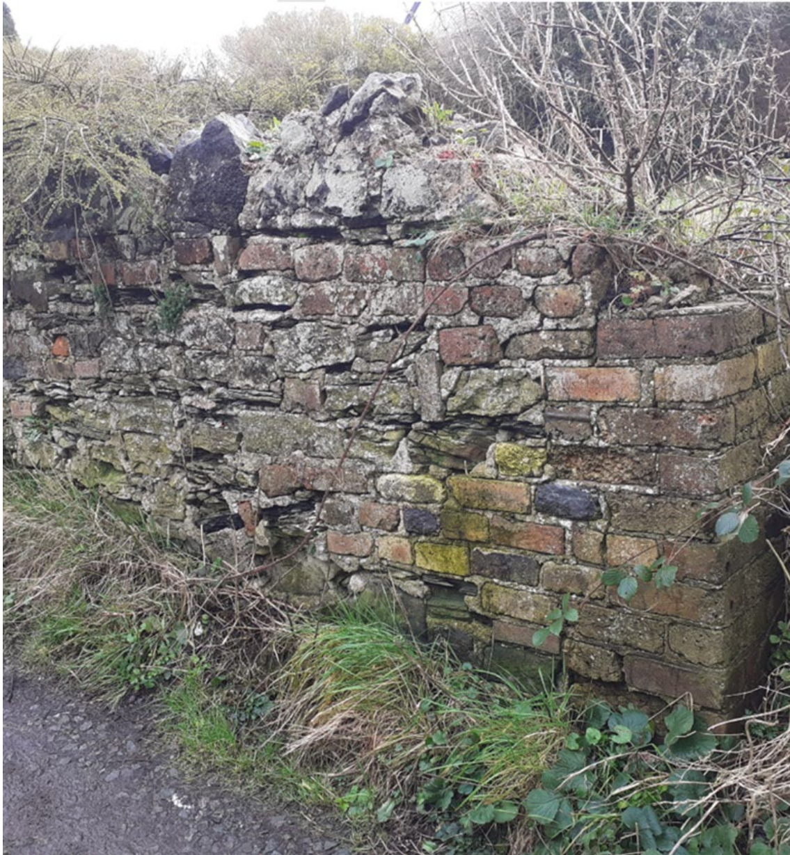
Plate 3 The wall, detail of south end, looking north-east
