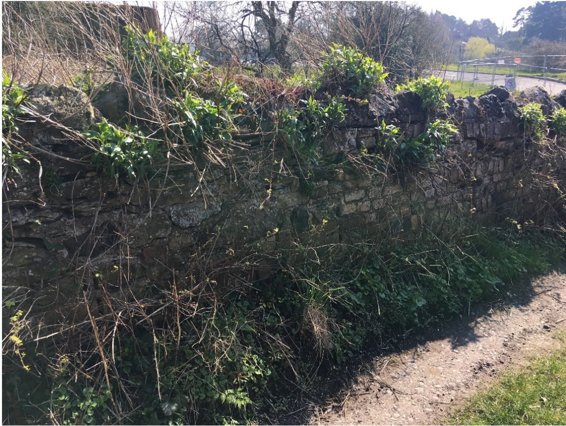
Plate 6 The wall, looking south
