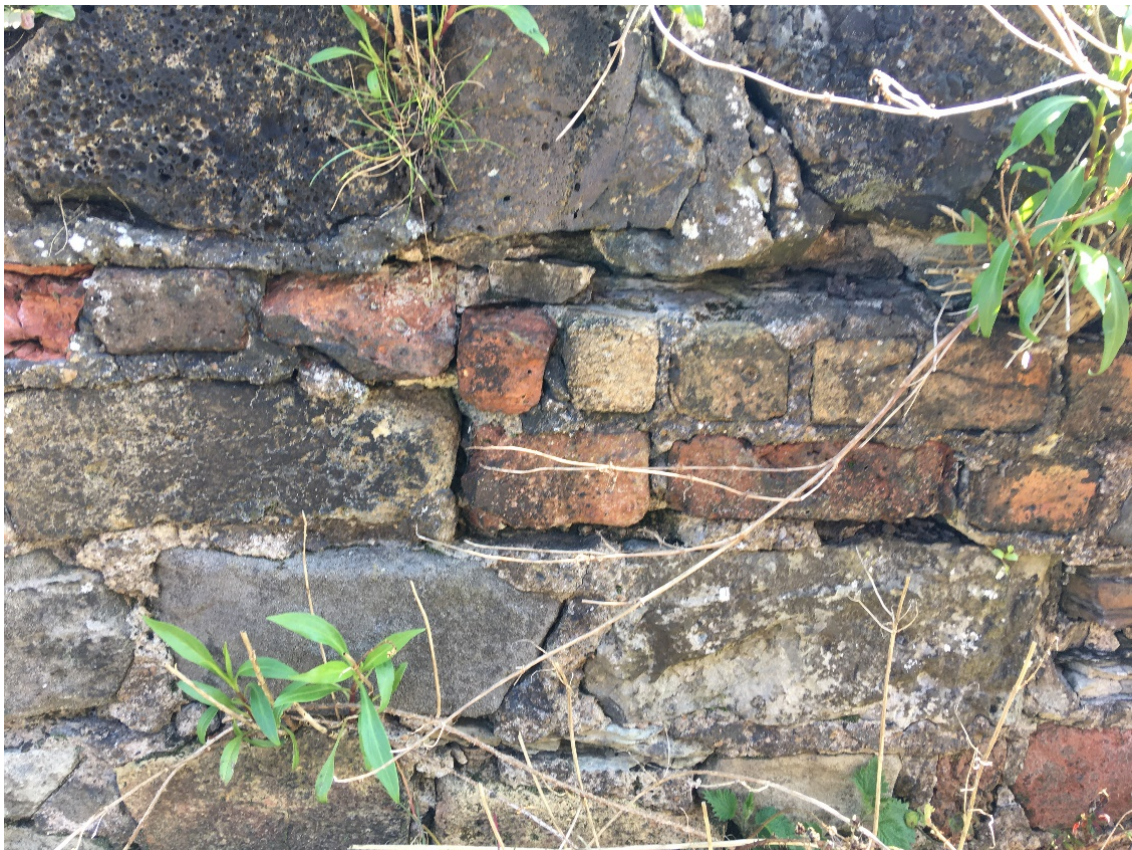
Plate 5 The wall, detail, looking south-east
