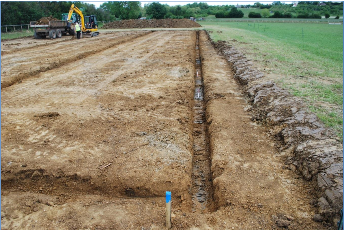
Plate 2 Drainage run looking north-east
