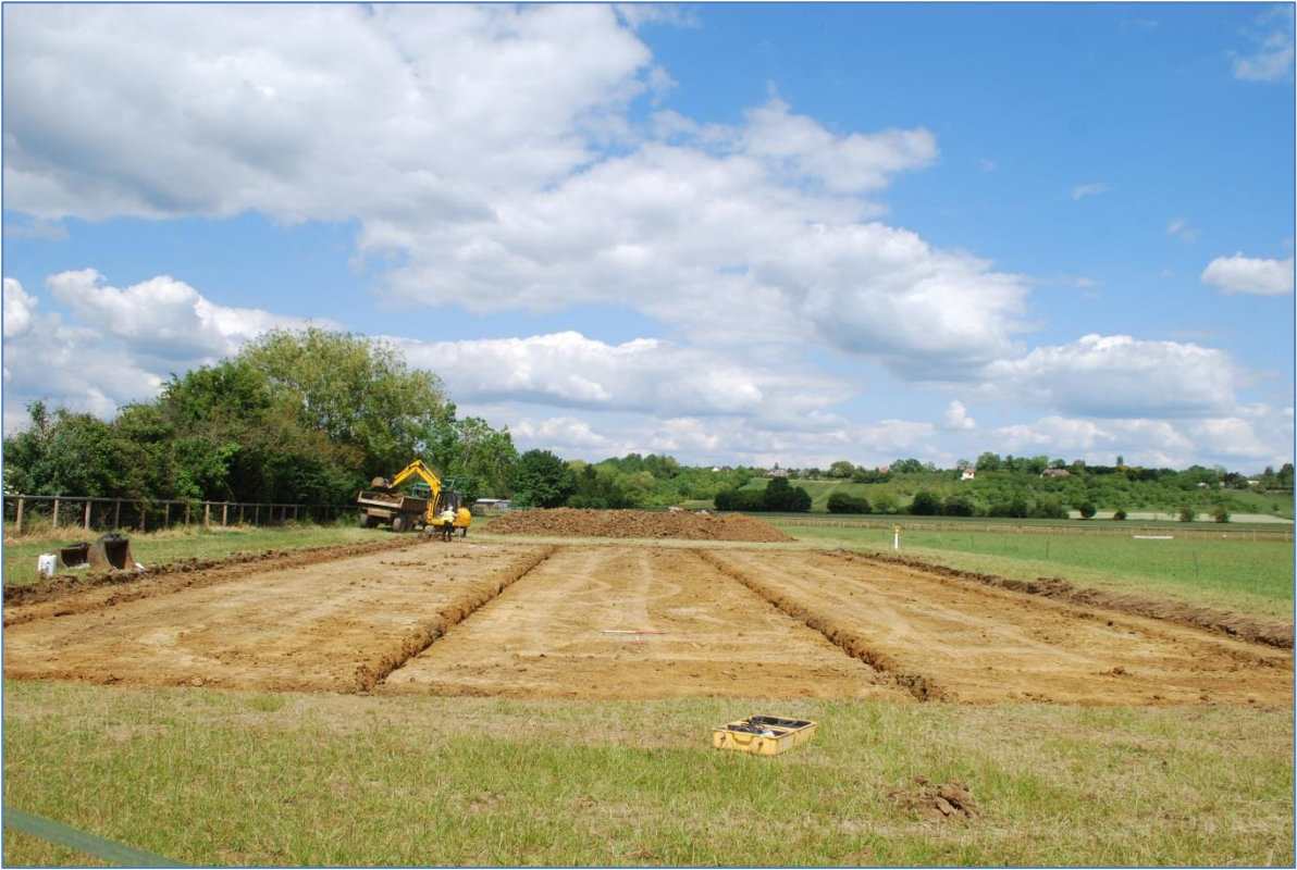
Plate 3 Drainage channels excavated looking Northeast
