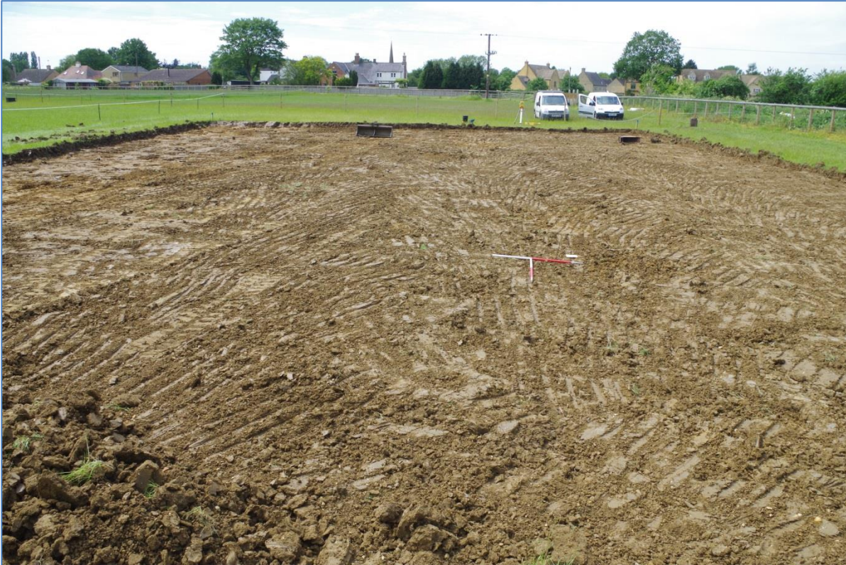
Plate 1 Topsoil strip of menage looking Southwest
