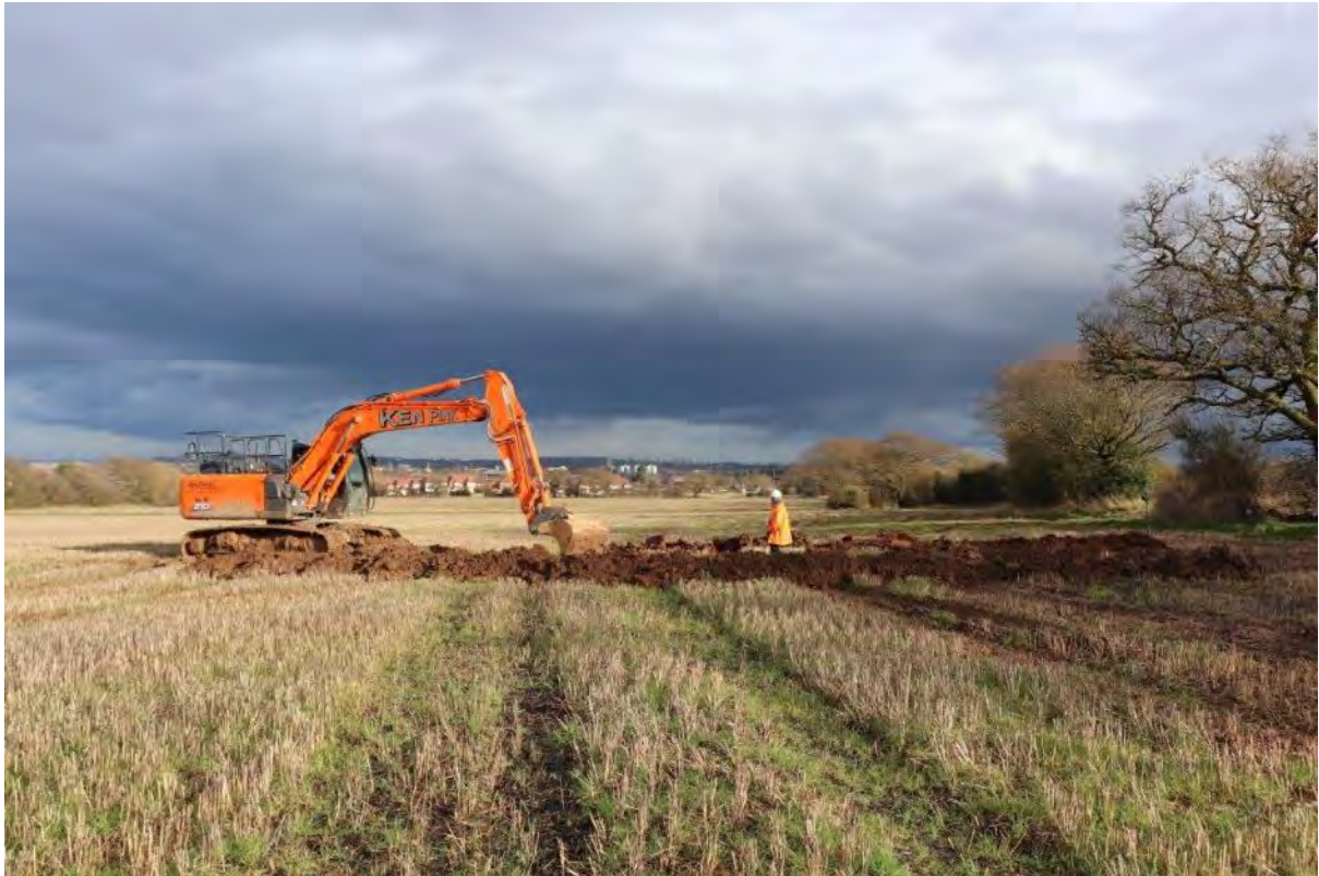
Plate 17: Looking east across to Trench 68 with excavation in progress.
