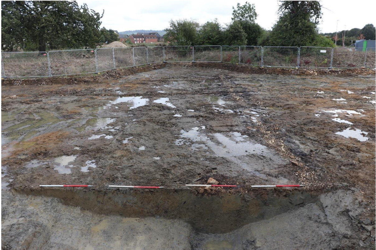
Plate 21: West facing section of large post-medieval boundary ditch CG33. 1m scales.
