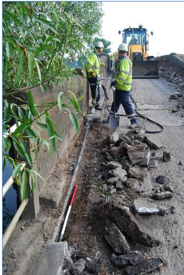
Plate 4 Breaking out the concrete along the parapet walls to reveal service cables
