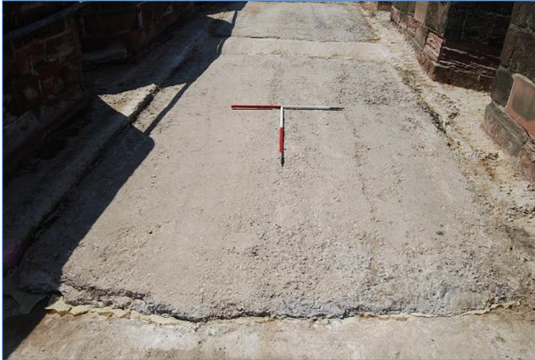
Plate 9 The concrete saddling between the arches after cleaning, looking south-west
