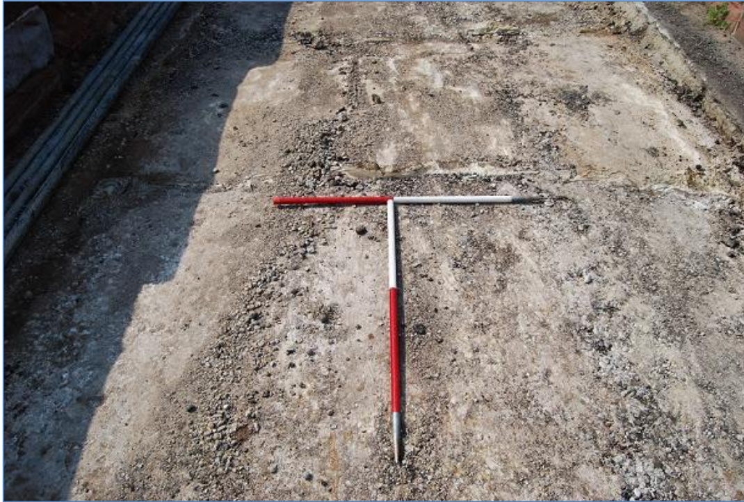
Plate 7 Example of saddling concrete and underlying plastic sheeting between the bridge arches before cleaning
