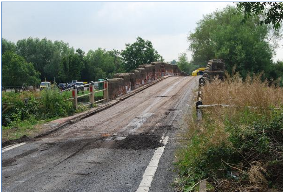
Plate 2 The road surface following planing, looking south
