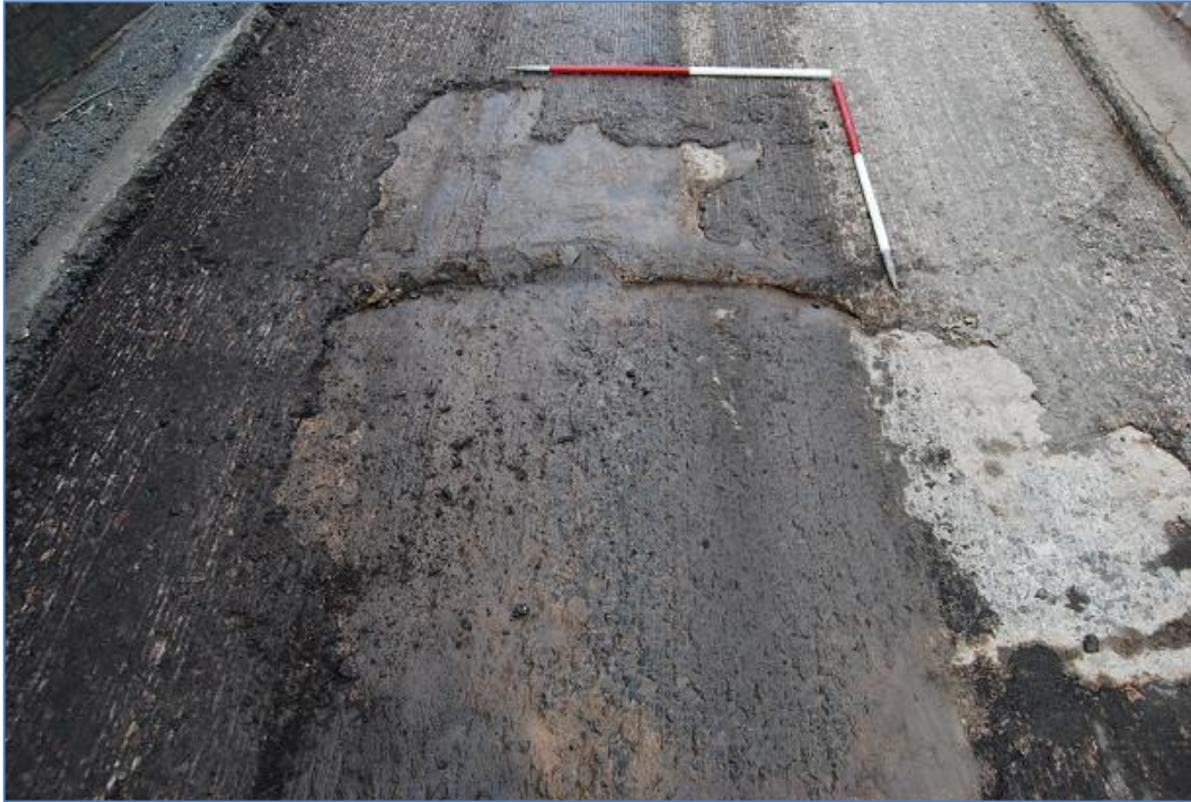
Plate 3 Uneven concrete that had caused cracking in the tarmac carriageway
