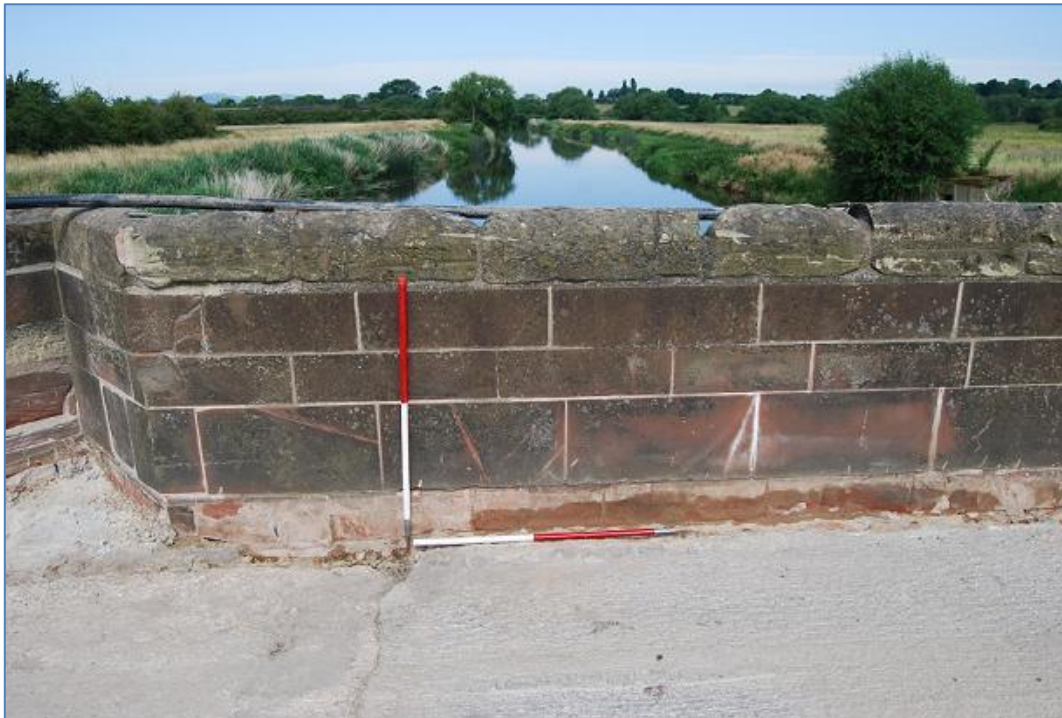
Plate 13 Example of parapet wall with sandstone revealed on north-west side of bridge, view west
