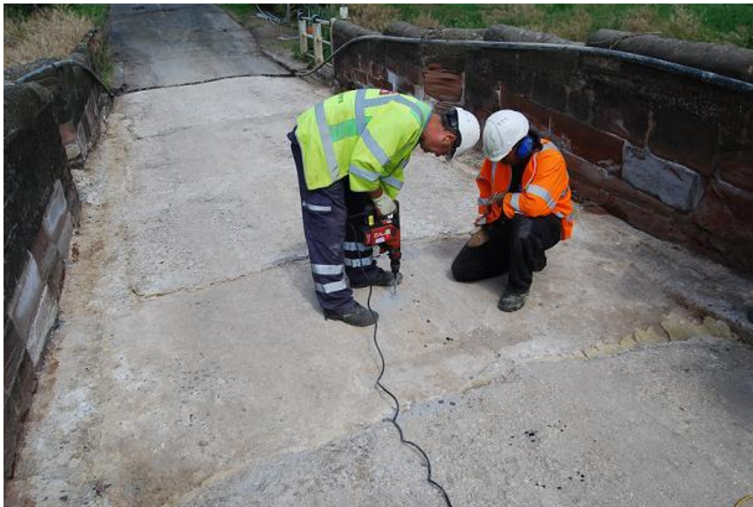
Plate 10 Example of drilling holes through the concrete in the centre of each arch, looking east
