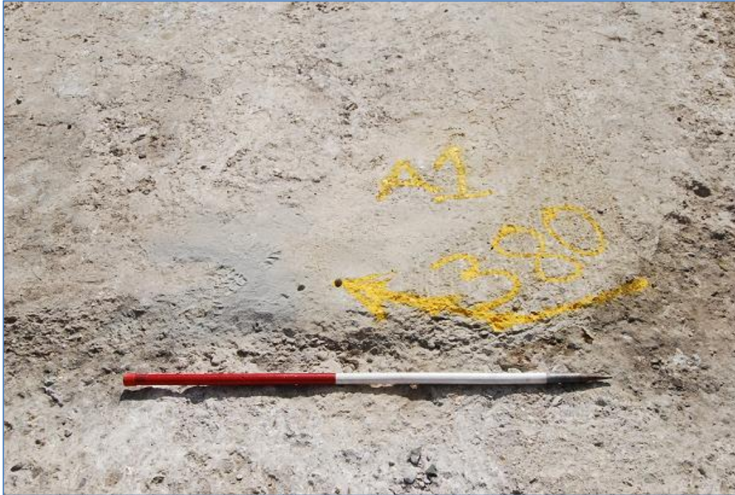
Plate 15 Example drill hole in arch 1; concrete is 380mm in depth overlying the sandstone bridge
