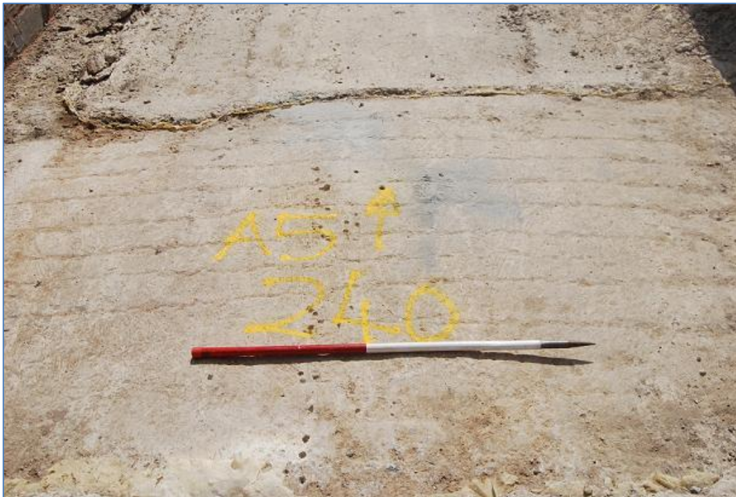
Plate 16 Example of drill hole in arch 5; concrete is 240mm in depth down to sandstone bridge
