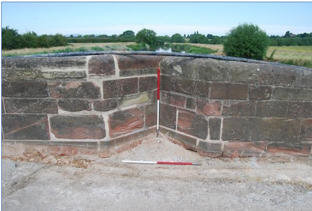
Plate 14 Refuge on Northwest side of bridge with sandstone revealed, view west
