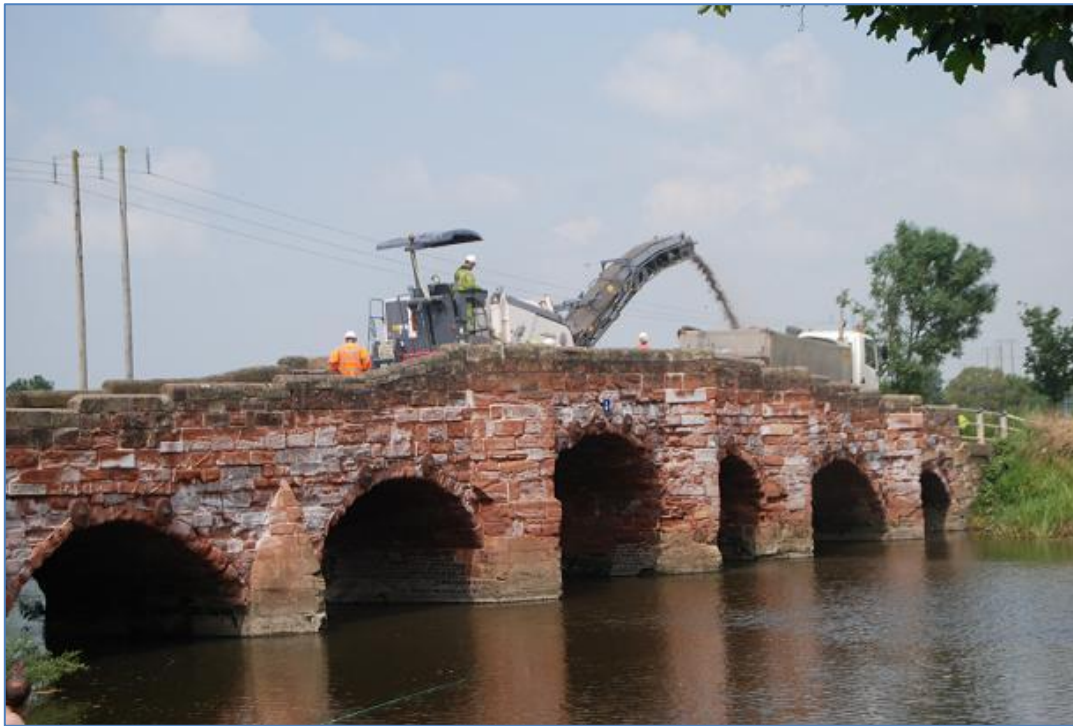
Plate 1 Planing top tarmac surface off the bridge, looking north
