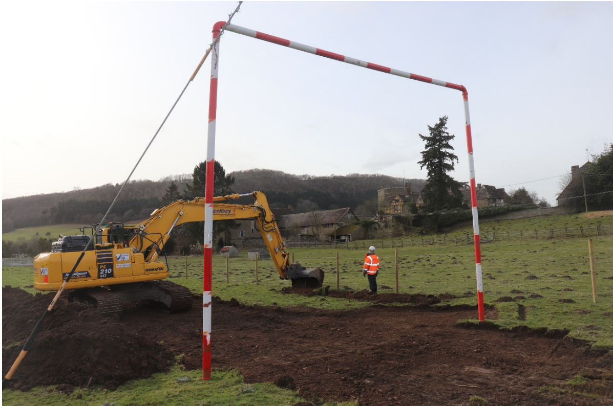
Plate 5: Easement topsoil strip with Stokesay Castle in background. looking southwest.
