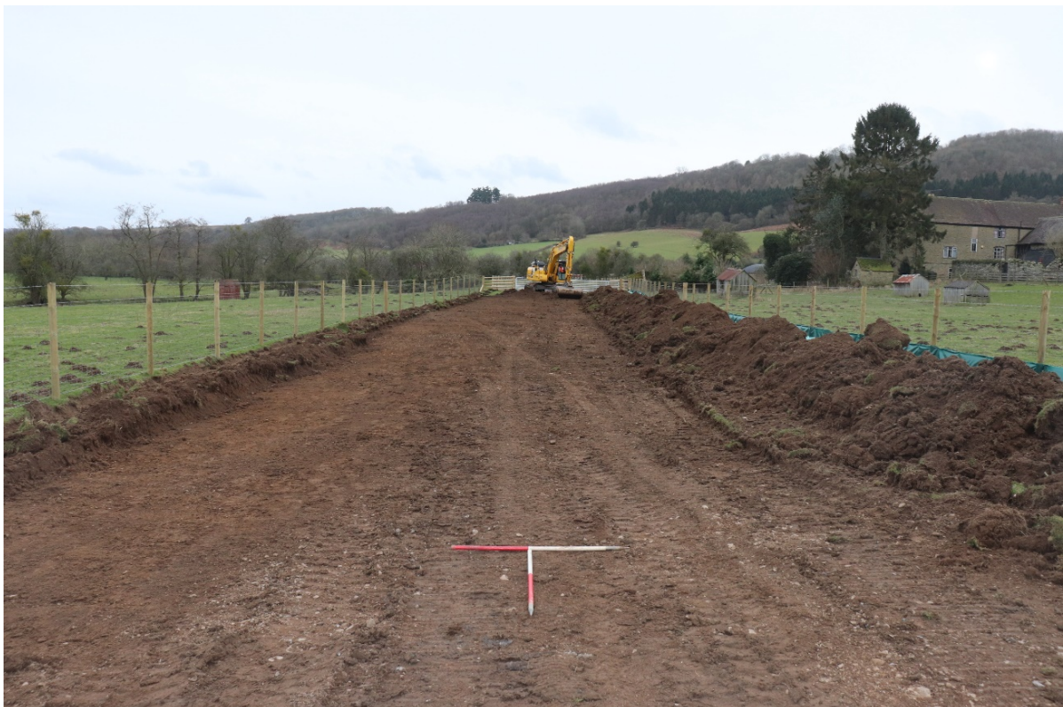
Plate 6: Easement topsoil strip looking south with 1m scales.
