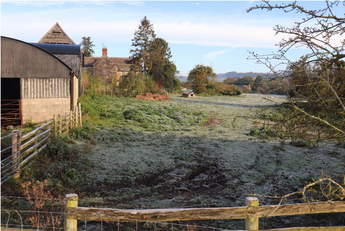
Plate 1: Scheduled Monument area of Stokesay Castle on initial site visit, prior to works commencing. From southern boundary looking north.
