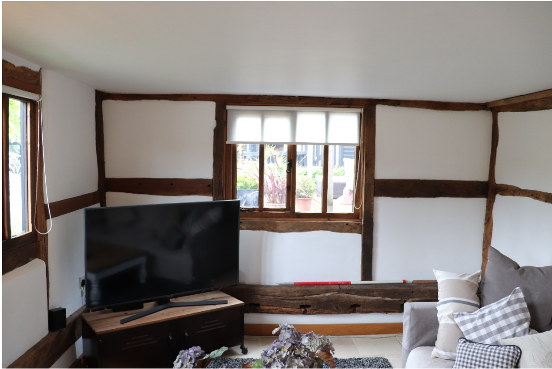
Plate 10 Phase 2 additional southern bay, looking south, 1m scale
