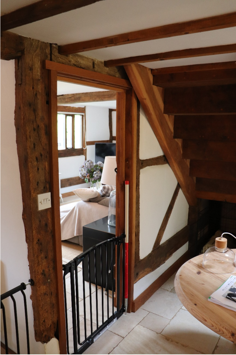
Plate 4 Phase 1 former exterior wall, looking south-west, 1m scale
