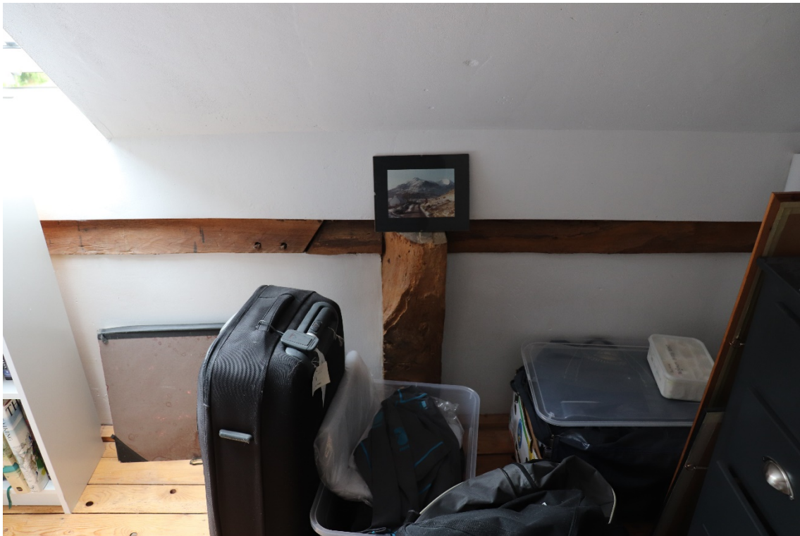
Plate 8 Phase 1 former bay frame jowl post, looking east
