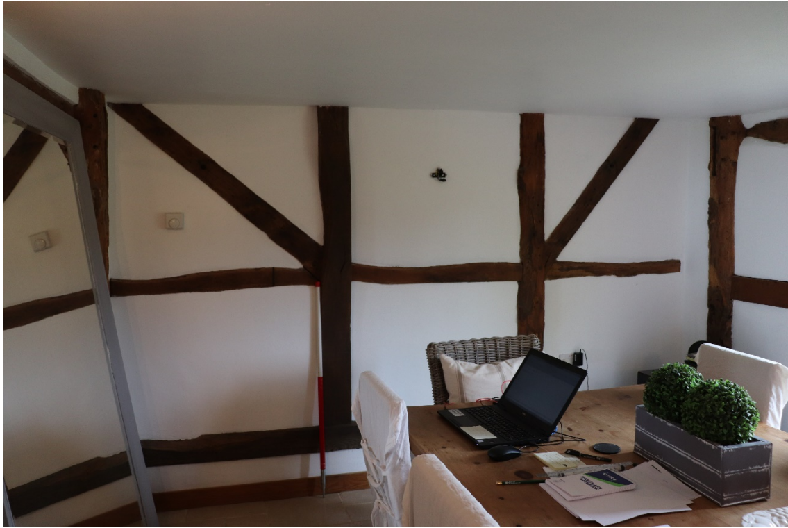
Plate 13 Phase 2 additional northern structure, looking north, 1m scale
