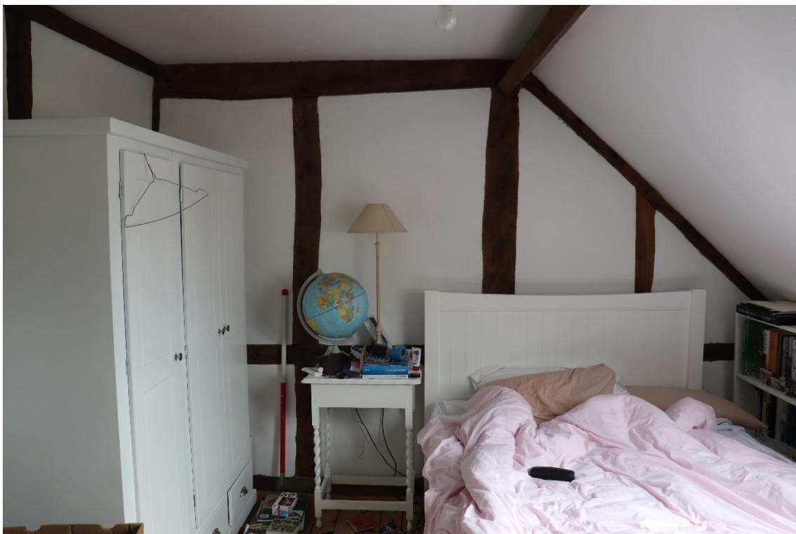
Plate 16 Phase 3 first floor room and inserted timbers, looking north, 1m scale
