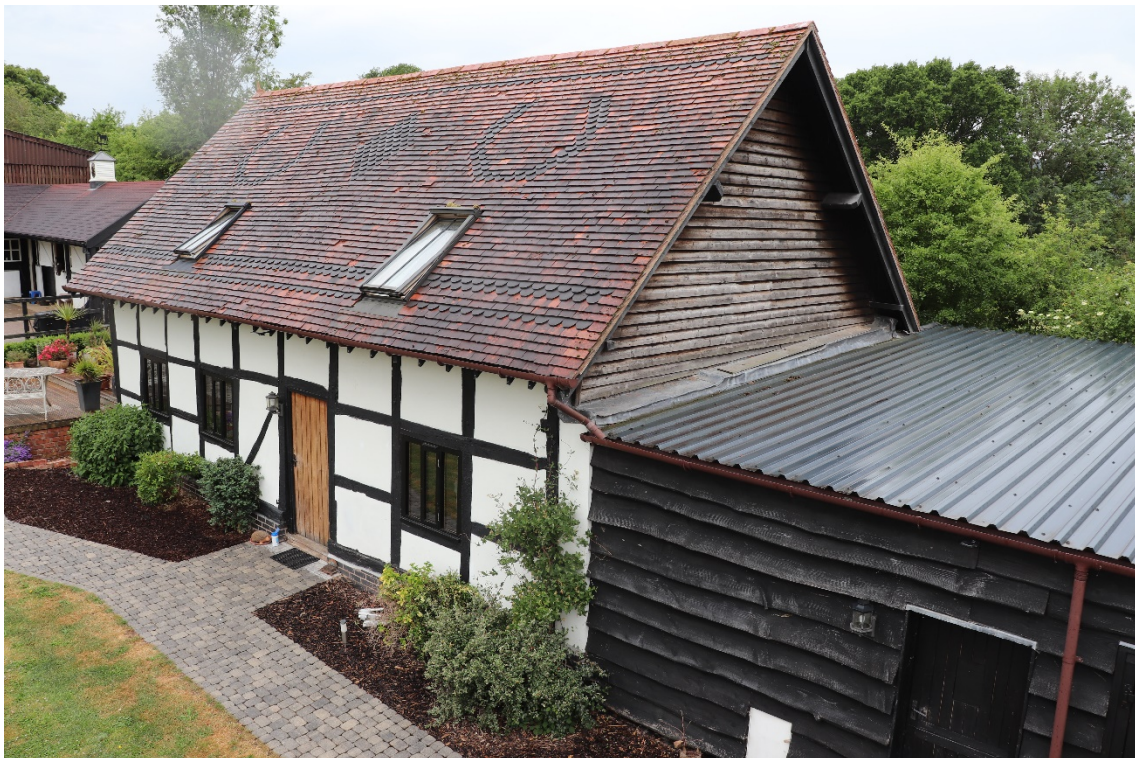
Plate 2 The building looking south-east
