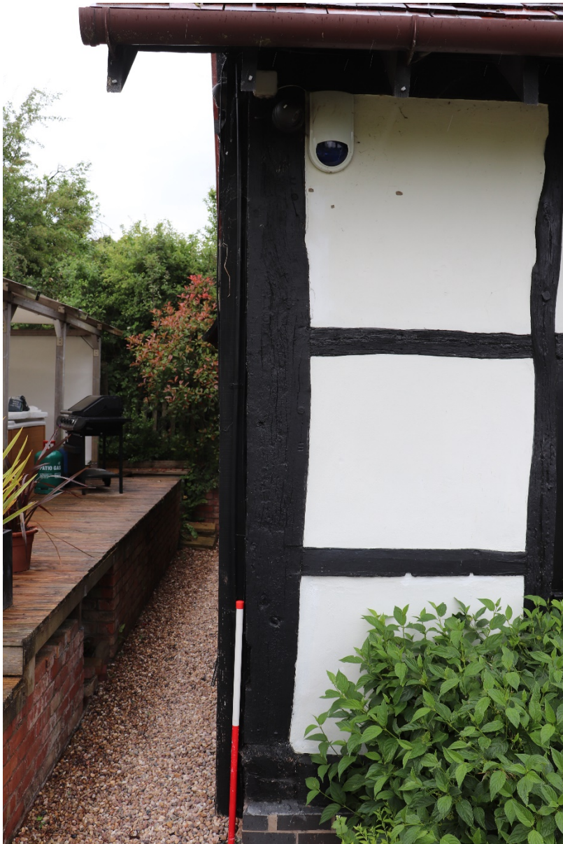
Plate 12 Re-used former tie within the Phase 2 additional southern bay, looking south, 1m scale
