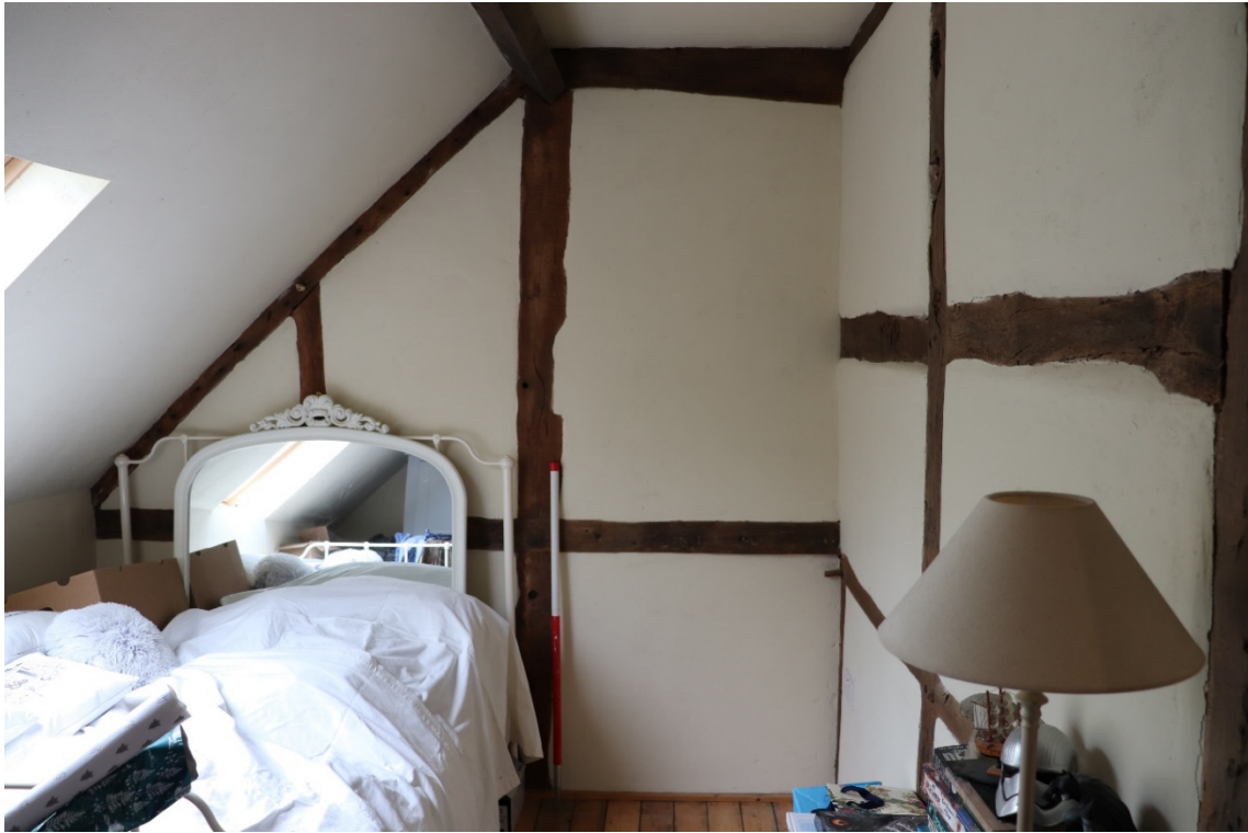
Plate 17 Phase 3 first floor room and inserted timbers, looking north, 1m scale
