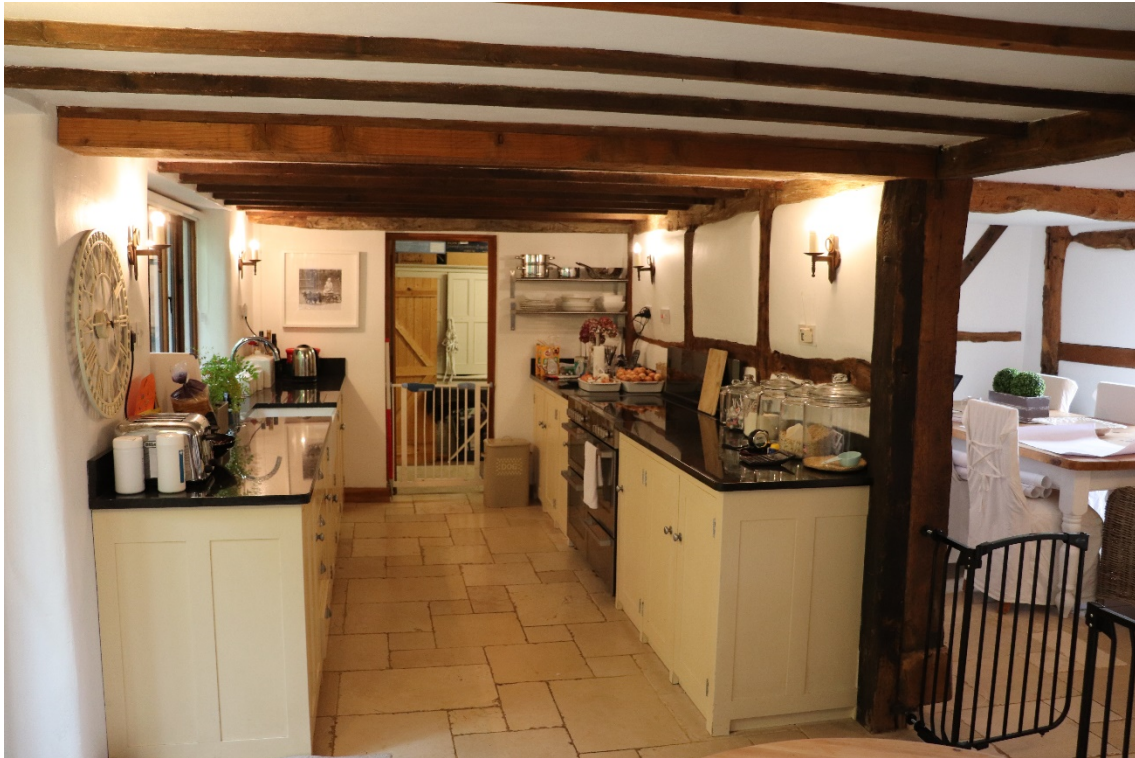
Plate 15 Phase 3 kitchen, looking north, 1m scale
