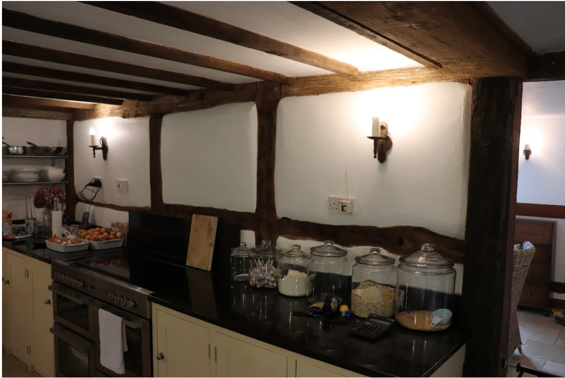
Plate 3 Phase 1 former exterior wall, looking north-east
