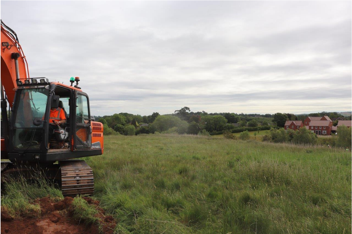
Plate 1 General view across site, looking north
