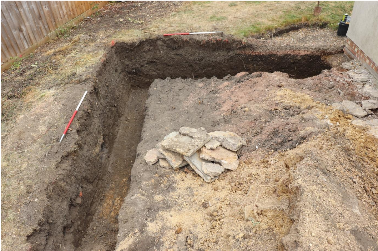
Plate 3: SE and SW facing sections of Trench 2 showing the made ground layer 202, the driveway 204, and the foundations of the previous extension. 2x1m scale, facing north east
