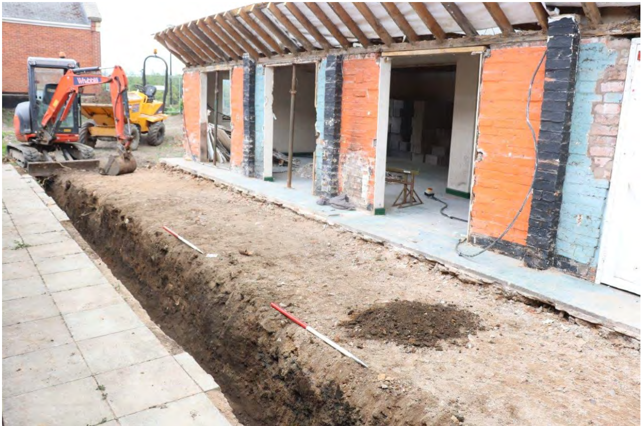
Plate 1 Trench 1 looking north (1m scales)
