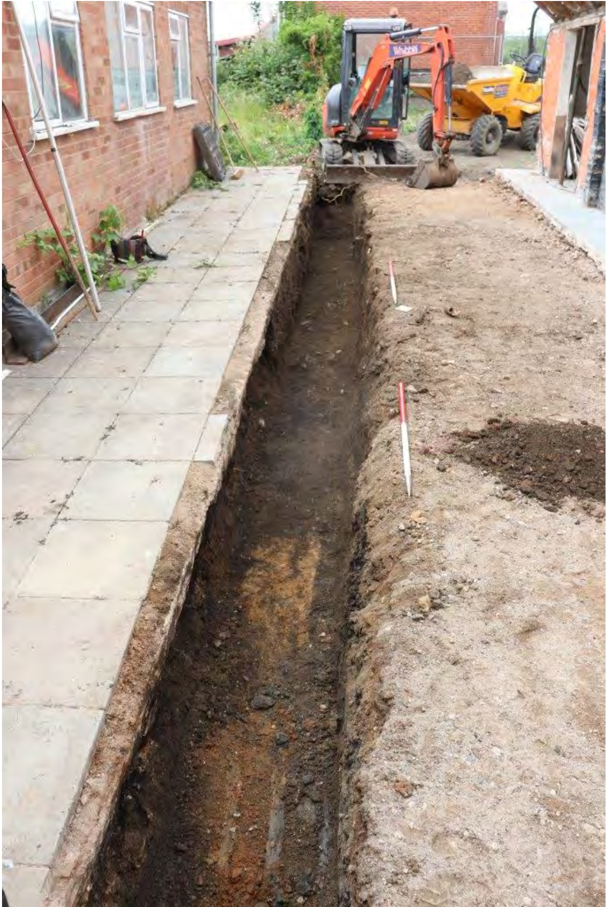
Plate 2 Trench 1 looking north-west (1m scales)
