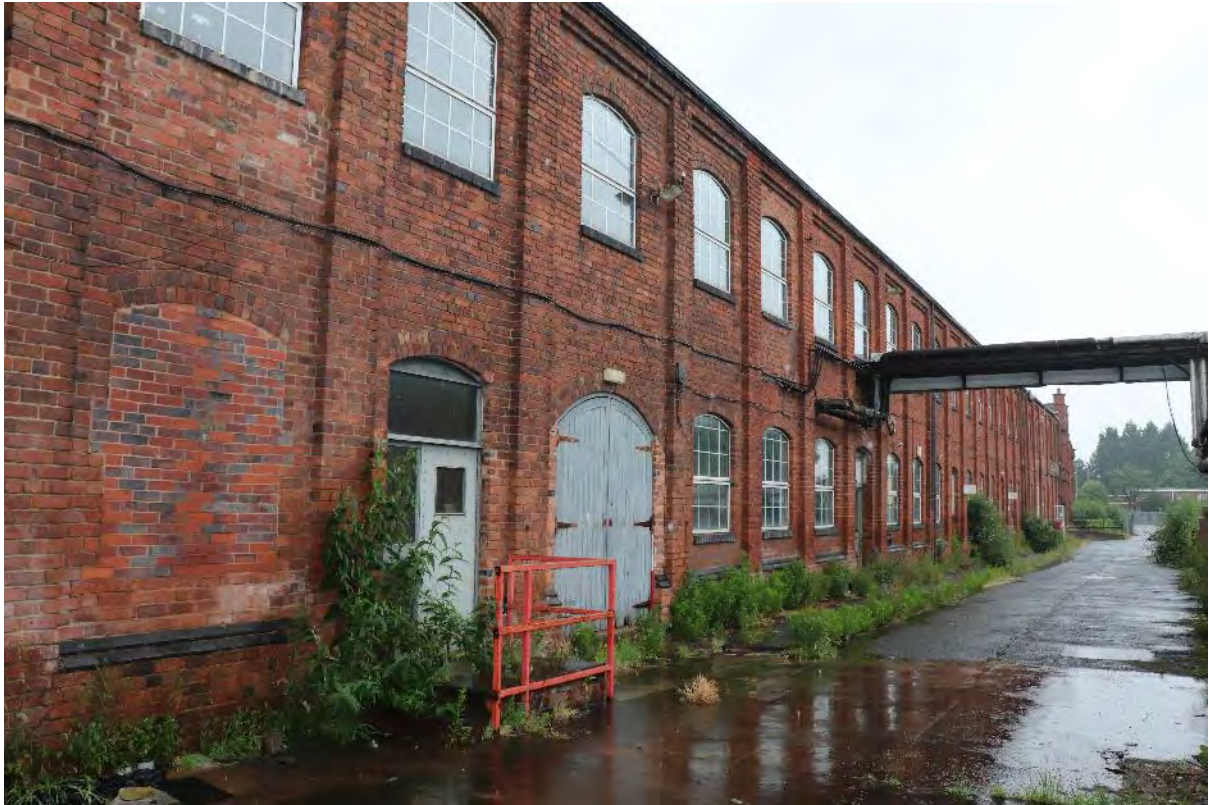
Plate 7 Duke Street north range, looking east, 1m scale
