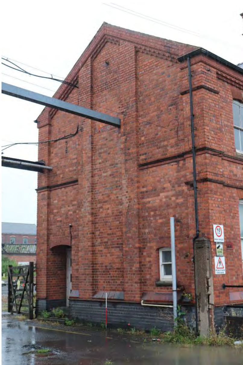
Plate 34 Phase 2 Duke Street south range north-western gable, 1m scale, looking south-east
