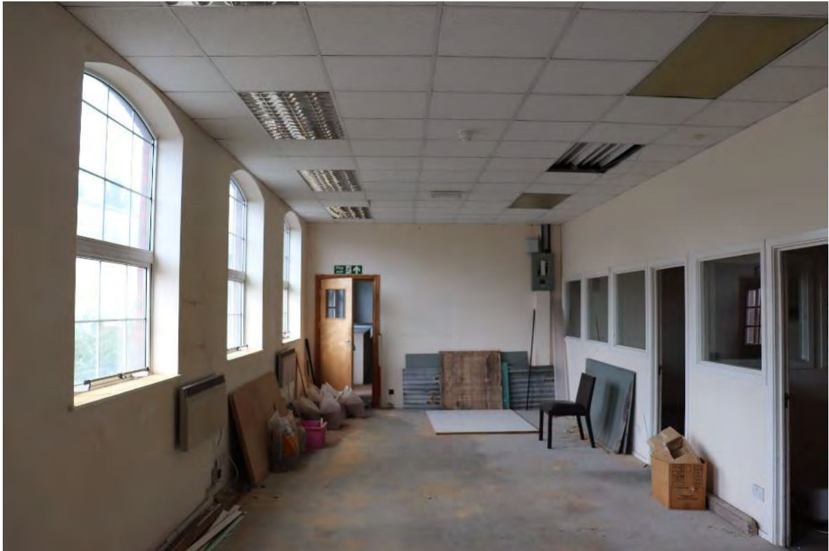
Plate 13 Phase 1a Duke Street ground floor, looking north-west, 1m scale
