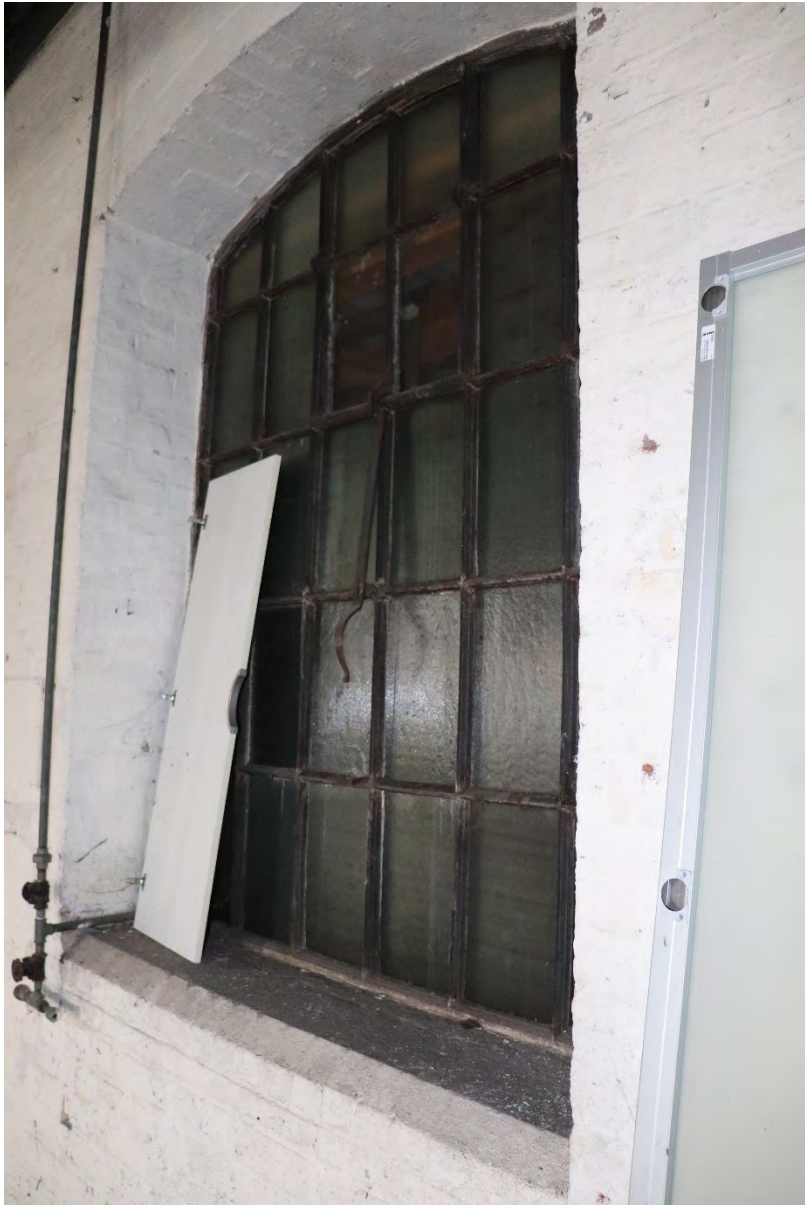
Plate 45 Phase 2 1902 building window, looking north
