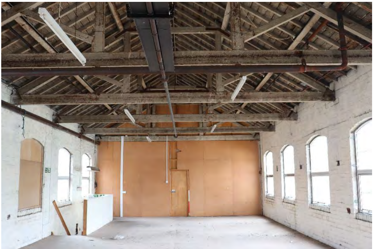
Plate 16 Phase 1a Duke Street first floor, looking south-east, 1m scale
