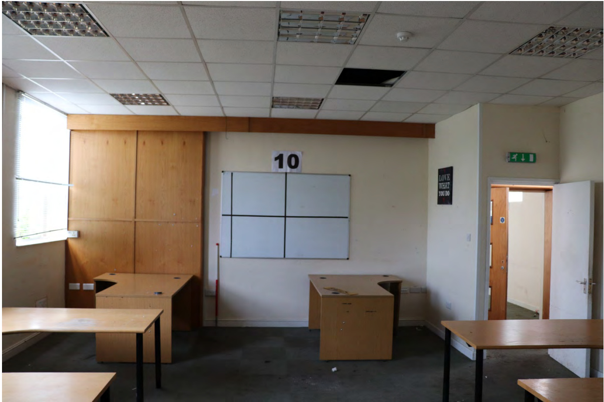
Plate 41 Phase 2 Duke Street south range ground floor, 1m scale, looking north-east
