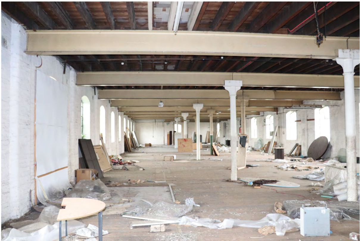
Plate 47 Phase 2 1902 building first floor, looking north-west, 1m scale
