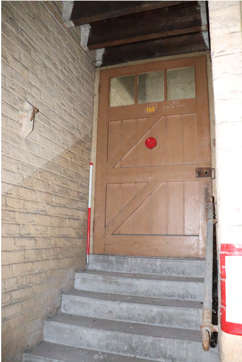
Plate 52 Phase 3 staircase added to the 1902 building, 1m scale, looking north
