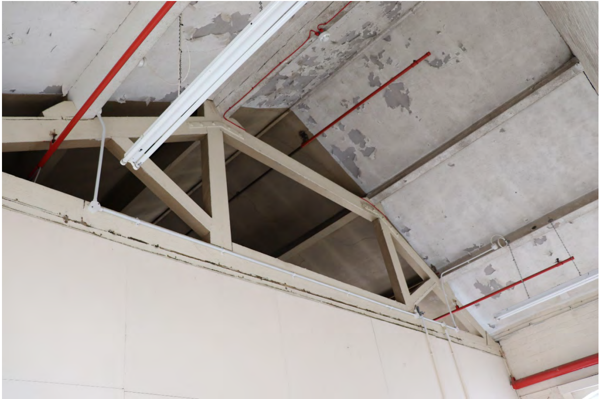
Plate 44 Phase 2 Duke Street south range roof truss, looking north
