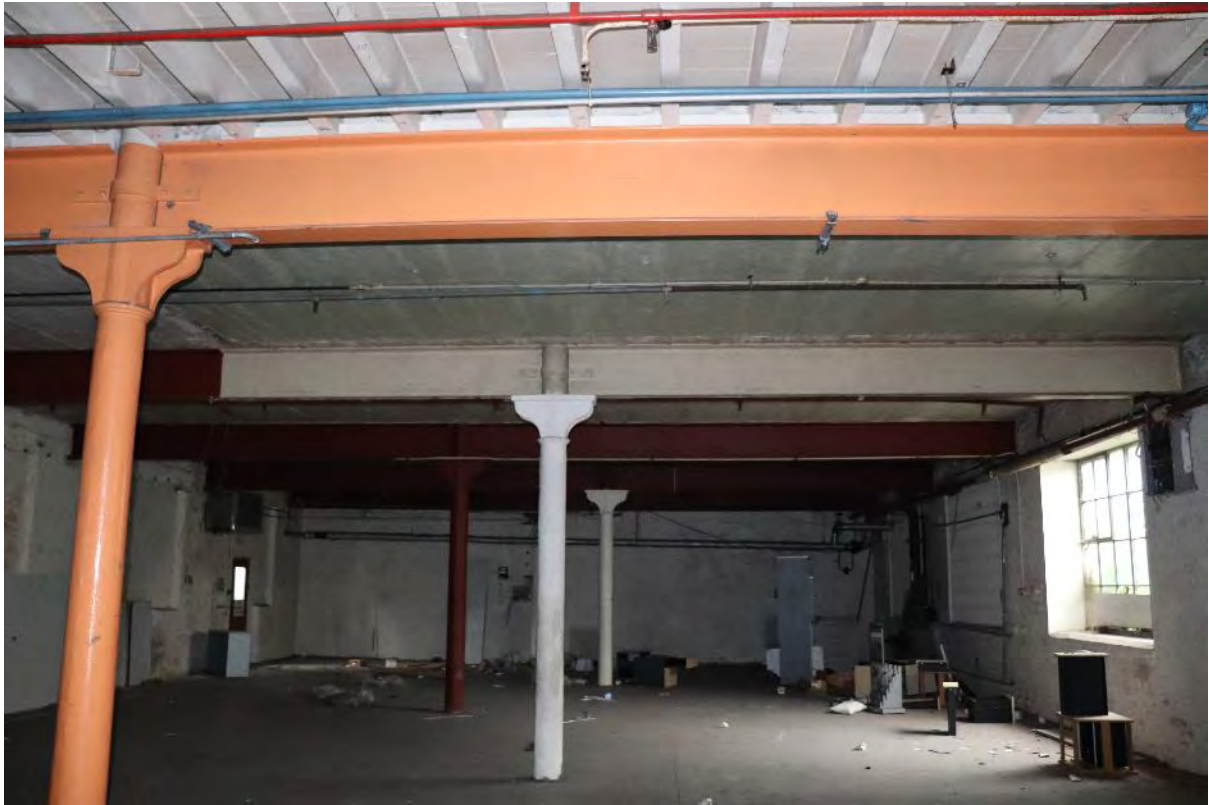
Plate 46 Phase 2 1902 building ground floor, looking north-east, 1m scale
