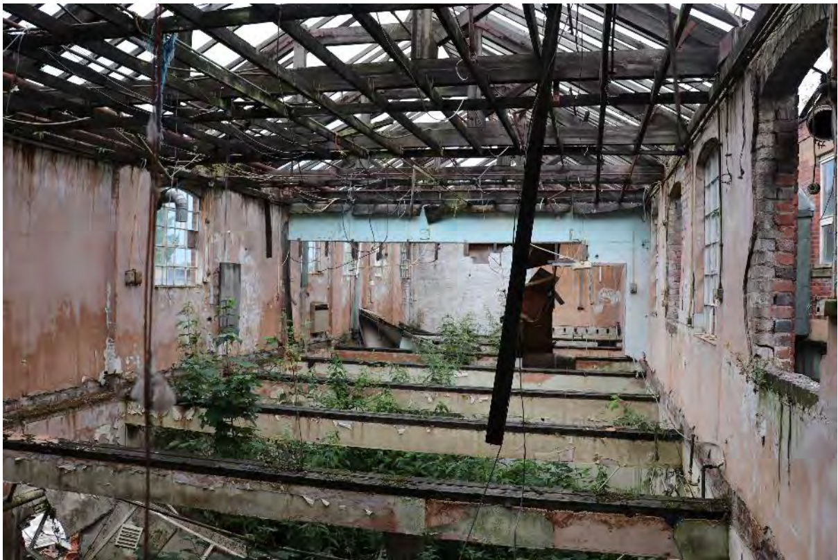
Plate 25 Phase 1 a Chenille and Yarn store first floor, looking north-east
