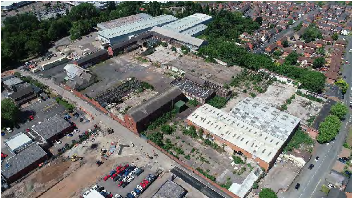
Plate 2 The site, looking west (image courtesy of RPS consulting)
