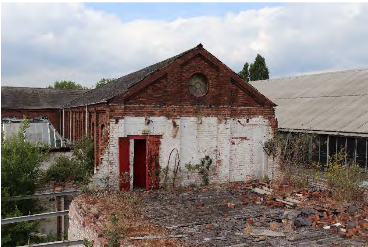
Plate 27 Duke Street north range Phase 1 b wing gable end, looking west
