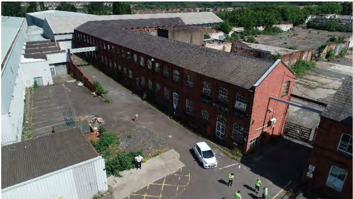
Plate 4 Duke Street north range, looking north (image courtesy of RPS Consulting)
