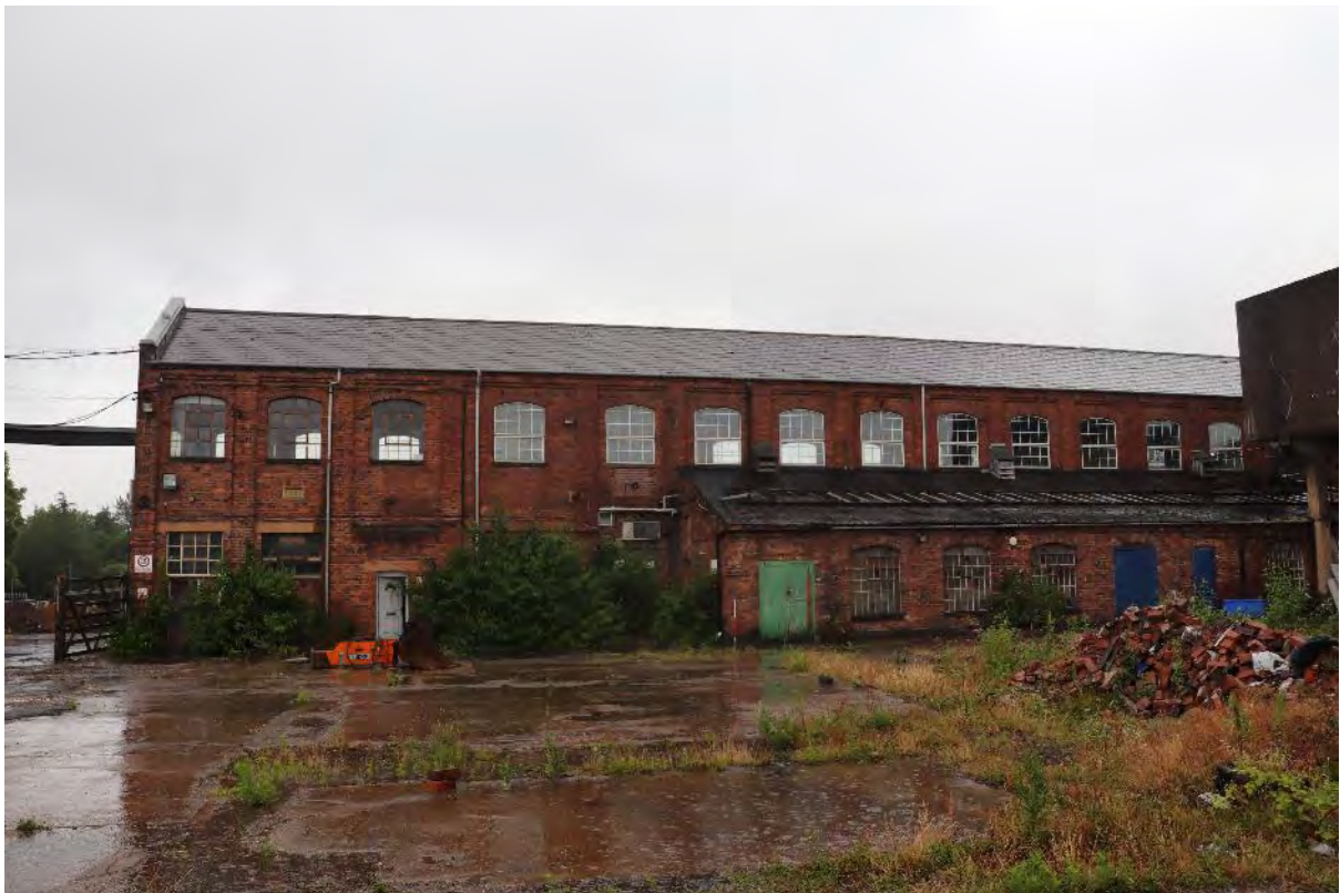
Plate 8 Duke Street north range, looking west, 1m scale
