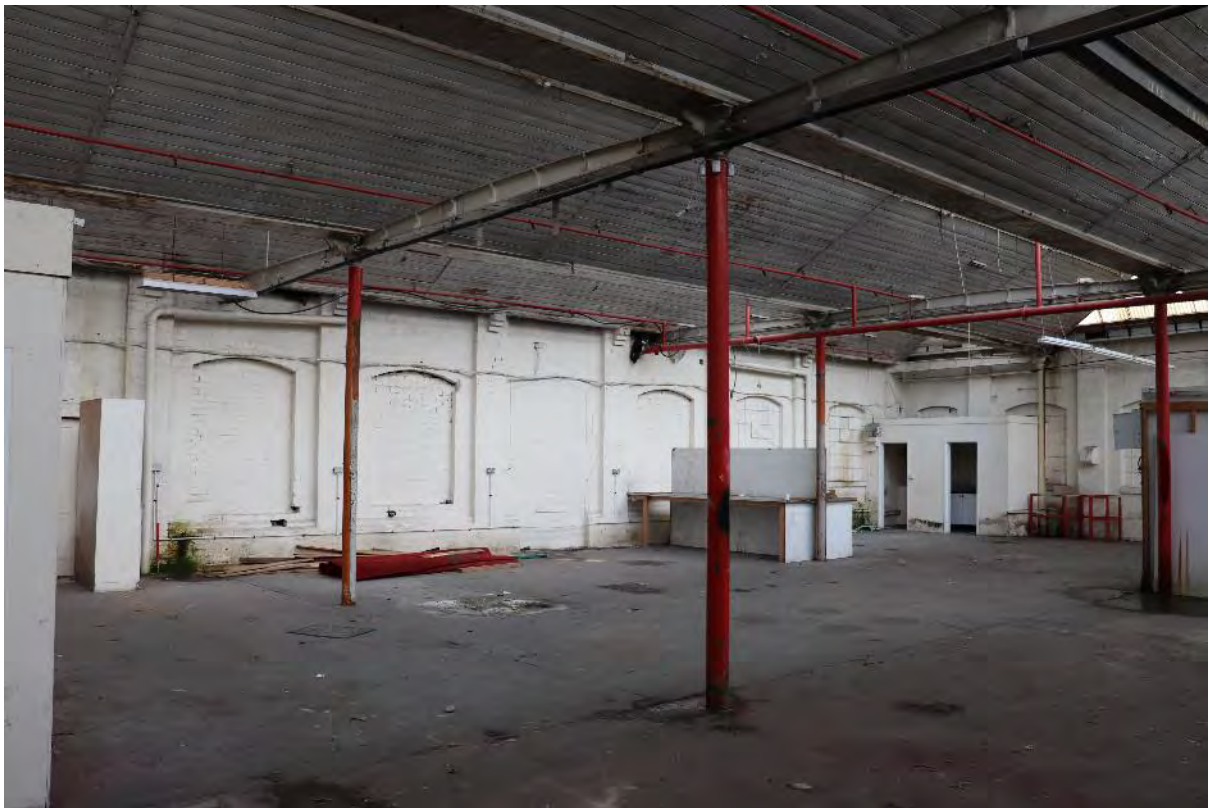
Plate 10 Duke Street north range former external wall, looking west, 1m scale
