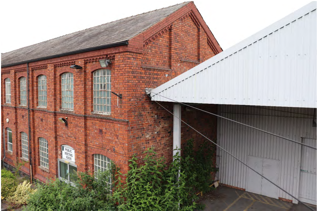
Plate 35 Phase 2 Duke Street south range south-eastern gable, 1m scale, looking north-east
