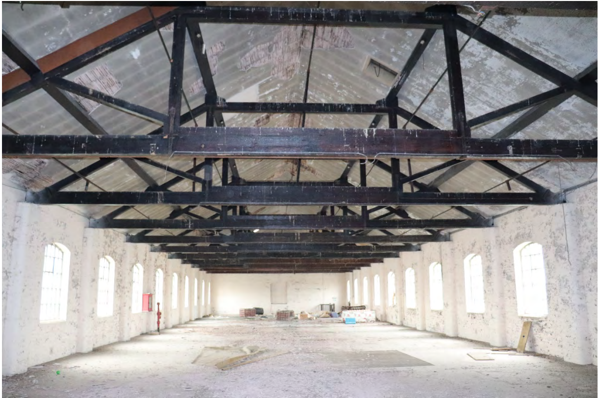
Plate 48 Phase 2 1902 building first floor, looking south-east, 1m scale
