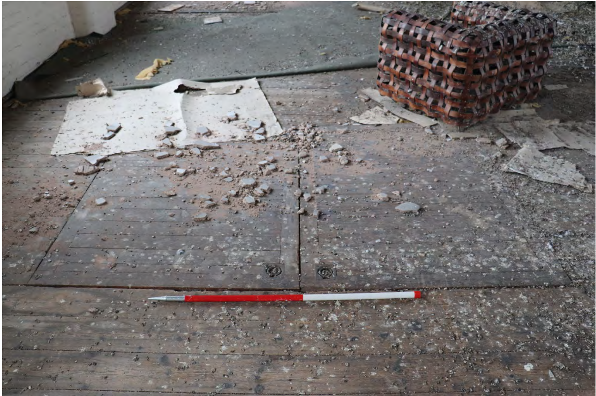
Plate 50 Phase 2 1902 building second floor trap door, looking south-west, 1m scale
