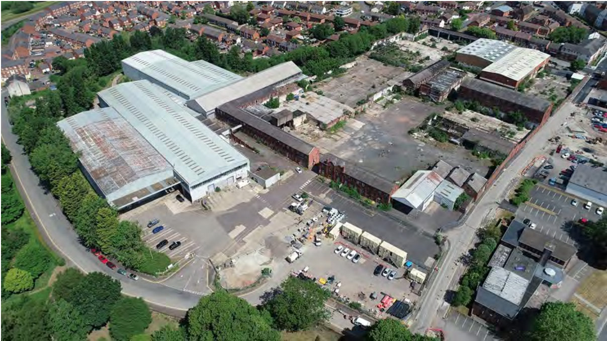
Plate 1 The site, looking north (image courtesy of RPS consulting)
