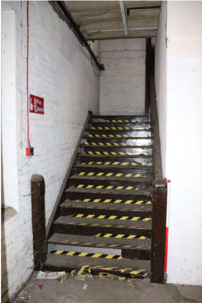
Plate 53 Phase 3 staircase added to the 1902 building, 1m scale, looking south-west
