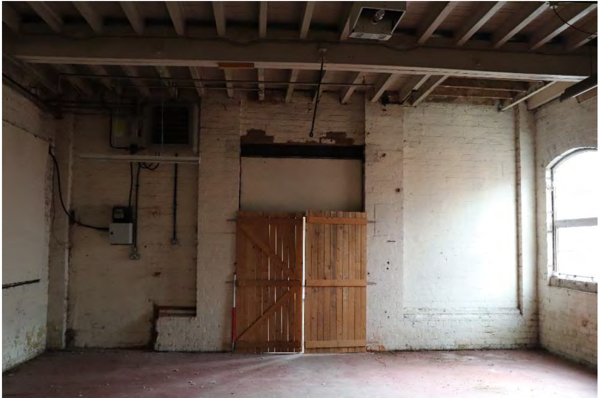
Plate 11 Phase 1a Duke Street north former gable end at ground floor level from within the Phase 1b addition, looking south-east, 1m scale
