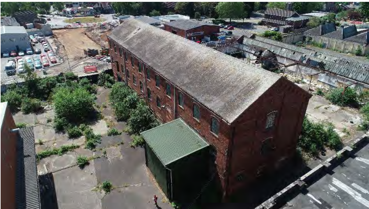
Plate 6 1902 building, looking south (image courtesy of RPS Consulting)
