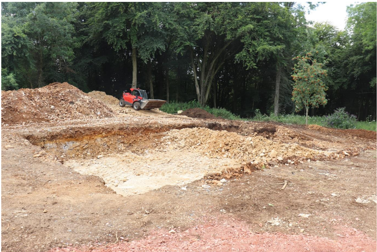
Plate 2: General shot of the trench, post excavation. Facing south
