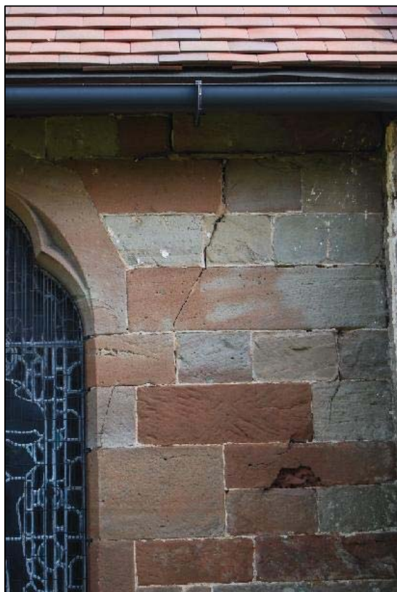
Plate 2 Cracks in the southeast wall due to subsidence
